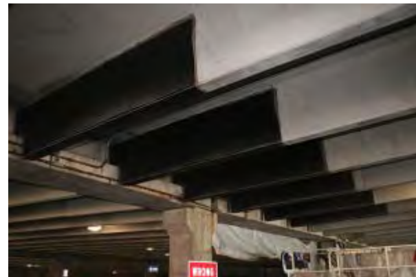
CFRP Reinforcement on Parking Garage Beams
