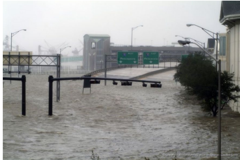
Figure 8: Flooding on I-10 Ramps
