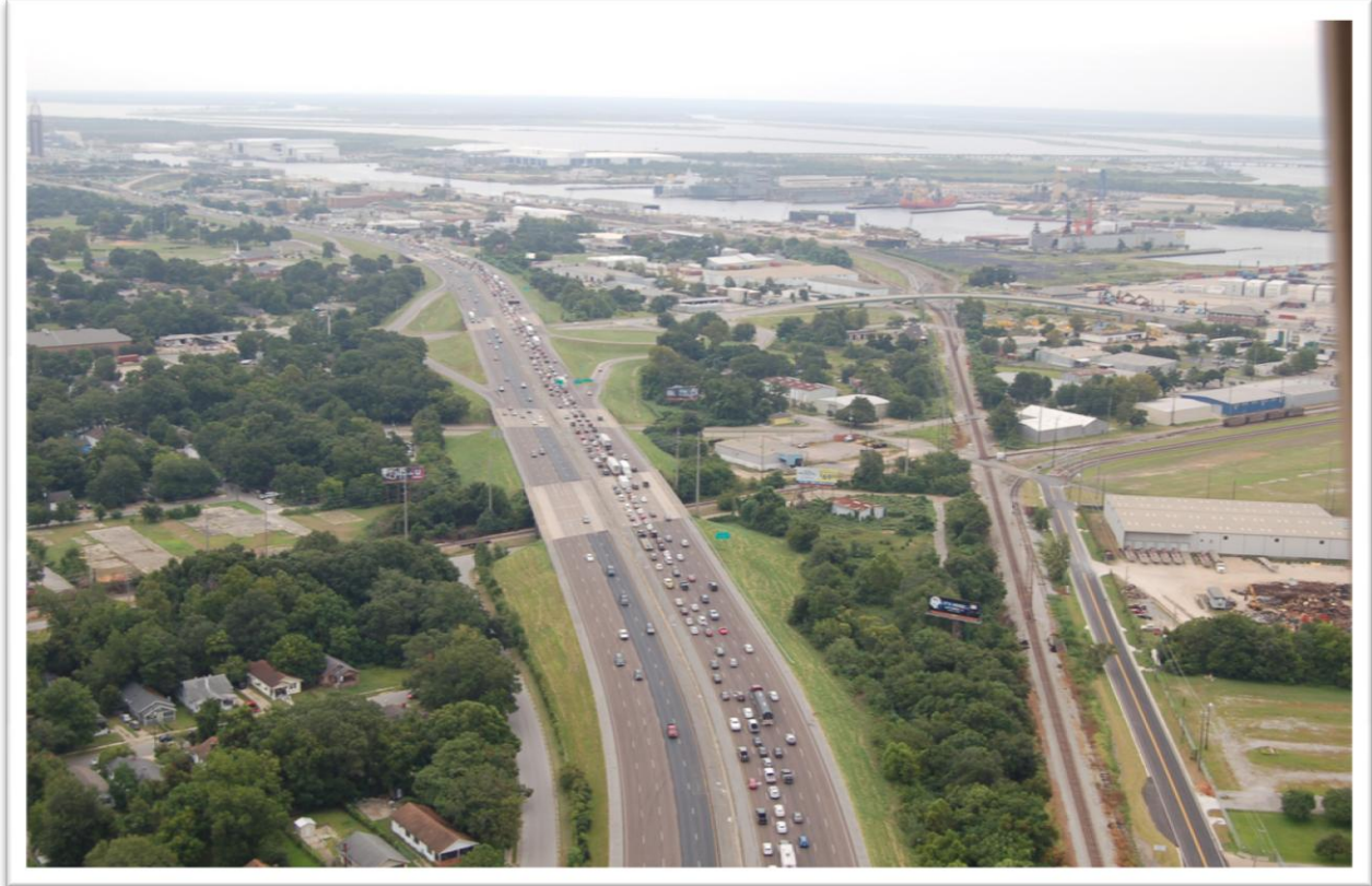
Figure 1: I-10 George C. Wallace Tunnel constraints limit both travel speeds and reliability, with the eastbound queue extending west of Virginia Street in this photograph.
