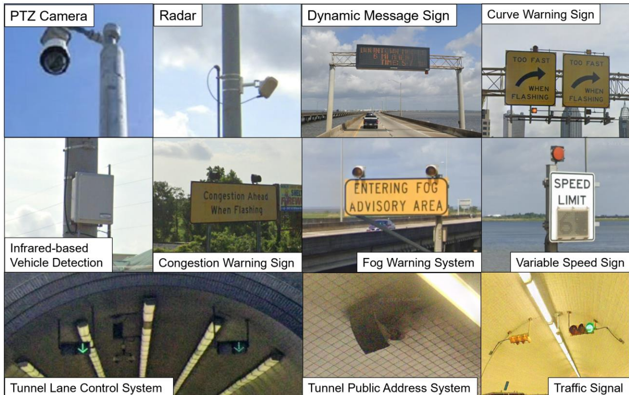
Figure 1: ITS Devices Currently in Use (source: Google Streetview)
