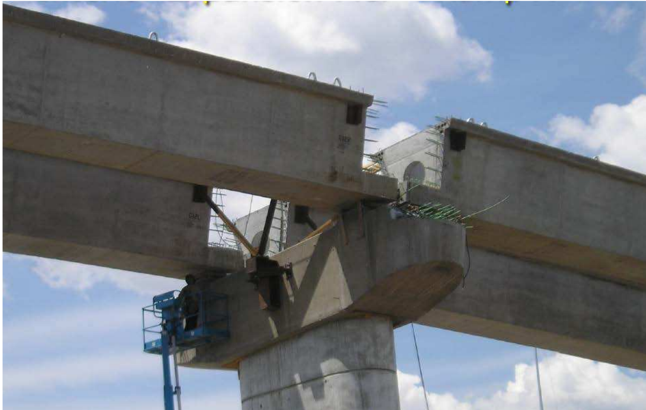
Figure 4 Placing interior diaphragm for curved U-beams at bent (photo Summit Engineering Group )
