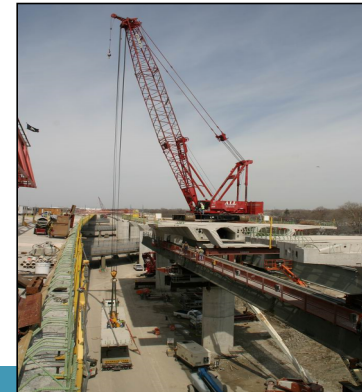
Span-by-Span Construction with Underslung Truss (Segment Delivery From Below)
