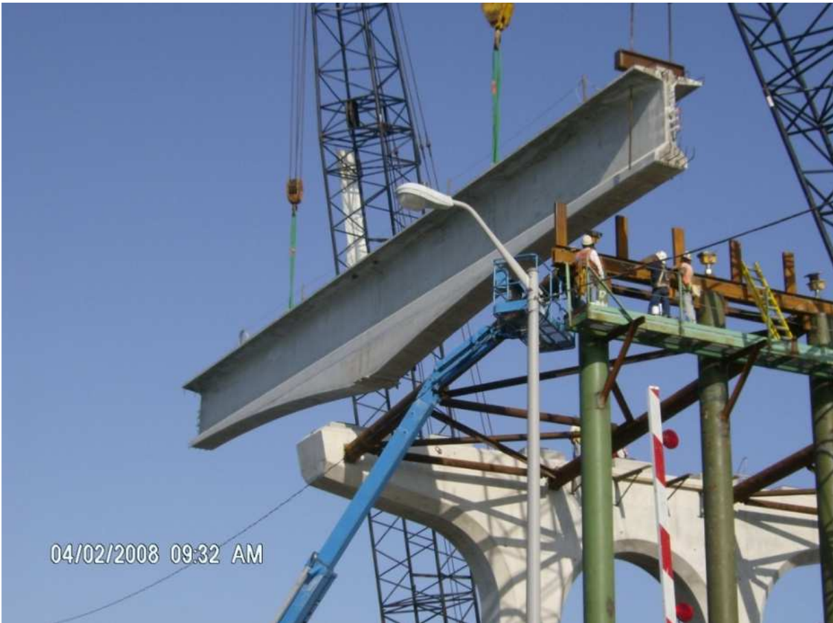
Figure 3 Haunched I-girder pier segment with shoring tower
