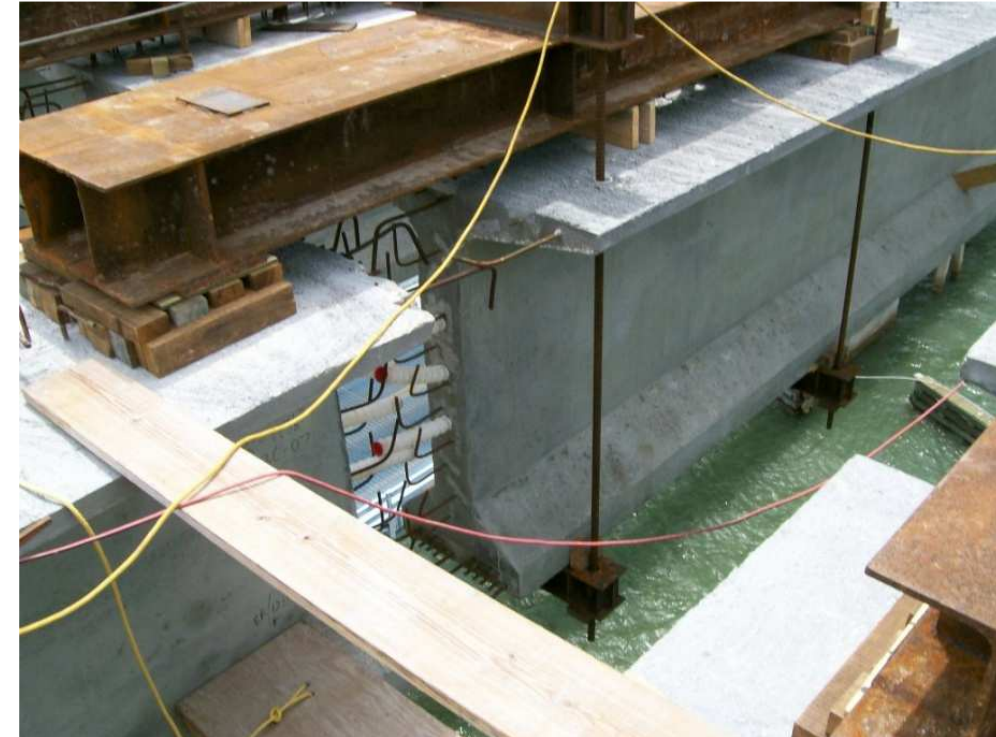
Figure 5 Splicing an I-girder using a strongback to support segments
