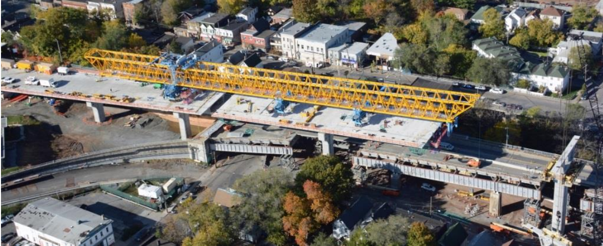
Figure 3 - Bayonne Bridge Overhead Gantry
