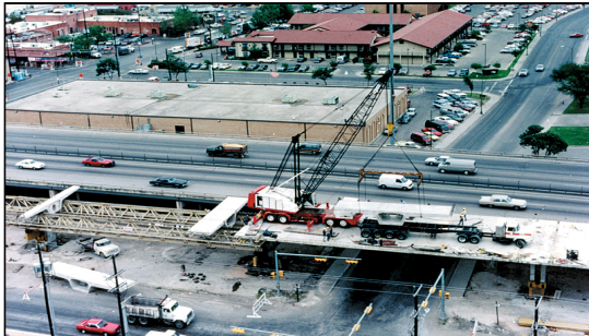
Span-by-Span Construction with Underslung Truss (Segment Delivery From Above)
