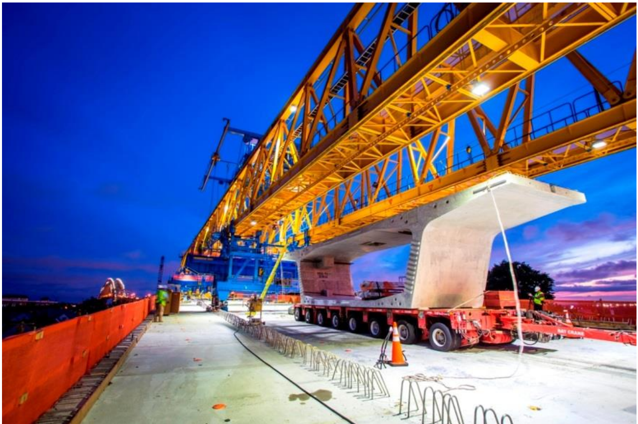
Figure 4 - Bayonne Bridge Segment Delivery
