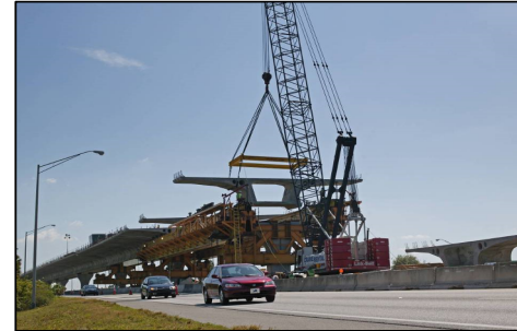
Span-by-Span Construction with Underslung Truss (Segment Delivery From Below)
