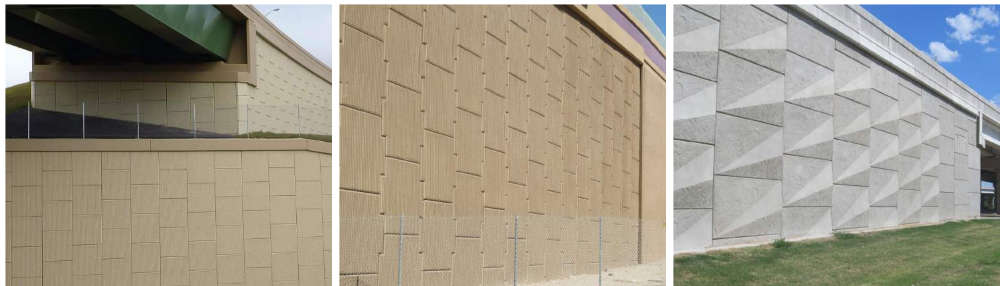
Top : Abutment wall configurations- Vertical, full slope, partial slope | Bottom: Sample colors and finish for retaining wall
