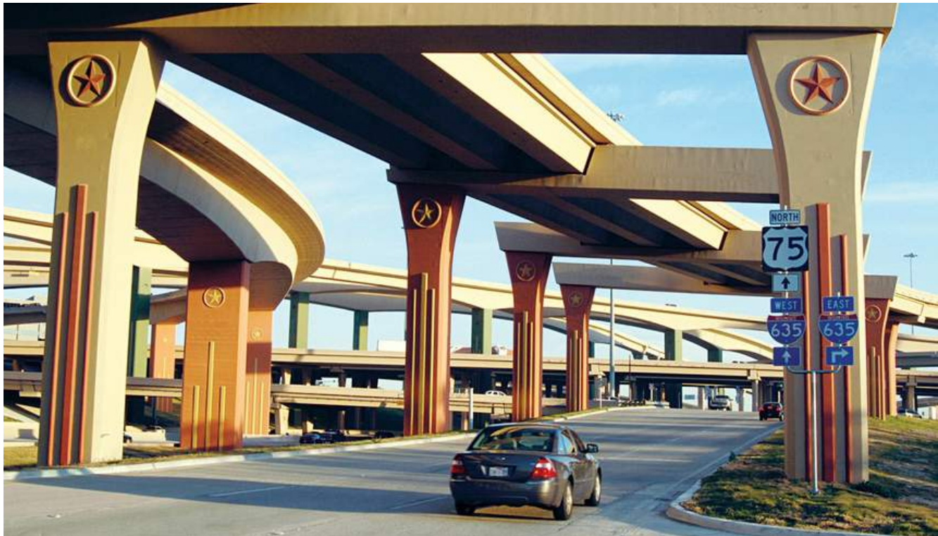
All: Straddle bents with closed box superstructure in various relationships to the at grade roadway
