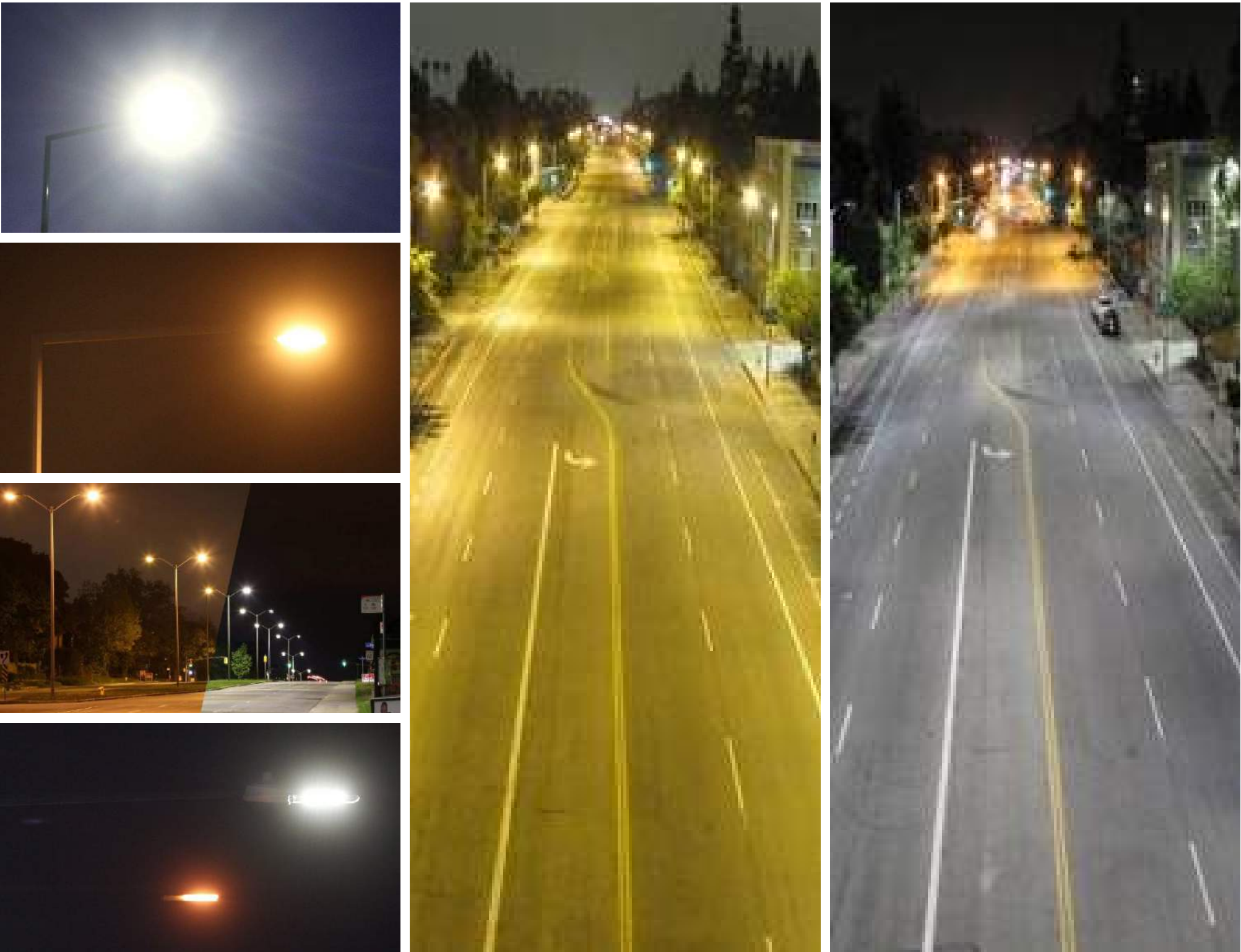
Left: Samples of High Pressure Sodium and LED/Metal Halide | Middle: Example for High Pressure Sodium | Right: Example of LED and High Pressure Sodium
