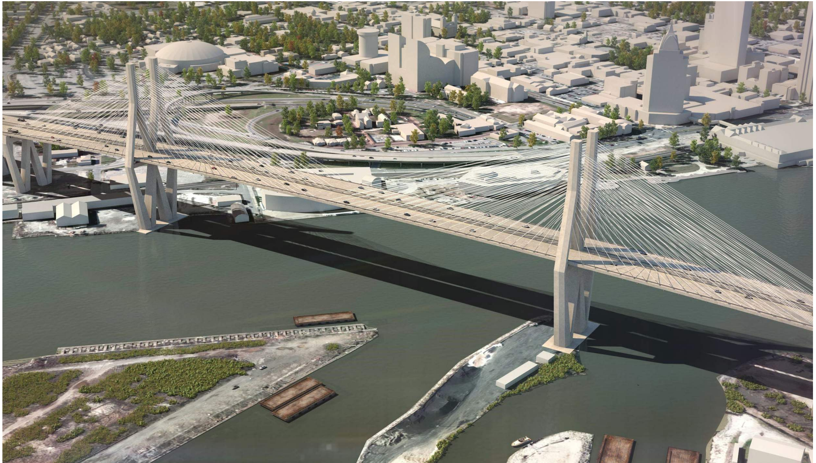
Aerial Rendering of the Main-span and Tie-down Pier with faceted form
