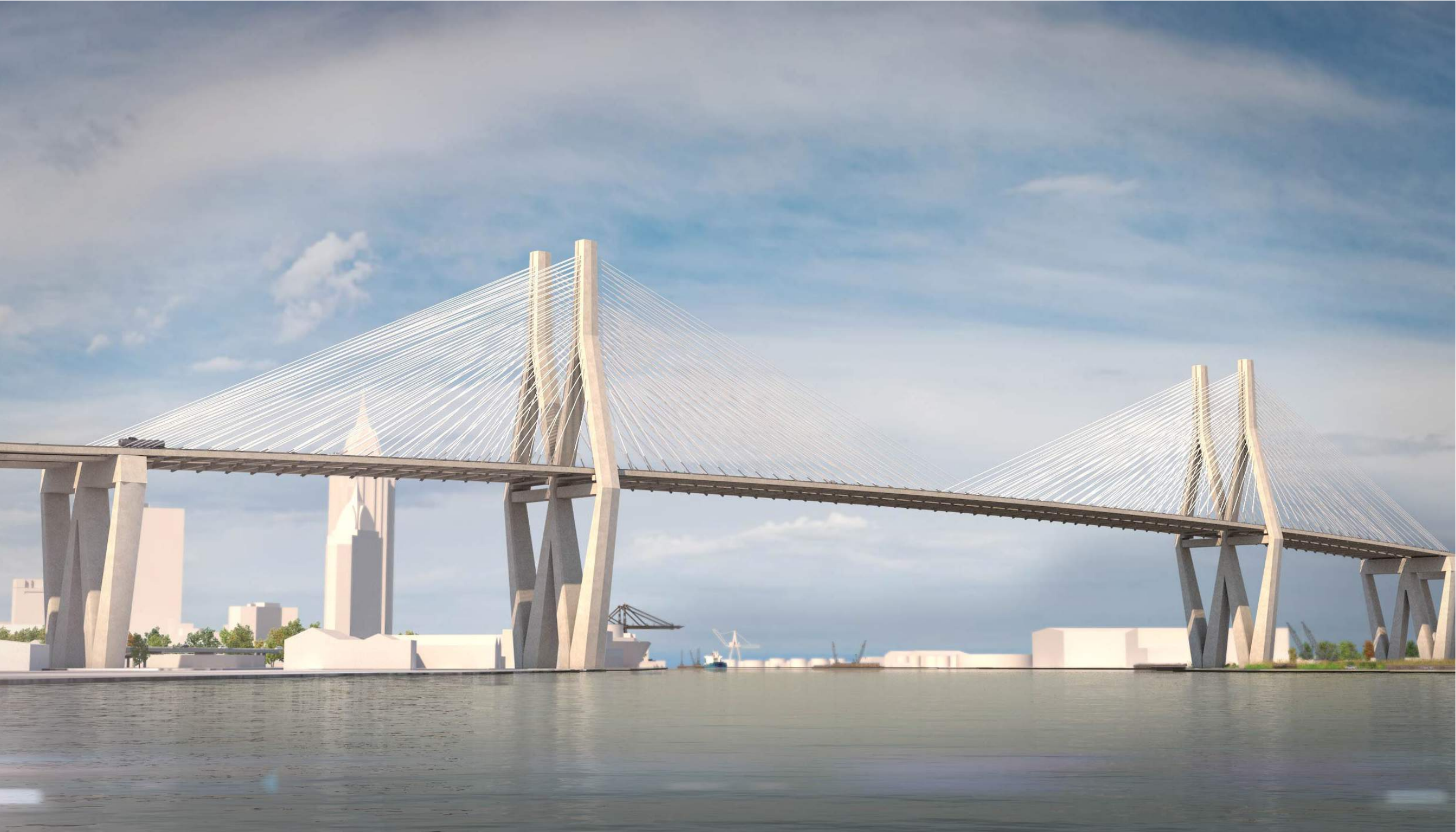
Water level rendering of the Main-span and Tie-down Piers with Faceted form
