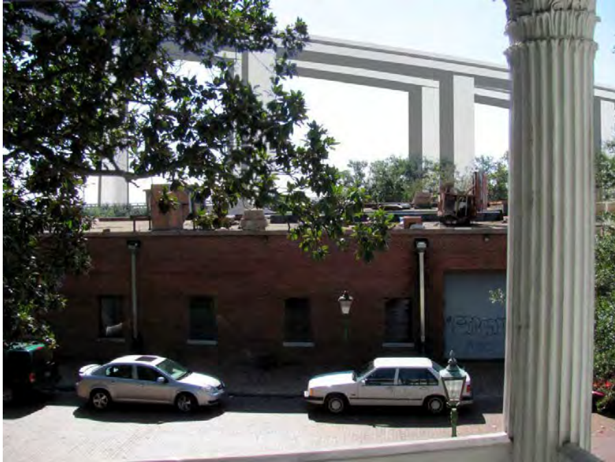
View to the south from the second-story front balcony of Condé-Charlotte Museum House showing Alternative A.
