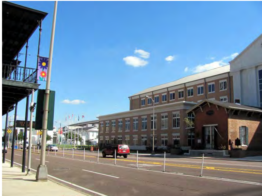
View from the intersection of Government and Conception Streets to the southeast viewshed showing Alternative B' and a mixture of historic and non-historic structures. Alternative B would be similarly visible. Alternative C would not be visible.
