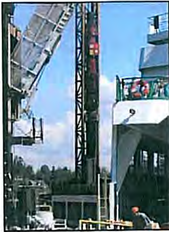
D30-42 Finishing Dolphin Piles.
