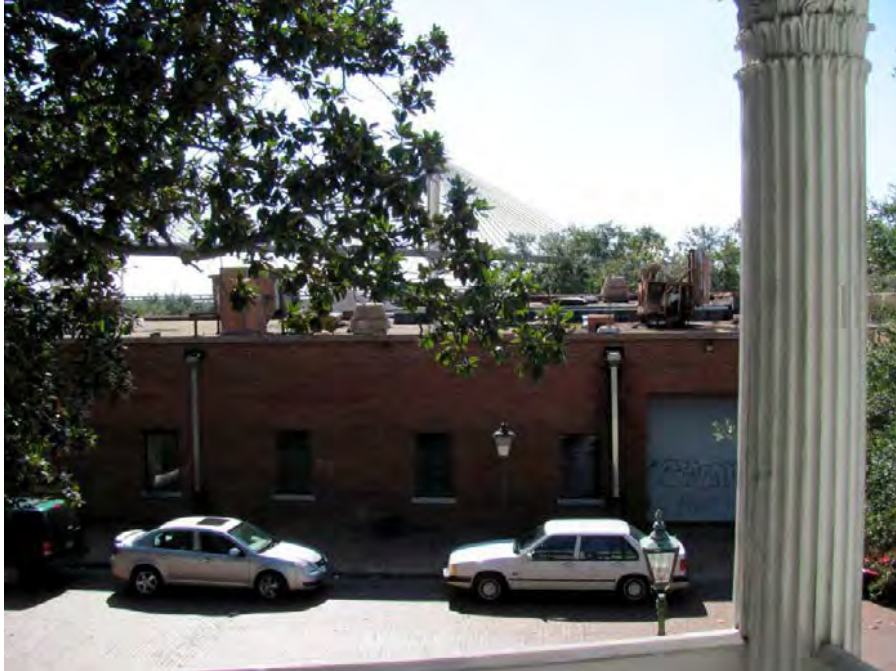
View to the south from the second-story front balcony of Condé-Charlotte Museum House showing Alternative C.
