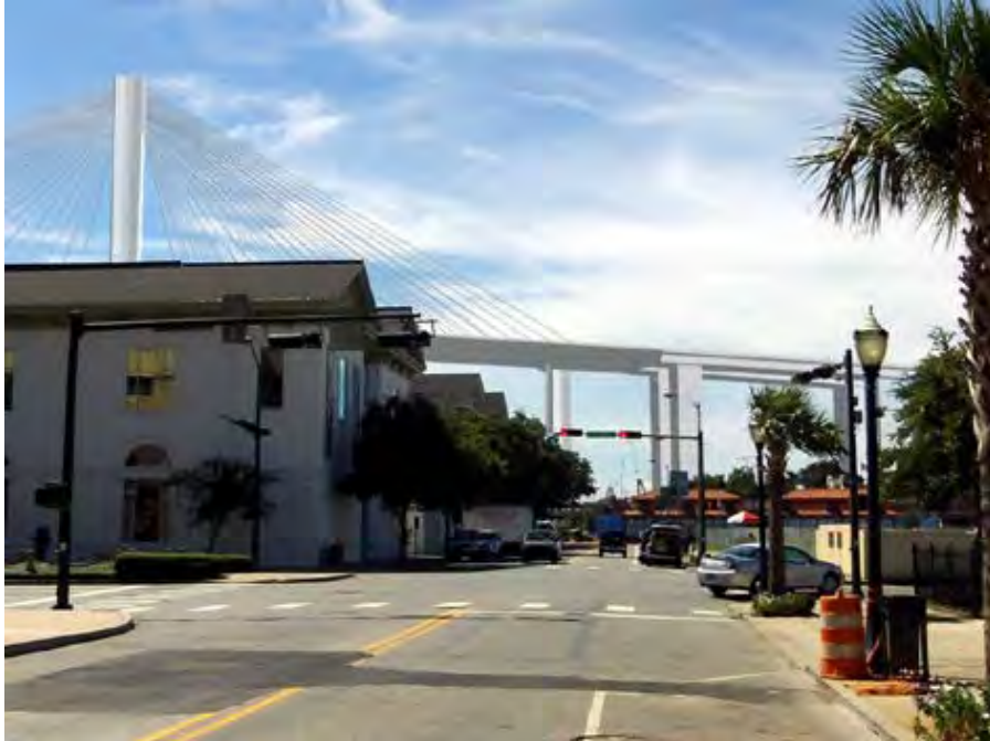
View to south from S. Royal Street showing Old Southern Market and City Hall and Alternative A.
