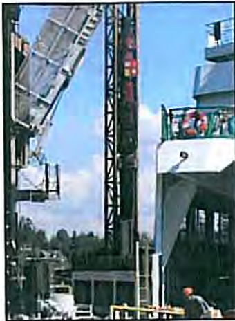
D30-42 Finishing Dolphin Piles.
