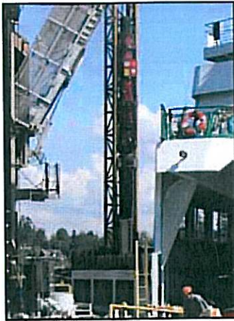
D30-42 Finishing Dolphin Piles.
