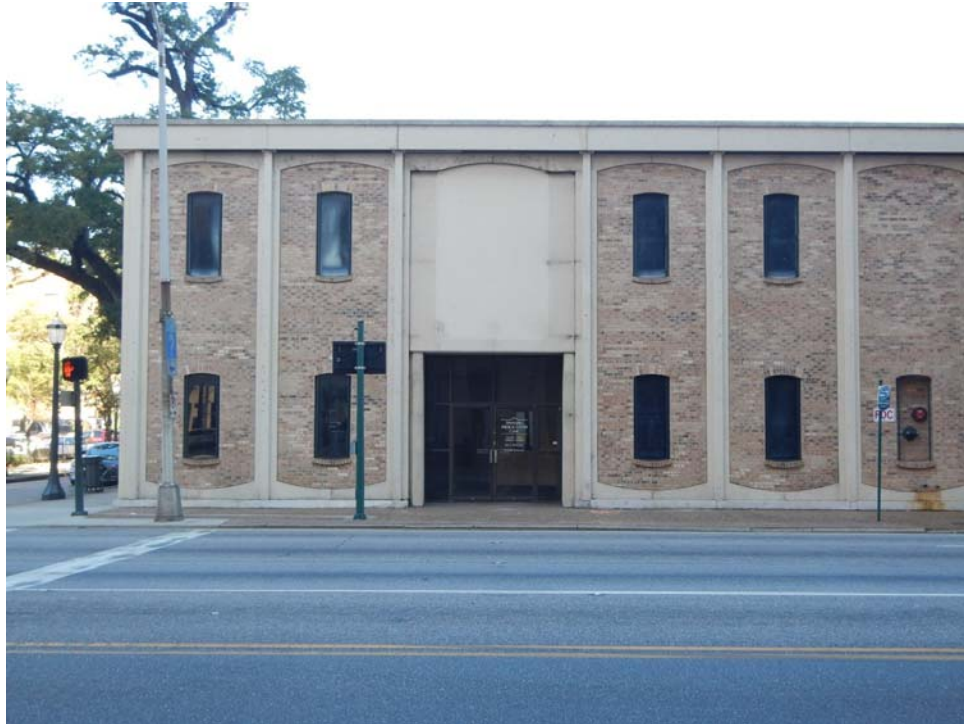
Figure 38. Building at 210 Government Street, view to the north-northwest.
