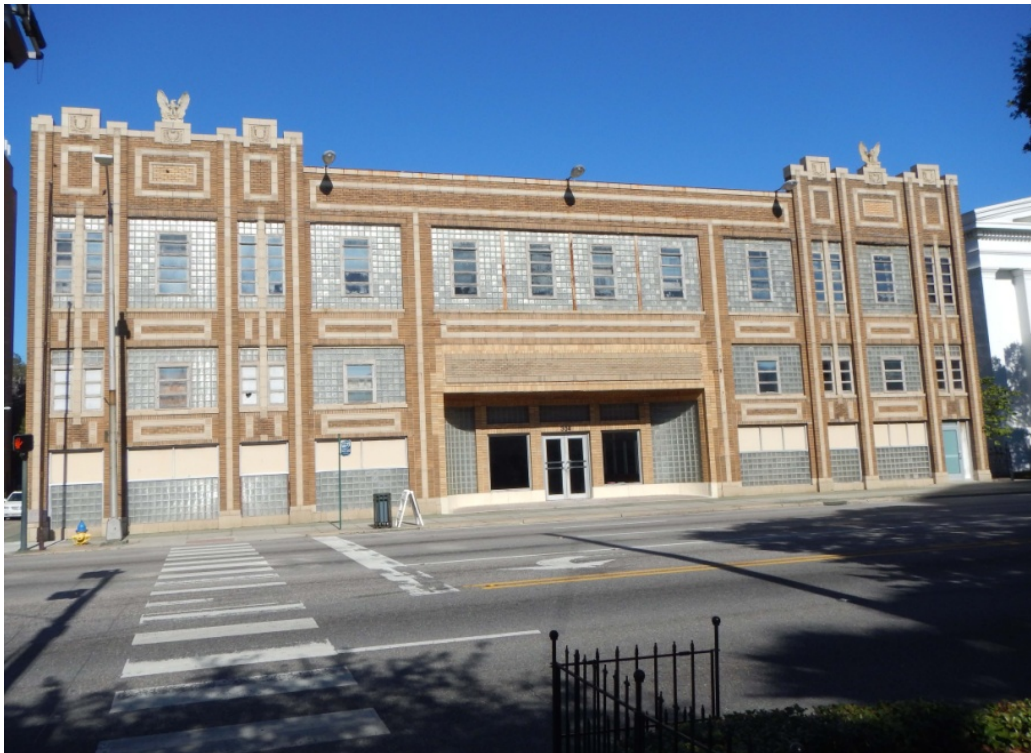
Figure 45. Façade of the Mobile Press-Register Building at 304 Government Street, view to the north.
