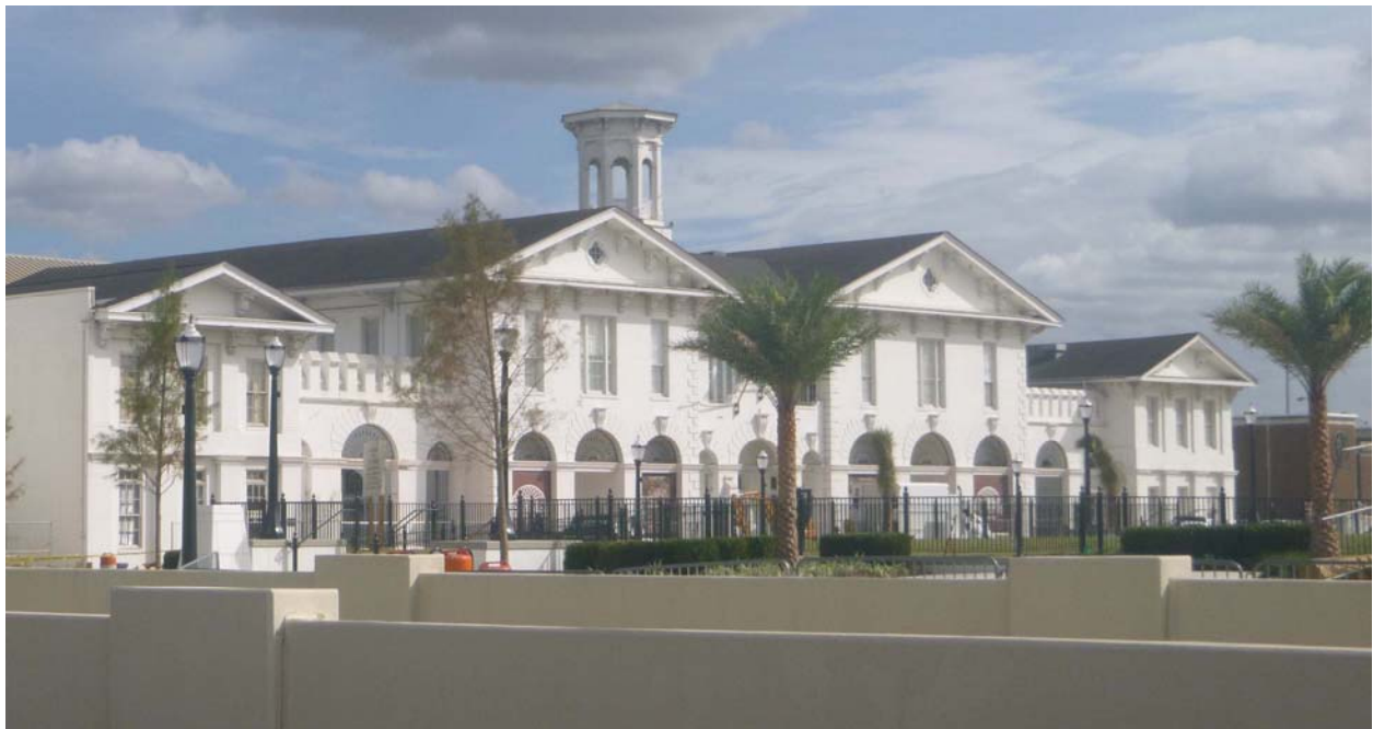
Figure 64. West side of Southern Market (now History Museum of Mobile), view to the southeast with the concrete entrance to Bankhead Tunnel in the foreground.
