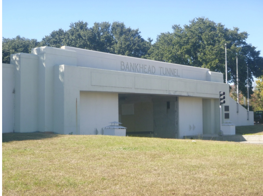
Figure 14. East entrance of Bankhead Tunnel on the east side of the Mobile River, view to the northwest.
