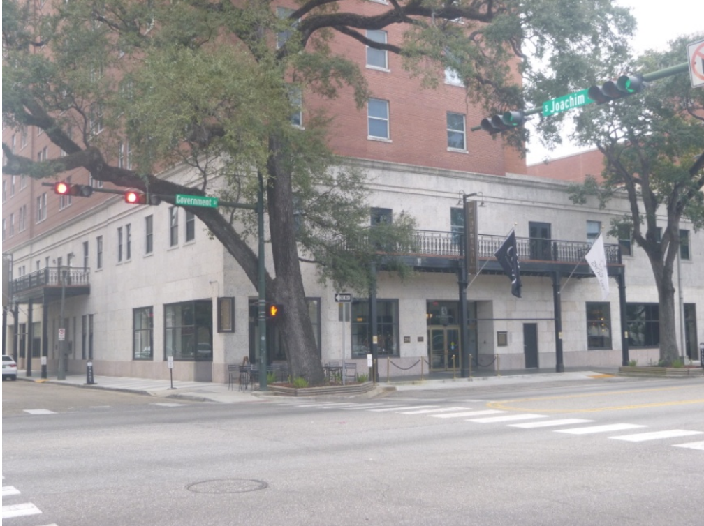
Figure 57. East entrance on S. Joachim Street (left) and north entrance on Government Street (right) to Admiral Semmes Hotel, view to the southwest.
