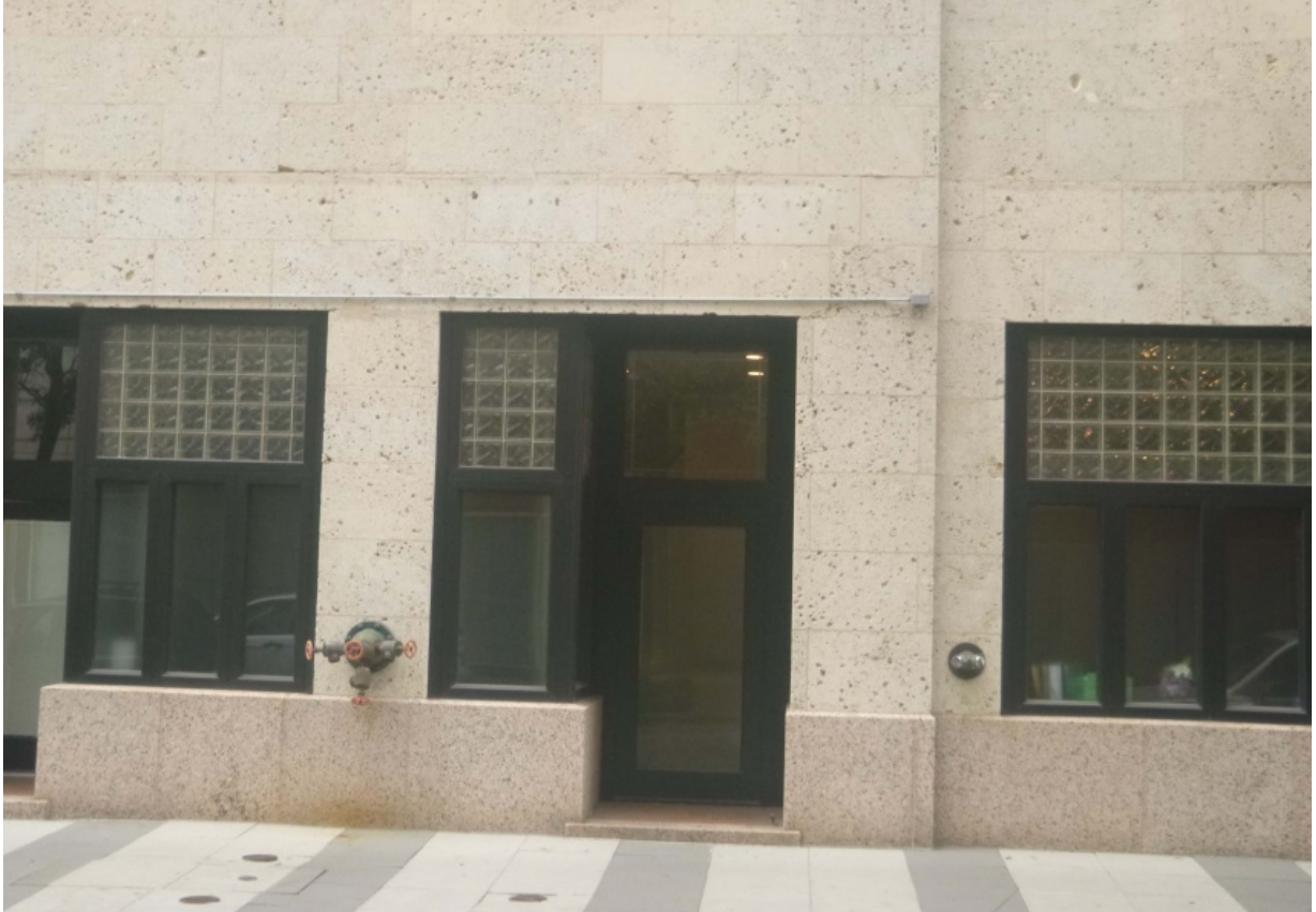
Figure 59. Detail of the pinkish granite (lower) and locally-mined limestone with numerous fossils (upper) on the first floor of Admiral Semmes Hotel.
