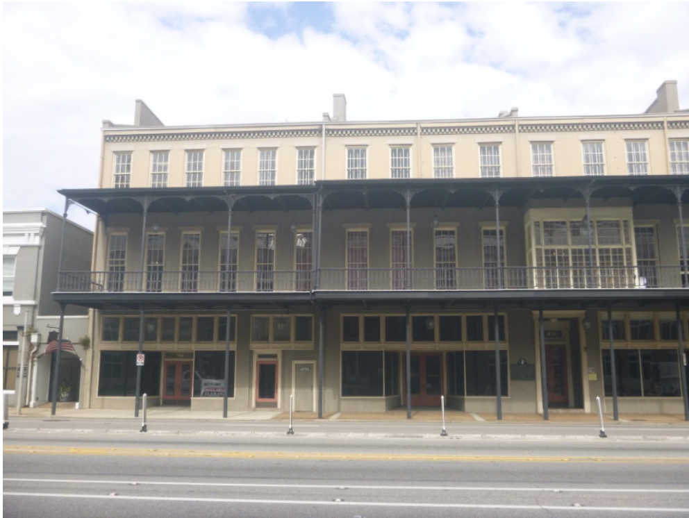
Figure 26. Original Federal-style brick buildings constructed in 1856 at 156 and 158 Government Street (right) and 1940 addition (left) built to look like the older buildings, view to the north-northwest.
