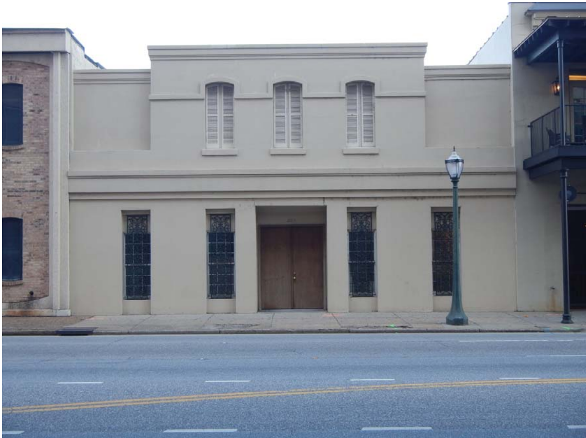
Figure 36. Façade of early 20th-century building at 206 Government Street, view to the north-northwest.
