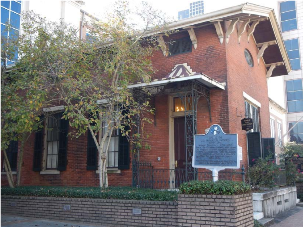
Figure 51. East side of Dr. Levert's Office, view to the southwest.
