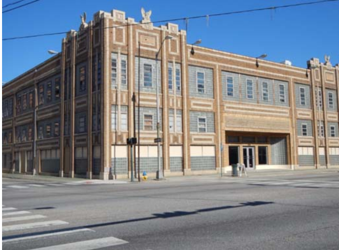
Figure 46. Mobile Press-Register Building at 304 Government Street, view to the northeast.
