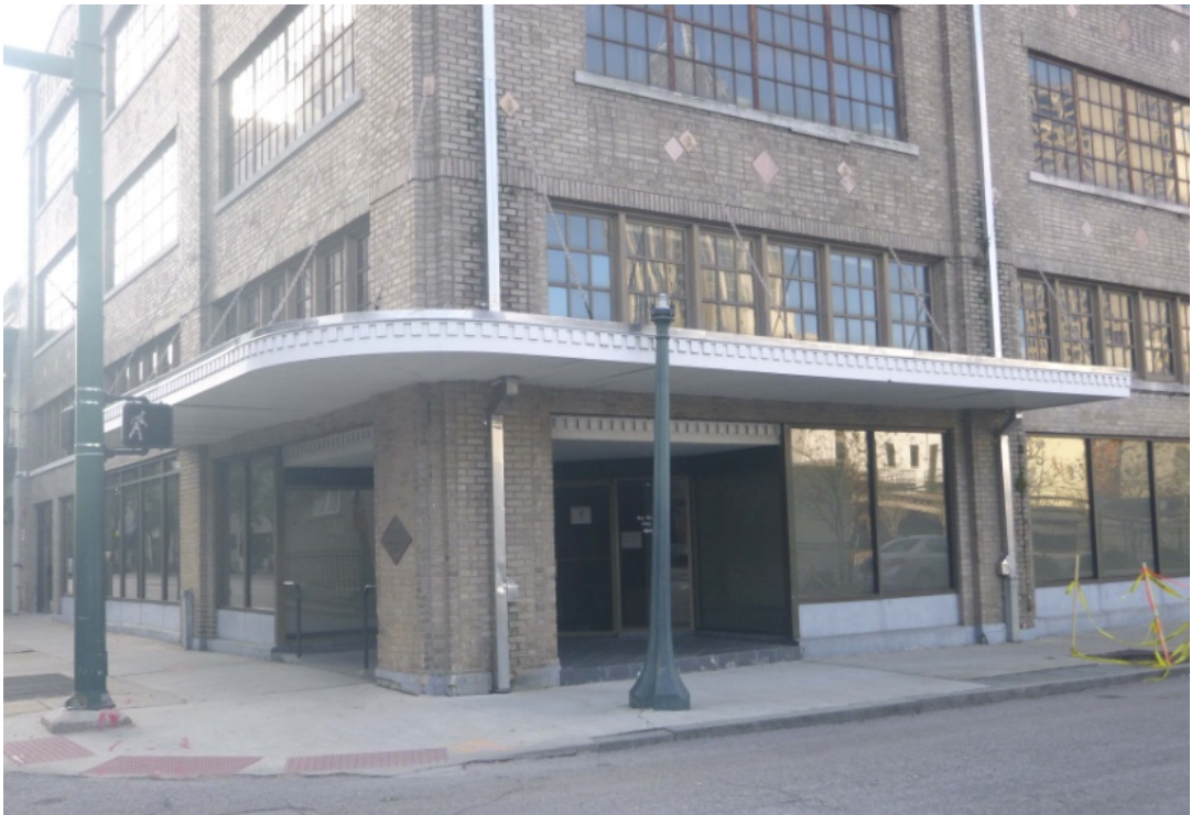
Figure 34. Corner entrance to the building at 200 Government Street.
