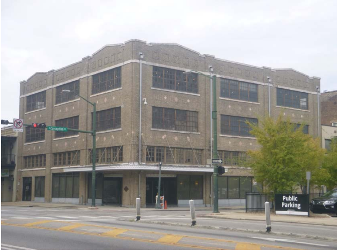
Figure 33. Building at 200 Government Street, view to the northwest.
