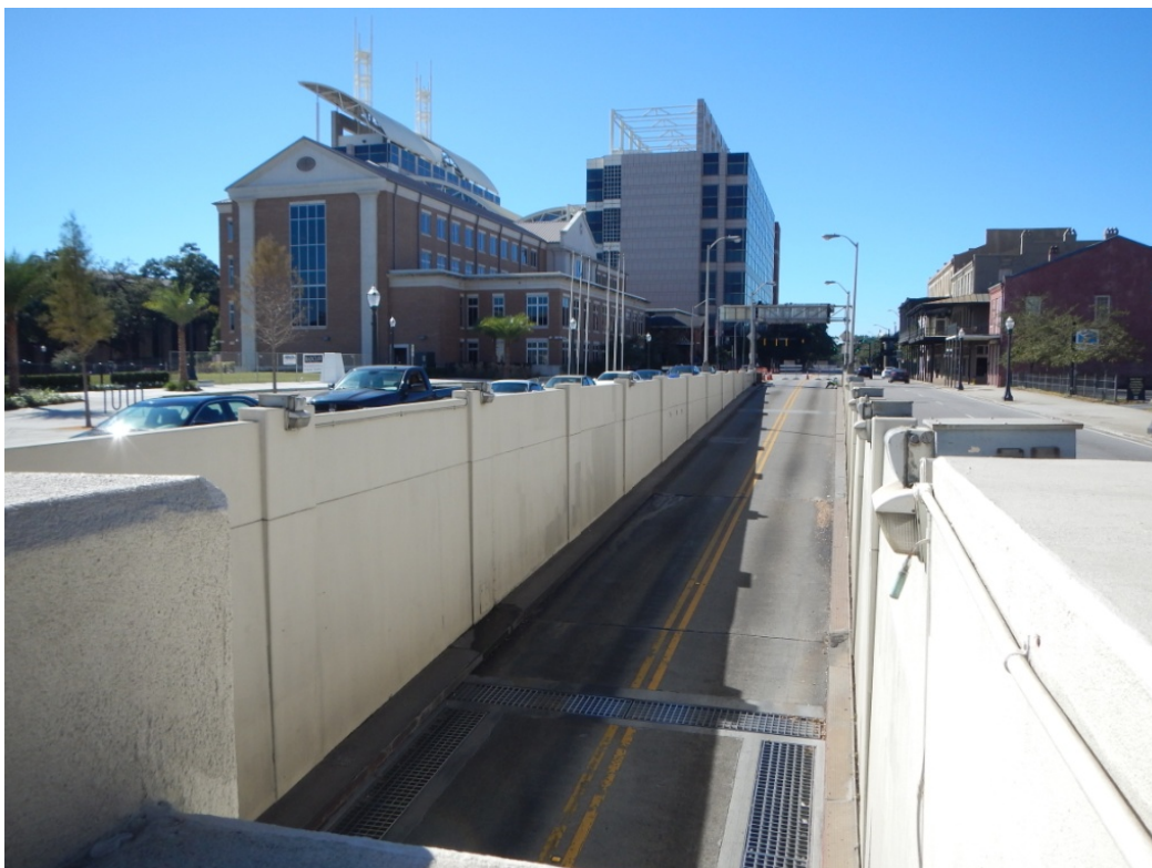
Figure 11. West entrance to Bankhead Tunnel in the middle of Government Street, view to the west-southwest.
