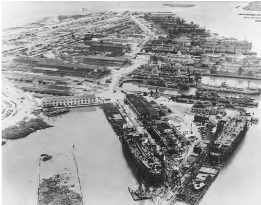
Alabama Dry Dock & Shipbuilding Company (ADDSCO) shipyard on Pinto Island, ca. 1950 (ADDSCO Collection, University of South Alabama Archives)
