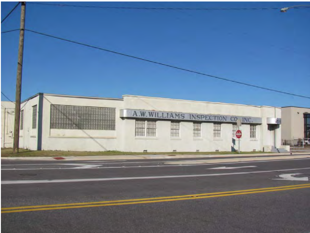
Figure 31. View to the northwest of Structure 19a, office building for A.W. Williams Inspection Co., Inc. at 208 Virginia Street on Survey Block 32.
