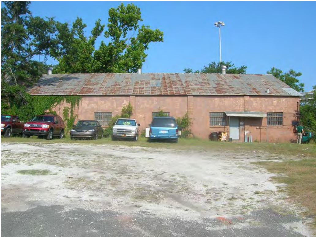
Figure 51. Structure 12, originally Montgomery Elevator Company, former File Storage and Electrical Shop, for the former Bender Shipyard. View to the west toward Alternate A. Alternates B and B’ would cross over the south end of Structure 12.
