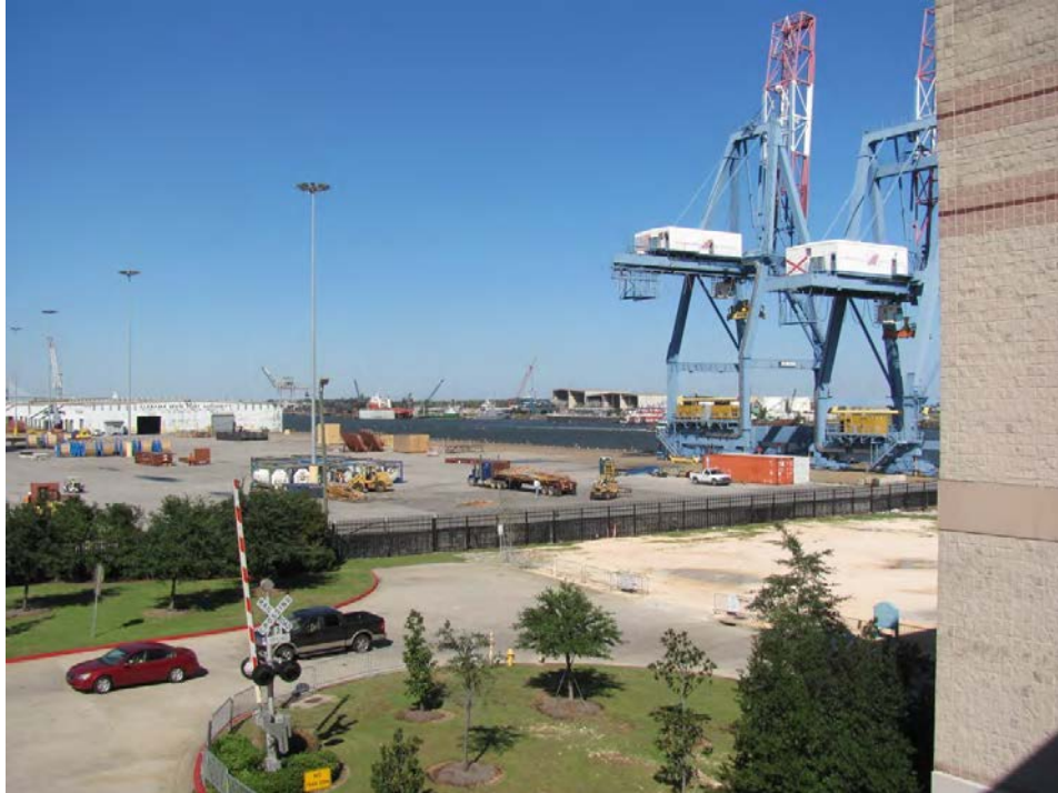
Figure 52-2. View to the north-northeast of Alabama State Docks and Mobile River from the second-story balcony on the north side of the Arthur R. Outlaw Mobile Convention Center (Resource #52).
