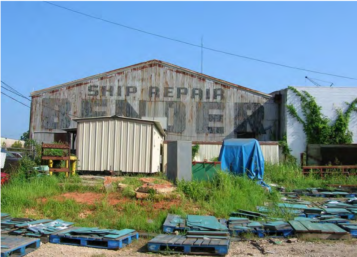
Figure 29. North side of Structure 4, machine shop, for former Bender Shipyard. View to the north toward Alternates A, B, and B'.
