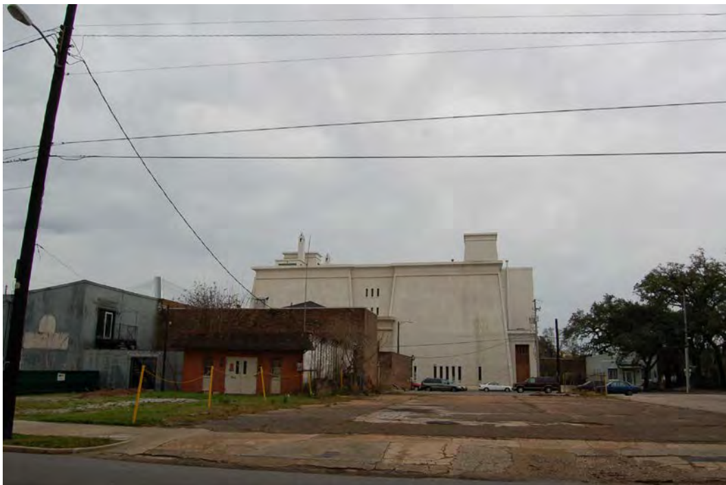
Figure 33-7. View to the south-southeast from the AT&T Building (Resource #33) showing Alternate B (left) with a sparse tree canopy, the rears of historic brick commercial buildings, the Scottish Rites Temple (Resource #36) (center), a vacant lot, and a paved parking lot across St. Michael Street. Due to distance (0.6 miles) and blockage by structures, Alternate B would be partially visible (10-20%) from this location. Alternate B' would be similarly visible.
