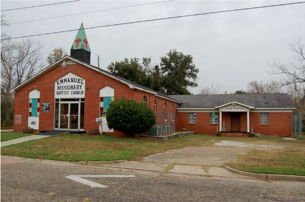
Figure 15-1. View to the north of Emmanuel Missionary Baptist Church (Resource #15) at 1108 Chimquapin Street in the MLK Heritage Neighborhood.
