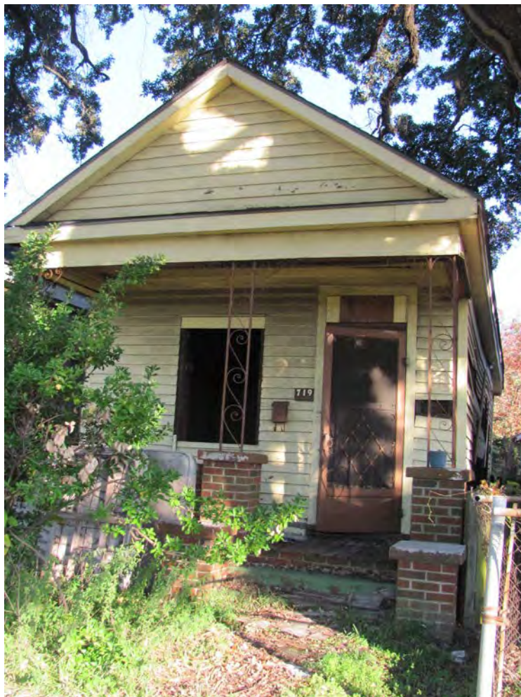
Figure 7. View to the east of Structure 4, shotgun house at 719 S. Conception Street on Survey Block 1.
