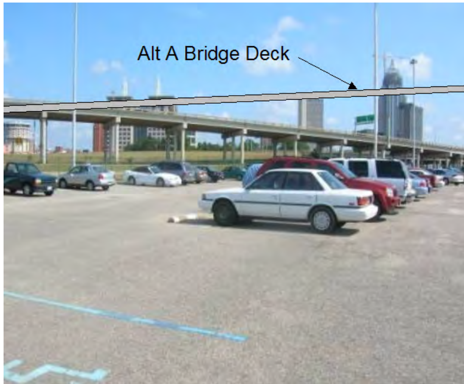
Figure 4. View to the northwest of the proposed location of Alternate A bridge deck north of the parking lot for the main offices of the former Bender Shipbuilding & Repair Company, Inc., showing existing I-10.
