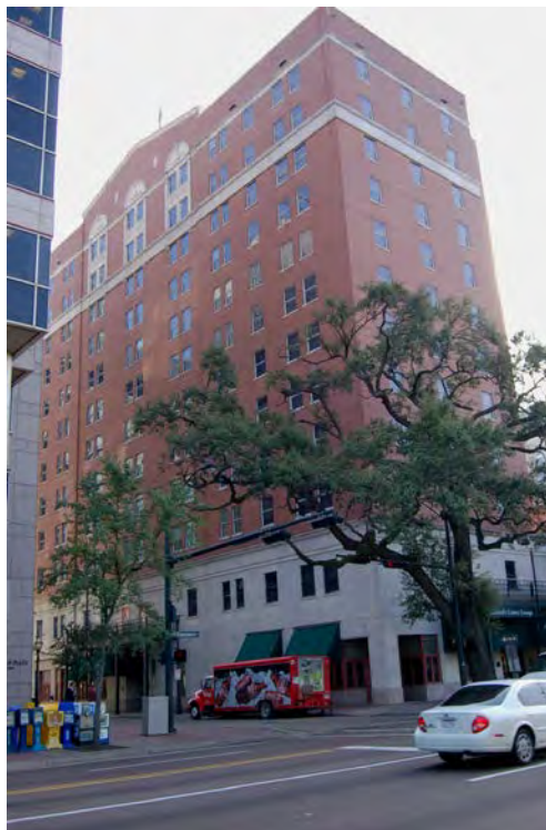
Figure 32-1. View to the southwest of the 1940 Admiral Semmes Hotel (Resource #32) at 251 Government Street in Church Street East Historic District.
