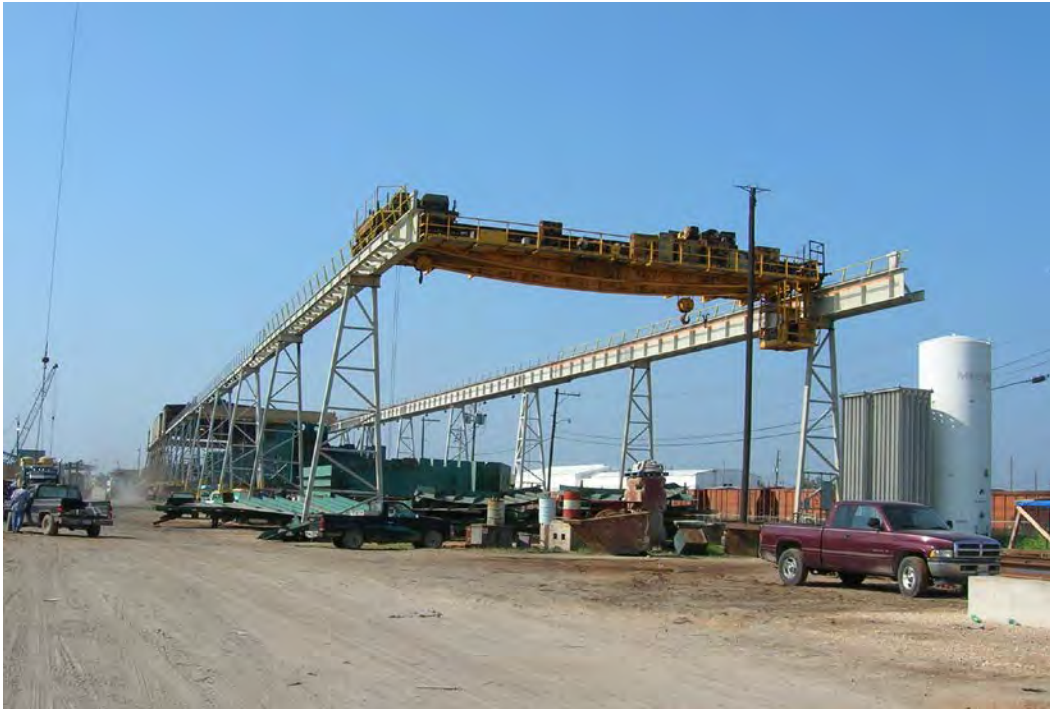
Figure 40. Structure 8, Hull Fabrication and Assembly Shop. View to the south.
