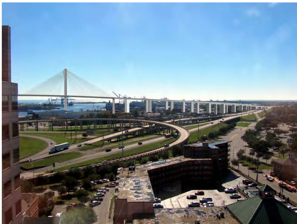
Figure 32-9. View to the south viewed from a 12th-floor room in Admiral Semmes Hotel (Resource #32). Due to distance (0.6 miles) and blockage by buildings (left), Alternate C (0.3 miles) would be partially visible (50%) above existing I-10 interchange.
