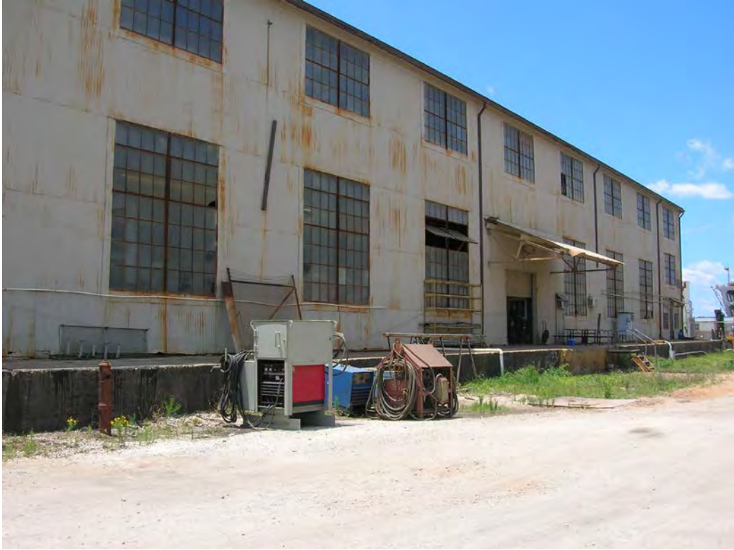
Figure 37. North side of Structure 12, Warehouse No. 3. View to the southwest.
