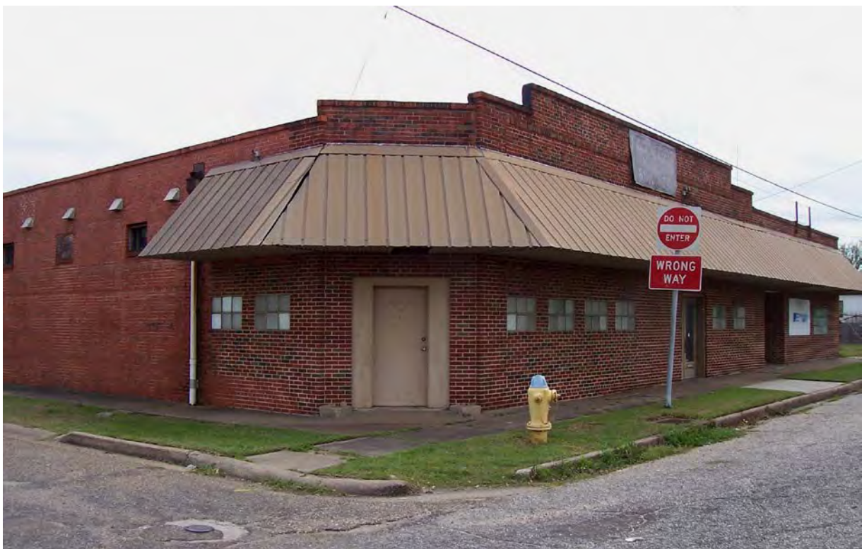
Figure 10. View to the southeast of Structure 7a, commercial building at 701 S. Conception Street on Survey Block 1.
