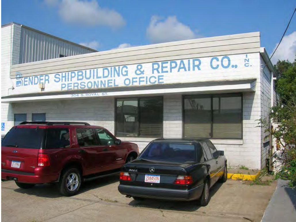
Figure 55. Structure 13, former Bender Shipyard Personnel Office. View to the west.
