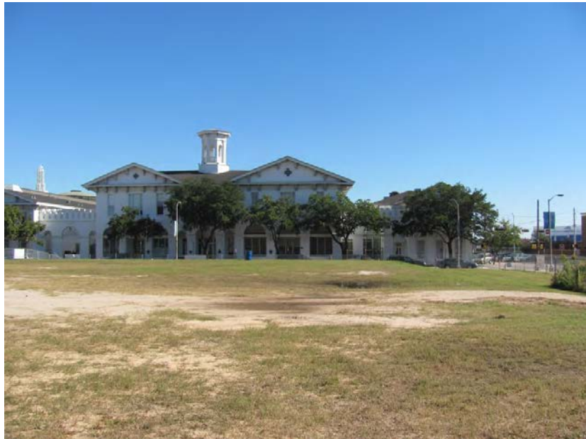
Figure 51-1. View to the east of Old Southern Market and City Hall (now Museum of Mobile) (Resource #51).
