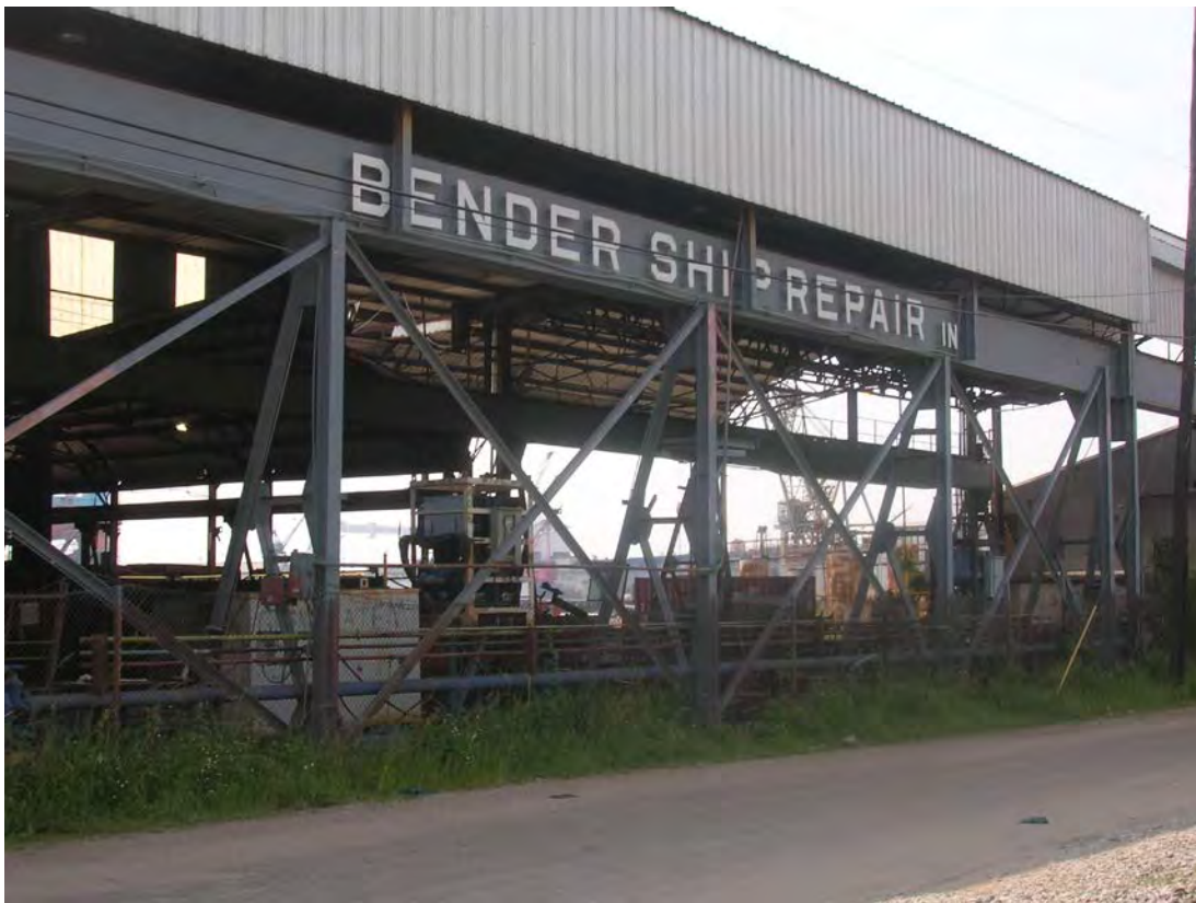
Figure 45. View to the southeast of the open workshop of former Bender Structure 3, Hull Fabrication Shop.
