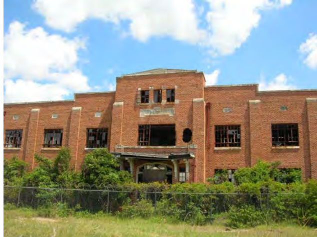
Figure 10. South façade and one of three entrances of Structure 1, Main Office. View to the north toward Alternate A, B, and B'.
