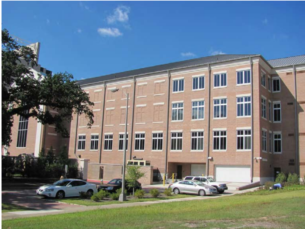
Figure 46-3. View to the northwest of the new four-story Probate Court Building on the north side of Christ Episcopal Church (Resource #46).
