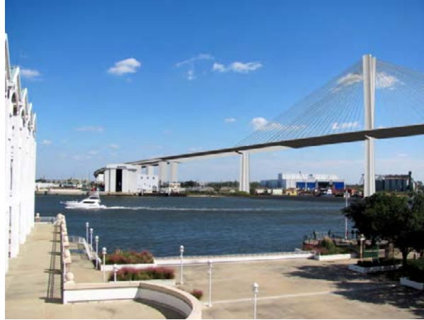
Figure 52-4. View to the east-southeast showing shipyards across the Mobile River on Blakeley Island from the second-story balcony on the south side of the Arthur R. Outlaw Mobile Convention Center (Resource #52). Alternate A would be visible (100%) from this location.
