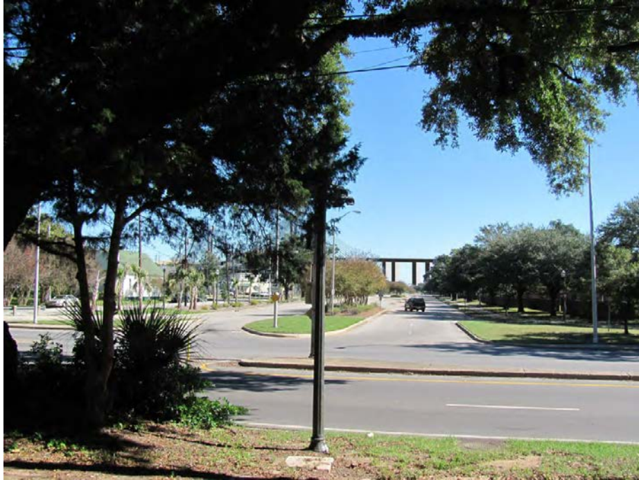
Figure 59-6. View to the east down Canal Street showing dense tree canopy and four-lane modern Canal Street. Alternate B (0.6 miles) would be partially visible (10-20%) from front of the historic structure at 162 S. Broad Street (Resource #59). Alternate B' would be similarly visible.
