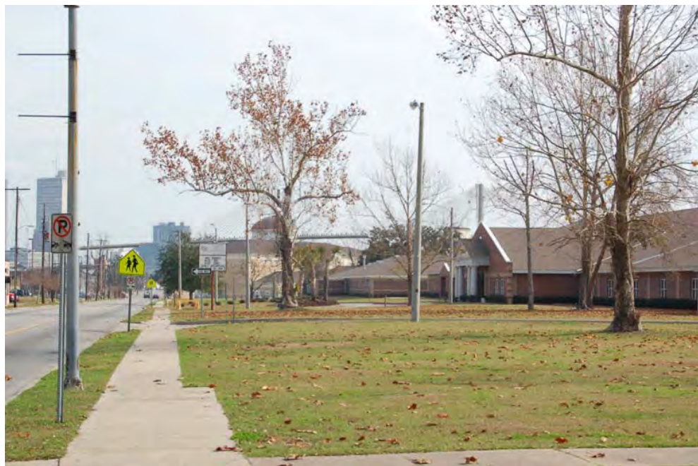
Figure 18-7. View to the southeast viewshed of the proposed I-10 Mobile River Bridge from the intersection of MLK Avenue and Kennedy Street (Resource #18) showing Alternate B', sparse canopy, Florence Howard Elementary School (right), one building on the Bishop State Community College campus (domed structure in center), and RSA-Bank Trust Building and Riverview Plaza Hotel (left). Due to distance (1.3-1.4 miles) and blockage by structures, Alternate B' would be partially visible (50%).
