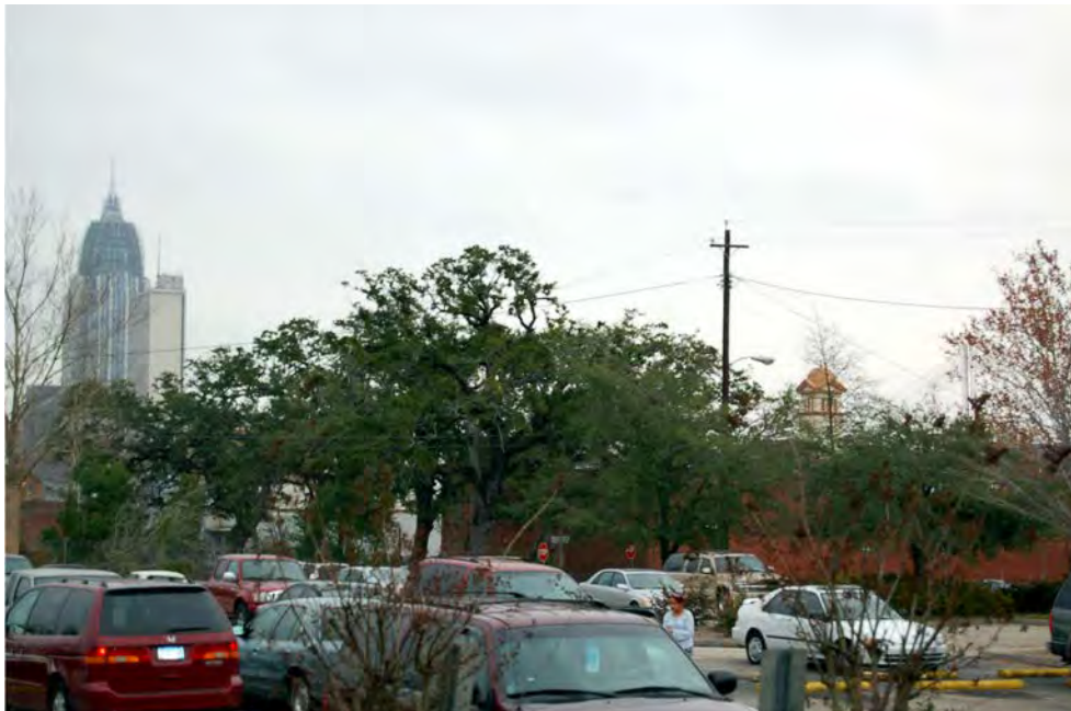
Figure 16-8. View from the east side of the United States Marine Hospital (Resource #16) to the east-southeast viewshed of the proposed I-10 Mobile River Bridge showing Alternate B (shown behind trees at right side of photograph), a mixture of historic and nonhistoric structures, the RSA Tower and RSA-Bank Trust Building (left), and moderate tree canopy. Due to distance (0.9 mile) and blockage by structures and tree canopy, Alternate B would be partially visible (10-15%) from the United States Marine Hospital.
