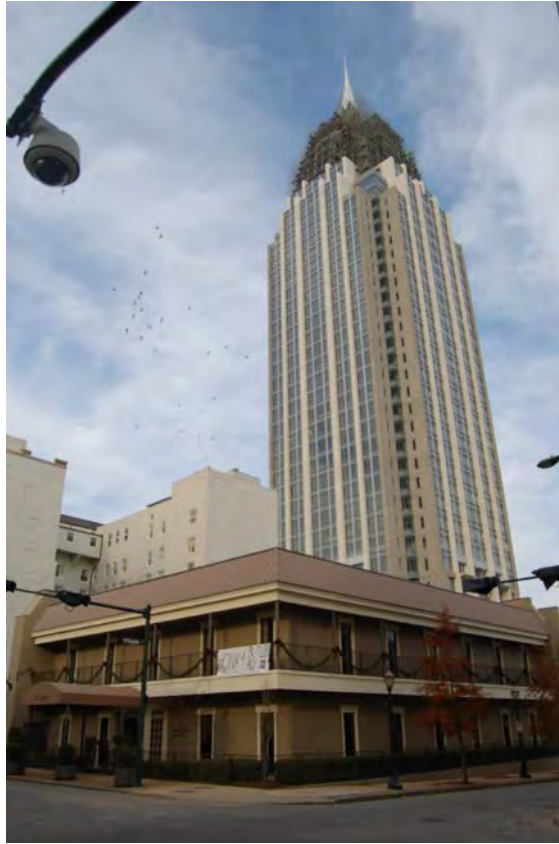
Figure 34-2. View to the northeast from the front of the Van Antwerp Building (Resource #34) showing the rear of the Battle House Hotel (left) and the RSA Tower (right) behind a two-story nonhistoric commercial building at the intersection of Dauphin and N. Royal Streets.
