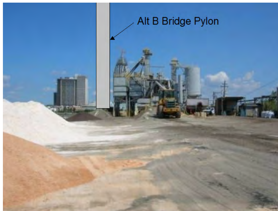
Figure 4. View to the north of the proposed location of Alternate B bridge pylon (where machinery owned by Mobile Abrasives is located), north of BAE Systems Southeast Shipyards.
