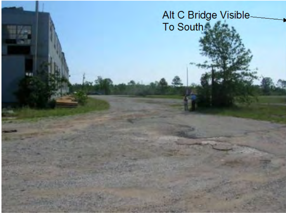
Figure 5. View to the east of the proposed route of Alternate C bridge route through the northern portion of BAE Systems Southeast Shipyards.
