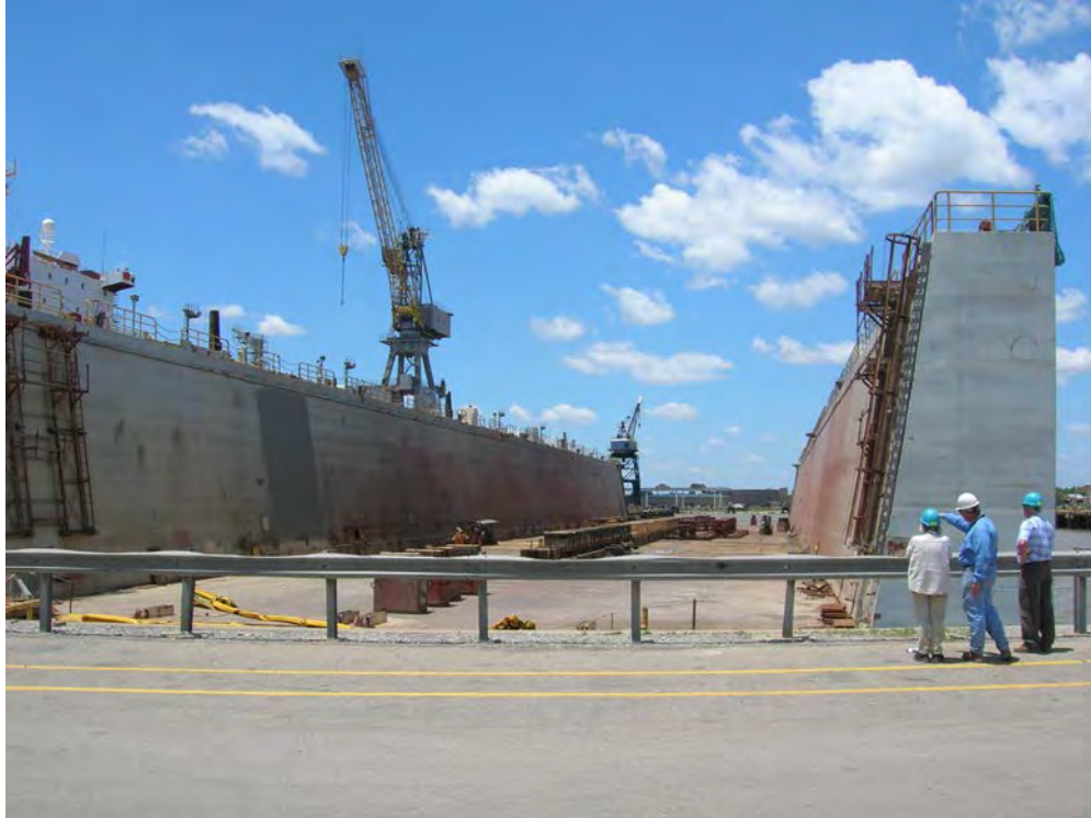
Figure 40. Structure 13, Dry Dock No. 17. View to the west toward Alternate C.
