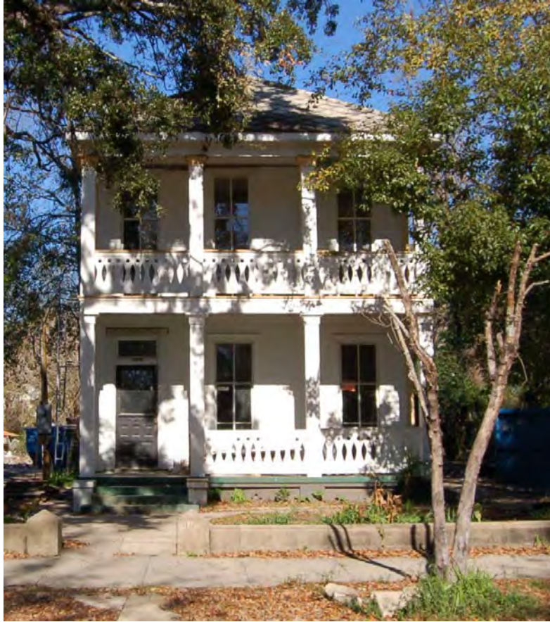
Figure 6-1. View to the north of the 1859 Cain-Werneth House (Resource #6) at 906 Palmetto Street in Oakleigh Garden Historic District.
