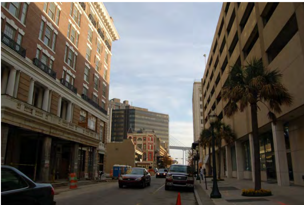
Figure 35-5. View from the Battle House Hotel (left) (Resource #35) to the south-southeast viewshed of the proposed I-10 Mobile River Bridge showing a mixture of historic and nonhistoric structures on N. Royal Street. Alternate A (0.4 miles) would be partially visible (10-20%) between the Riverview Plaza Hotel (left) and the Van Antwerp Building (Resource #34) and other buildings (right) from this location.
