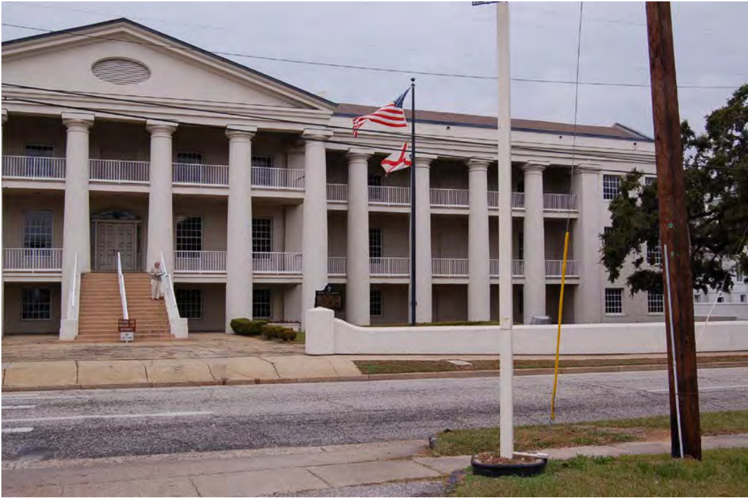
Figure 16-3. View to the north of City Hospital, built in Greek Revival style in 1830 as Mobile's third hospital, located on the block west of the United States Marine Hospital (Resource #16).
