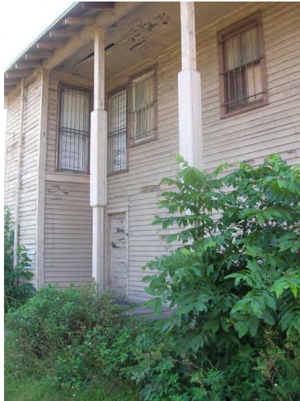
Figure 50. Rear of Structure 11, former Union Hall. View to the northeast.
