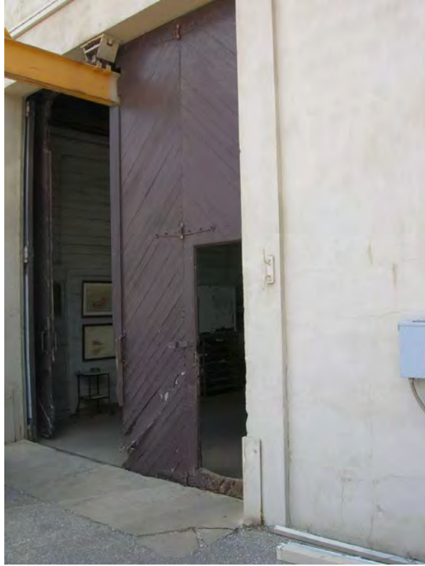
Figure 18. Original wooden door and overhead crane on Structure 4, electrical shop.
