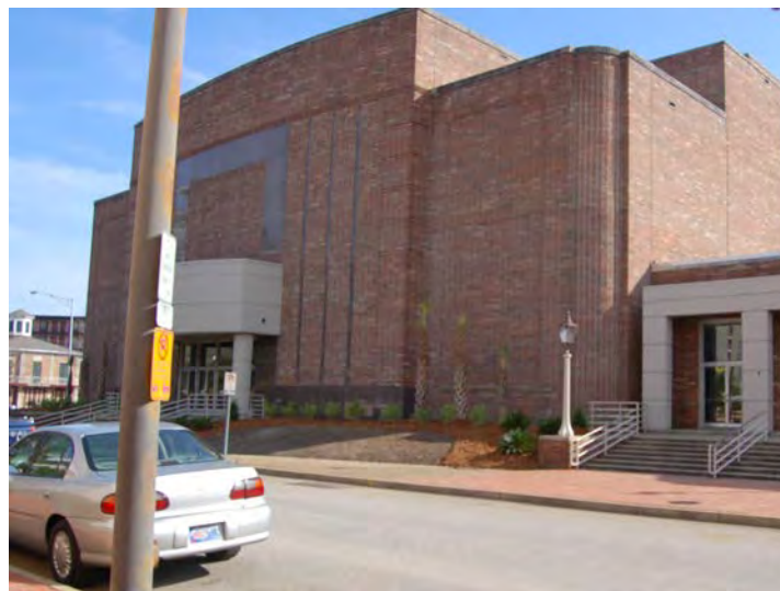
Figure 31-5. View to the southeast of Mobile Civic Center from the rear entrance of Malaga Inn (Resource #31).
