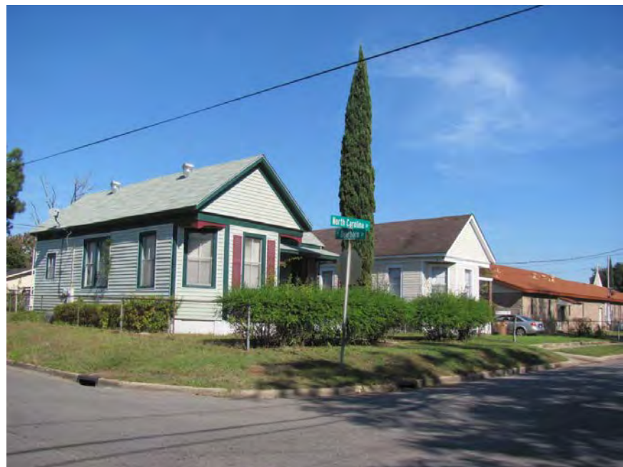
Figure 55-5. View to the northeast from the intersection of N. Carolina and S. Dearborn Streets (Resource #55) showing minimal tree canopy and two historic structures (left) and nonhistoric church (right) on N. Carolina Street. Due to distance (0.5 to 0.7 miles) and blockage by structures and tree canopy, Alternates A, B, B', and C would not be visible from the intersection of N. Carolina and S. Dearborn Streets (Resource #55).
