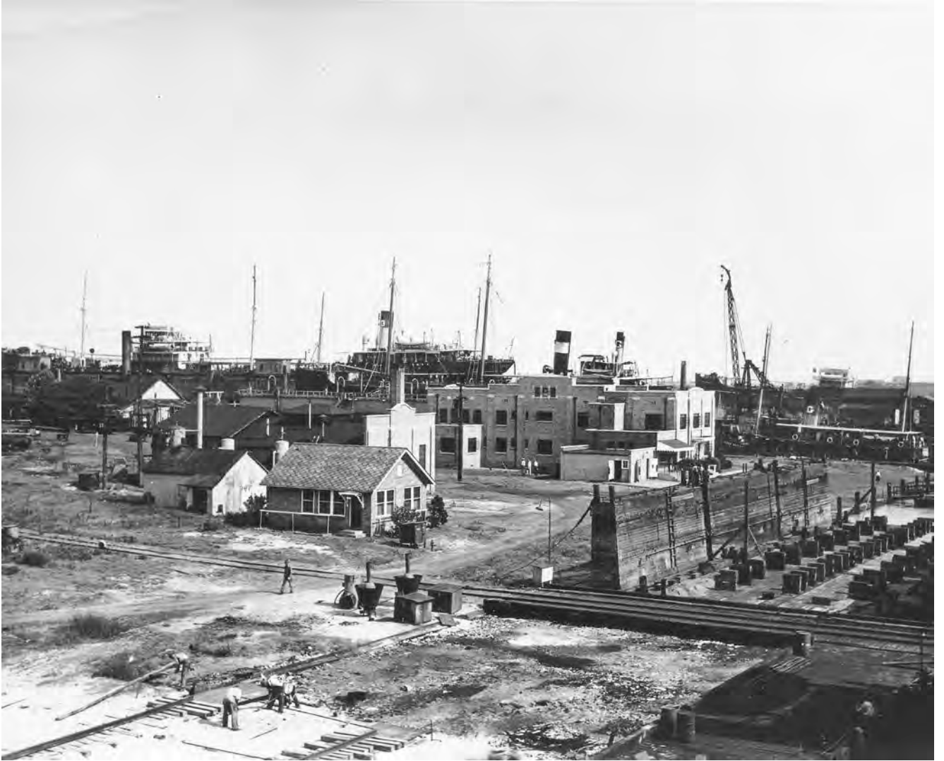
Figure 12. 1939 photograph of ADDSCO shipyard. View to the south showing Structure 1, main office, near the center of the photograph (ADDSCO Collection, University of South Alabama Archives).
