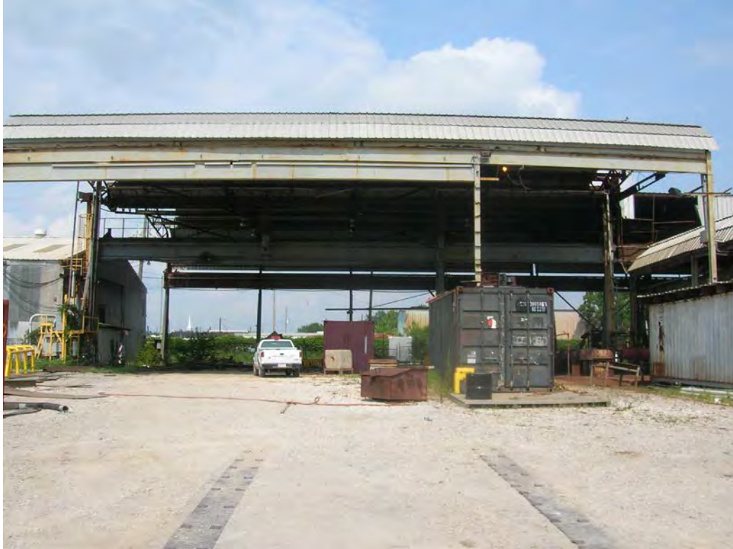
Figure 21. Open workshop of Structure 3, Hull Fabrication Shop. View to the west.
