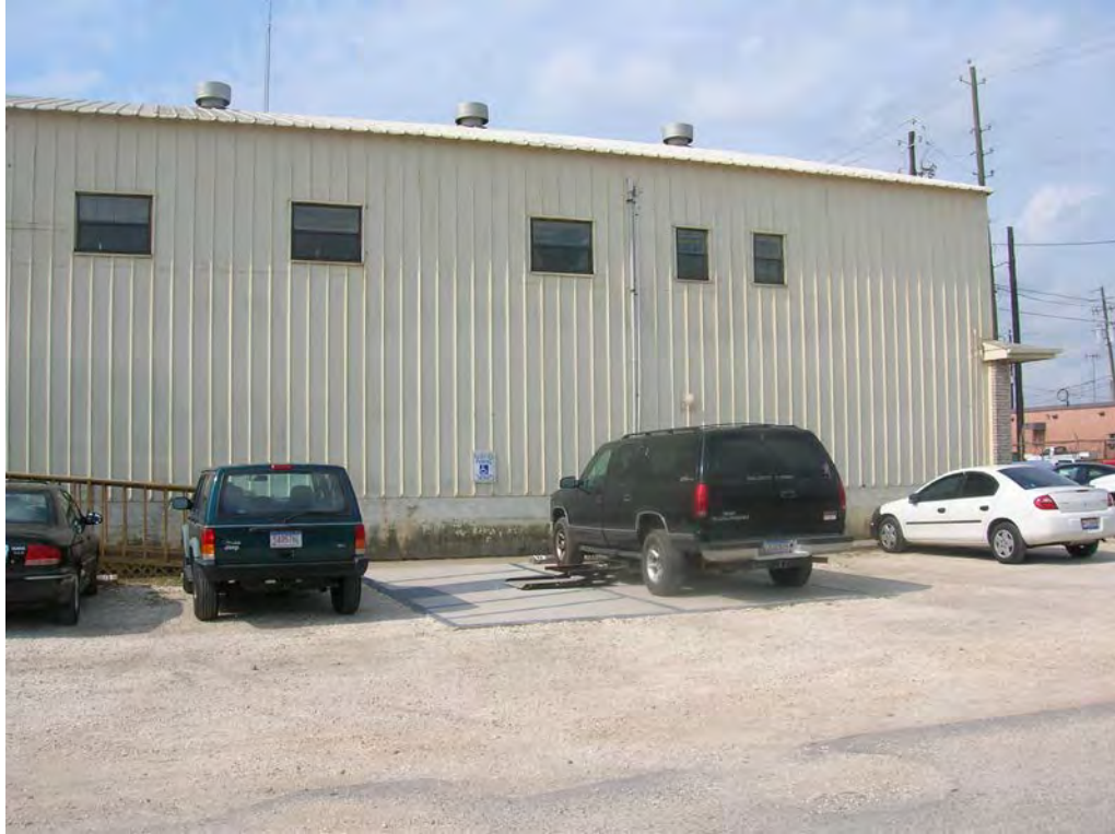
Figure 18. North side of Structure 2, Engineering, Planning & Safety Shop. View to the south.
