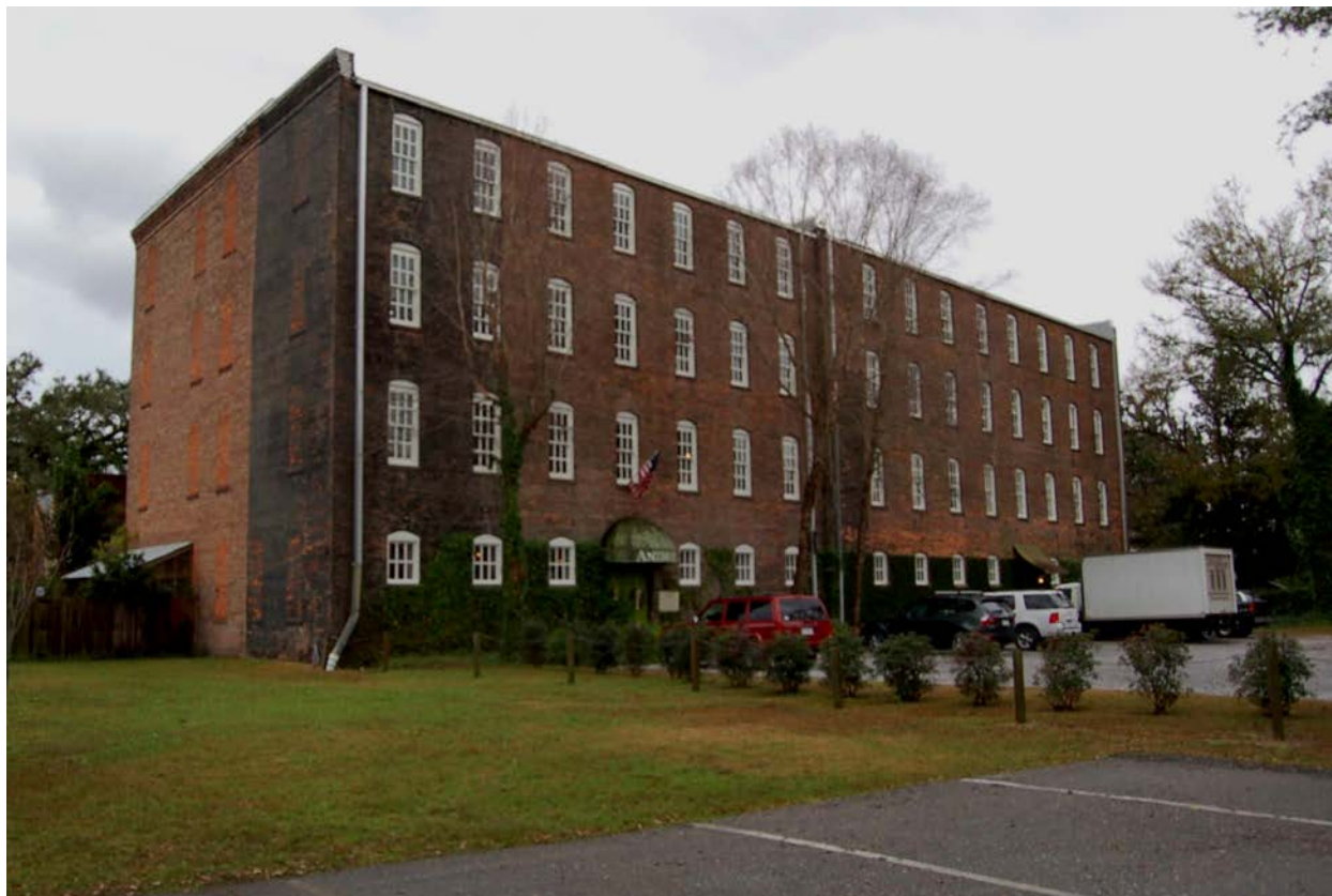
Figure 9-1. View to the southwest of the north side of the historic brick warehouse, now Atchison Imports European Antiques (Resource #9), at 921 Dauphin Street showing the bricked-up east windows (left).
