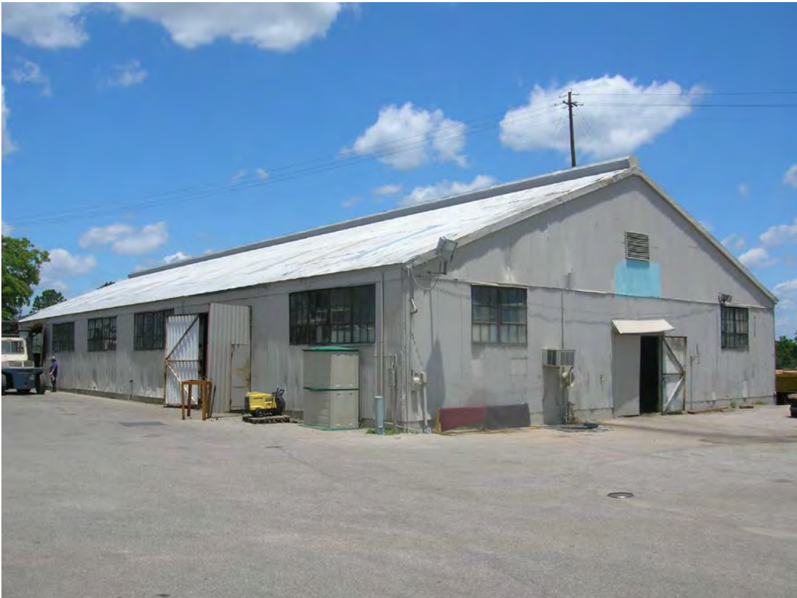
Figure 30. Structure 9, originally Carriage House, currently vehicle repair shop at BAE Systems Southeast Shipyards. View to the northeast.
