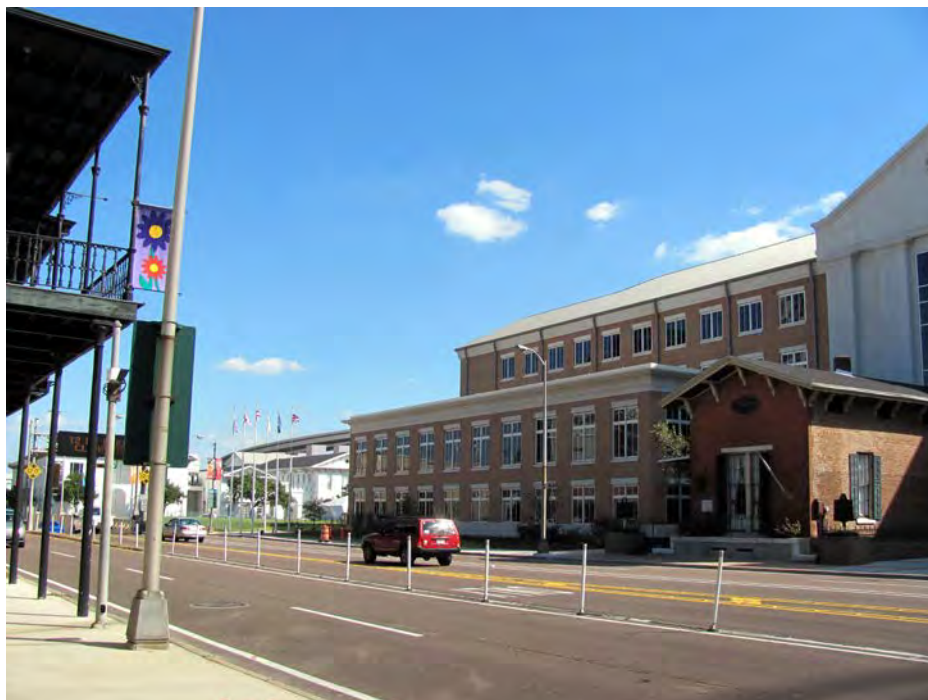
Figure 27-7. View from the intersection of Government and Conception Streets (Resource #27) to the southeast viewshed showing Alternate B' bridge route, and mixture of historic and nonhistoric structures. Due to distance (0.4 miles) and blockage by structures, Alternate B' would be partially visible (10%) above buildings from Resource #27. Alternate B would be similarly visible.
