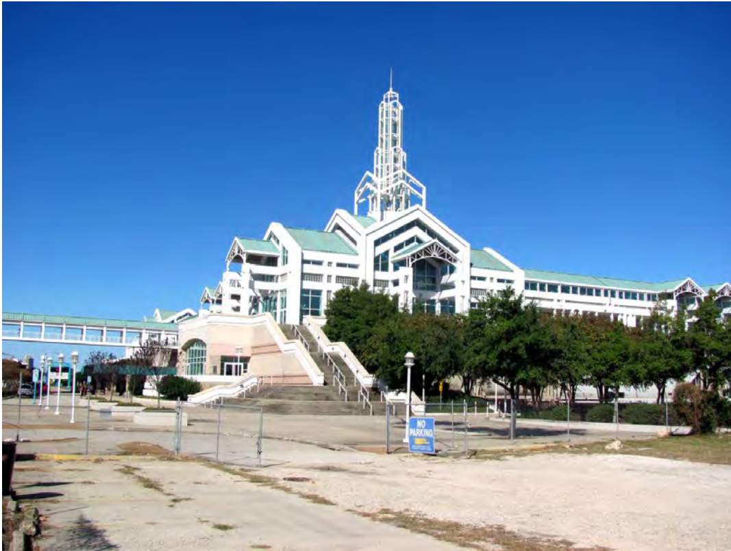
Figure 52-1. View to the north-northeast of Arthur R. Outlaw Mobile Convention Center (Resource #52) at 1 S. Royal Street.
