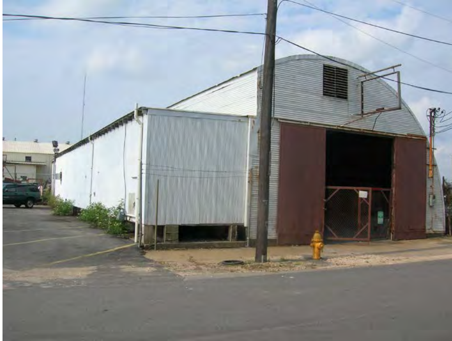
Figure 15. View to the southwest of the front of Structure 1, electrical maintenance shop for the former Bender Shipyard, on Eslava Street. Alternates B and B' bridge decks would cross immediately south of Structure 1.
