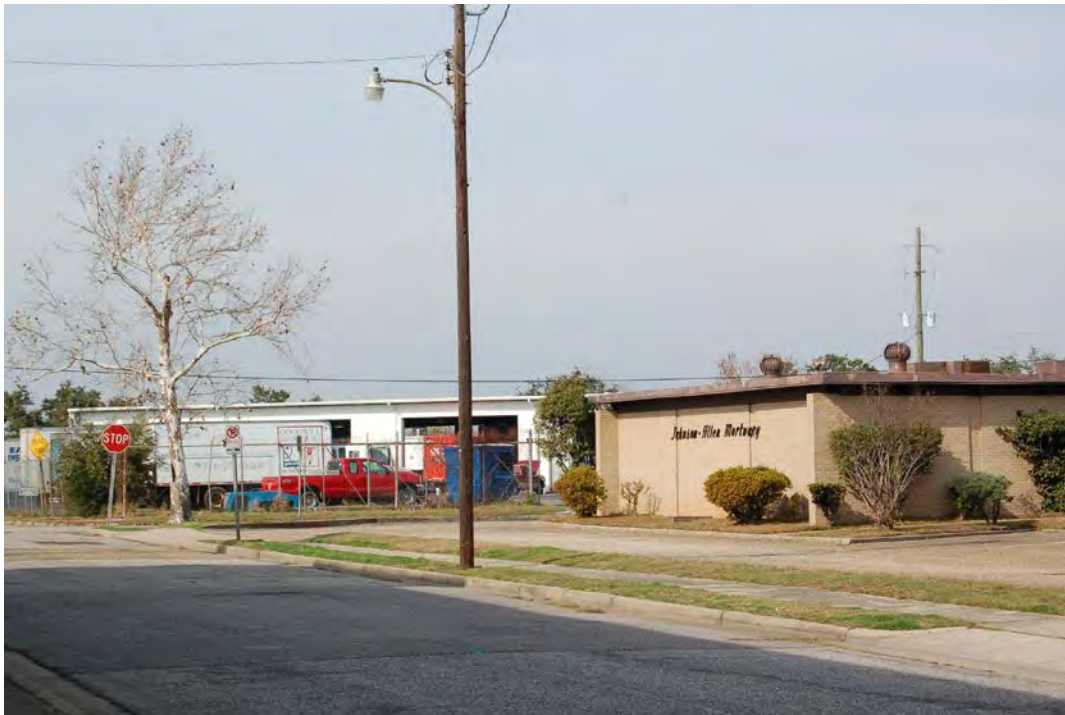
Figure 20-2. View to the north from the Stone Street Baptist Church (Resource #20) showing sparse tree canopy and two commercial buildings and associated paved parking lots.
