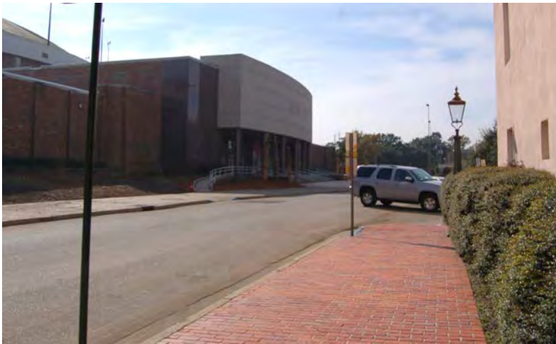
Figure 31-3. View to the west showing Mobile Civic Center (left), moderate tree canopy, and the rear of Malaga Inn (Resource #31) (right) on Civic Center Drive.
