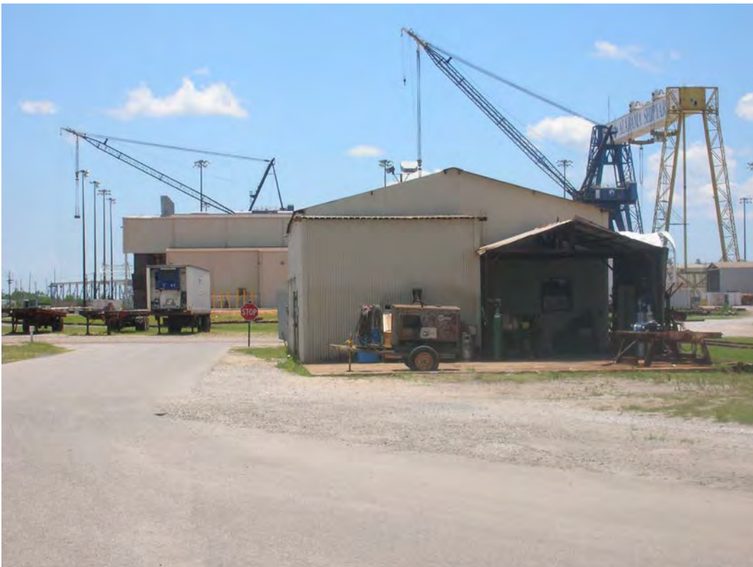
Figure 26. Structure 7, originally tractor repair shop, currently vehicle repair shop, at BAE Systems Southeast Shipyards. View to the south.
