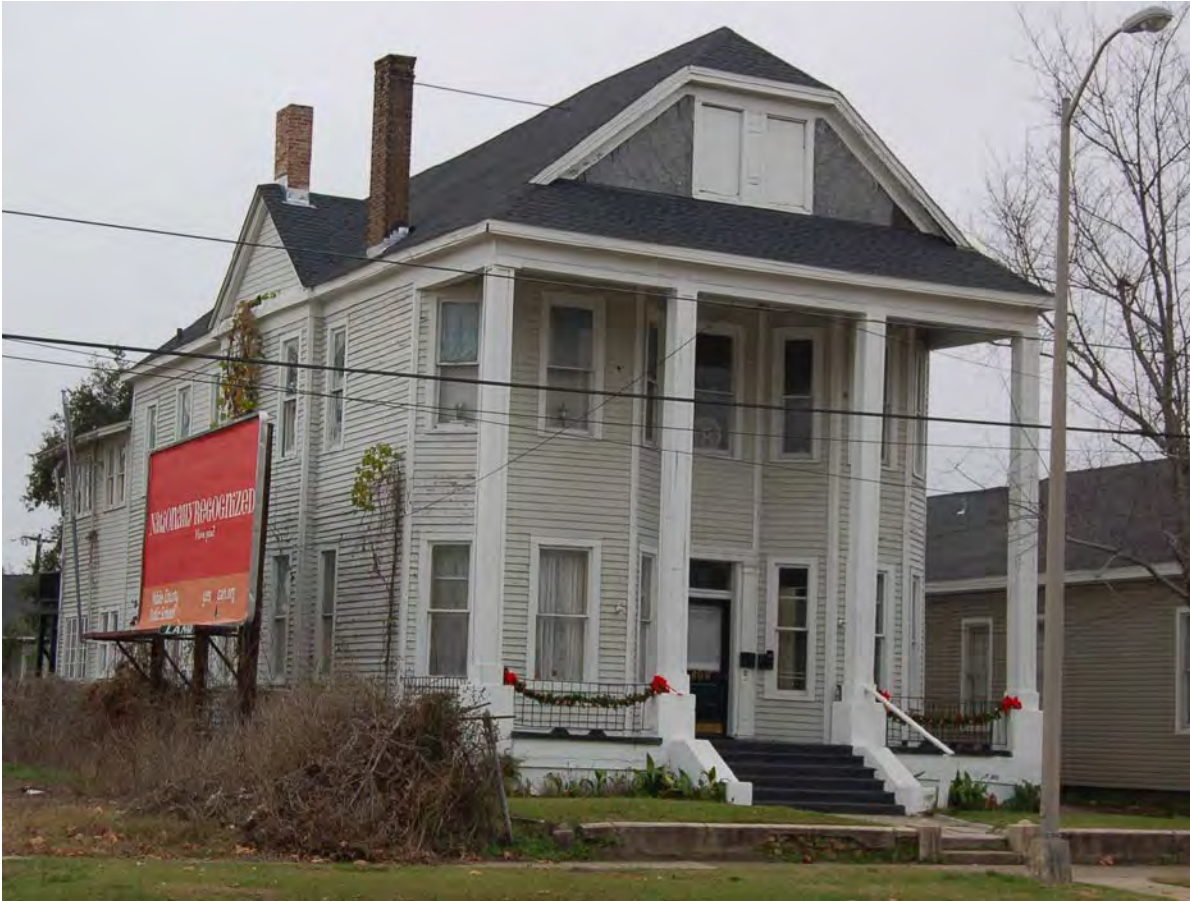
Figure 11-1. View to the southwest of the structure at 809 Springhill Avenue (Resource #11).
