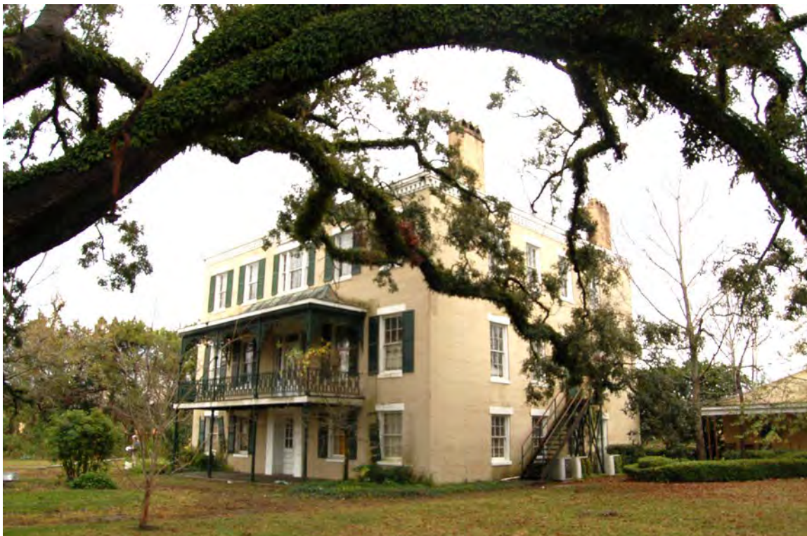
Figure 10-1. View to the southeast of the original 1845 portion of Protestant Orphans' Asylum, now known as Protestant Children's Hospital (Resource #10). Two-story front porch with ironwork added in the late 1800s or early 1900s.
