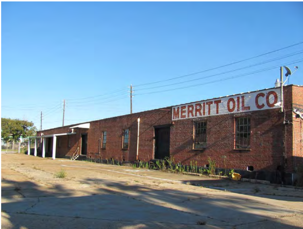
Figure 35. View to the north-northeast of Structure 20a, brick office and warehouse for Merritt Oil Company, Inc., at 401 North Carolina Street on Survey Block 23.
