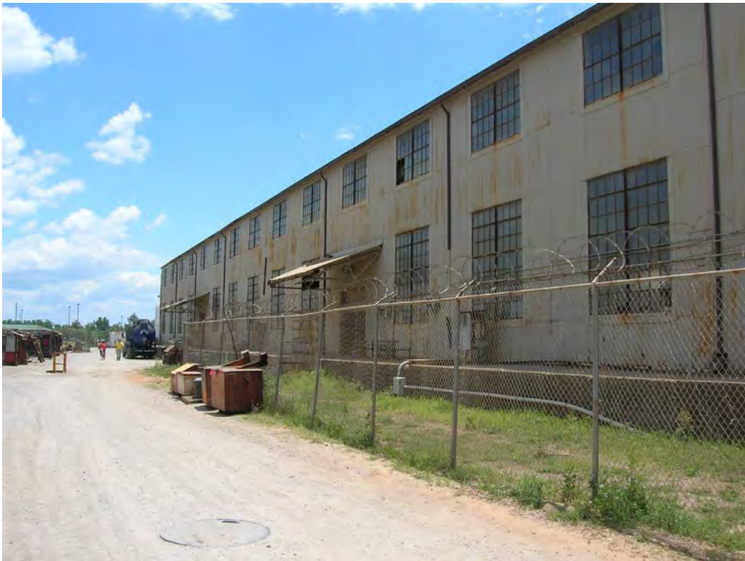
Figure 38. North side of Structure 12, Warehouse No. 3. View to the southeast.
