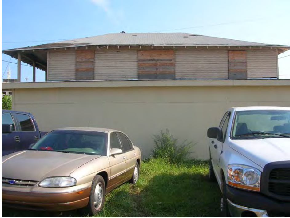
Figure 49. South side addition to Structure 11, former Union Hall. View to the north toward Alternate A.
