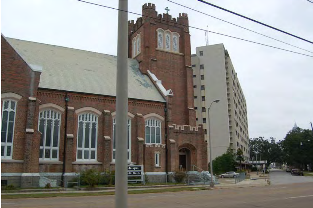
Figure 11-2. View to the northeast from the structure at 809 Springhill Avenue (Resource #11) showing St. Joseph's Catholic Church (Resource #12) (left), Tower on Ryan Park apartments (right), and Ryan Park with dense live oaks.
