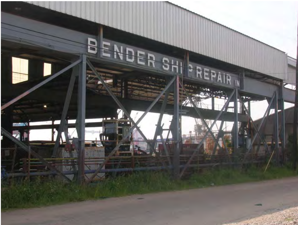
Figure 20. Open workshop of Structure 3, Hull Fabrication Shop for the former Bender shipyard. View to the southwest.
