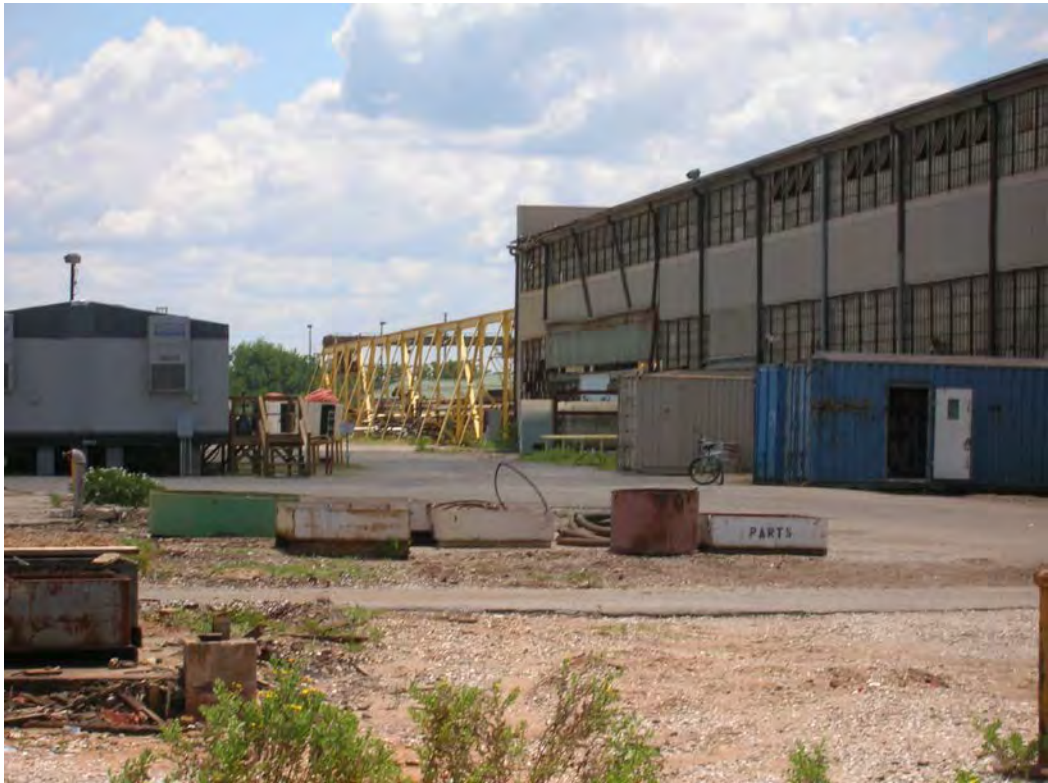
Figure 35. Overhead cranes at the rear of Structure 11, Machine Shop. View to the southeast.
