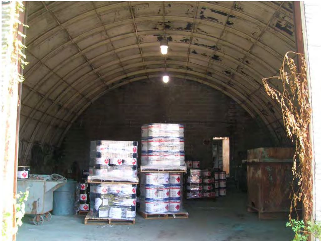
Figure 34. Interior of Structure 5, Quonset hut, originally Radcliff Gravel Company, former Bender Paint Kitchen. View to the north.
