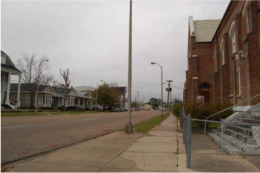
Figure 12-4. View to the west from St. Joseph's Catholic Church (Resource #12) (right), showing sparse tree canopy and row of historic houses (left) on south side of Springhill Avenue.
