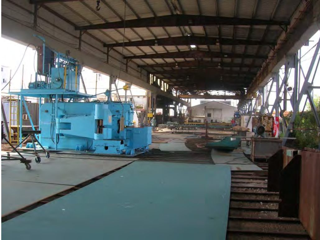
Figure 23. Open workshop of Structure 3, Hull Fabrication Shop. View to the south showing Structure 4, Machine Shop, in background.
