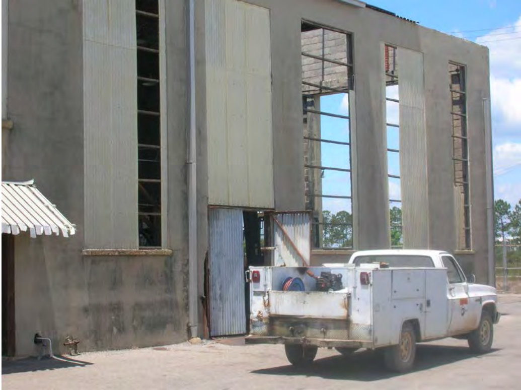
Figure 29. Structure 8, maintenance building. View to the northwest.
