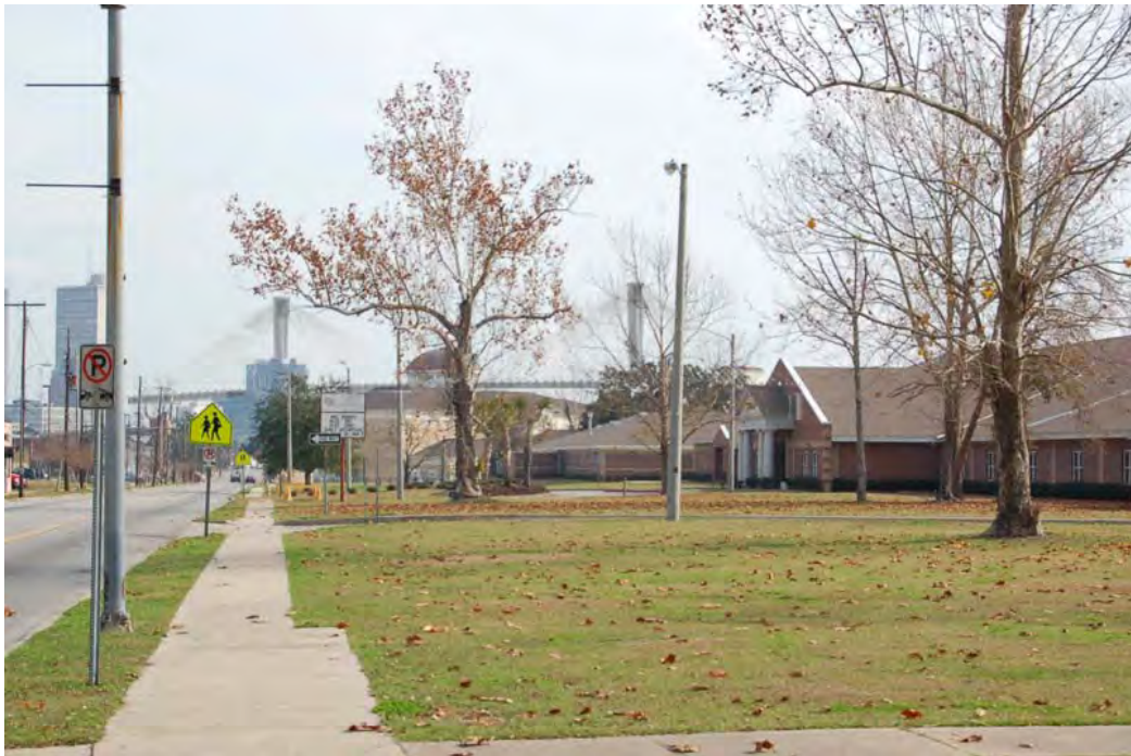
Figure 18-5. View to the southeast viewshed of the proposed I-10 Mobile River Bridge from the intersection of MLK Avenue and Kennedy Street (Resource #18) showing Alternate A, sparse canopy, Florence Howard Elementary School (right), one building on the Bishop State Community College campus (domed structure in center), and RSA-Bank Trust Building and Riverview Plaza Hotel (left). Due to distance (1.3-1.4 miles) and blockage by structures, Alternate A would be partially visible (50%).
