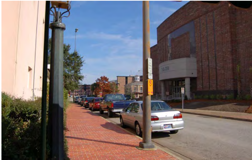
Figure 31-7. View from rear entrance of Malaga Inn (Resource #31) to the east-southeast of the proposed I-10 Mobile River Bridge showing Alternate B' (0.3 mile) which would be partially visible (10%) (center of photograph) above structures in the distance down Civic Center Drive.
