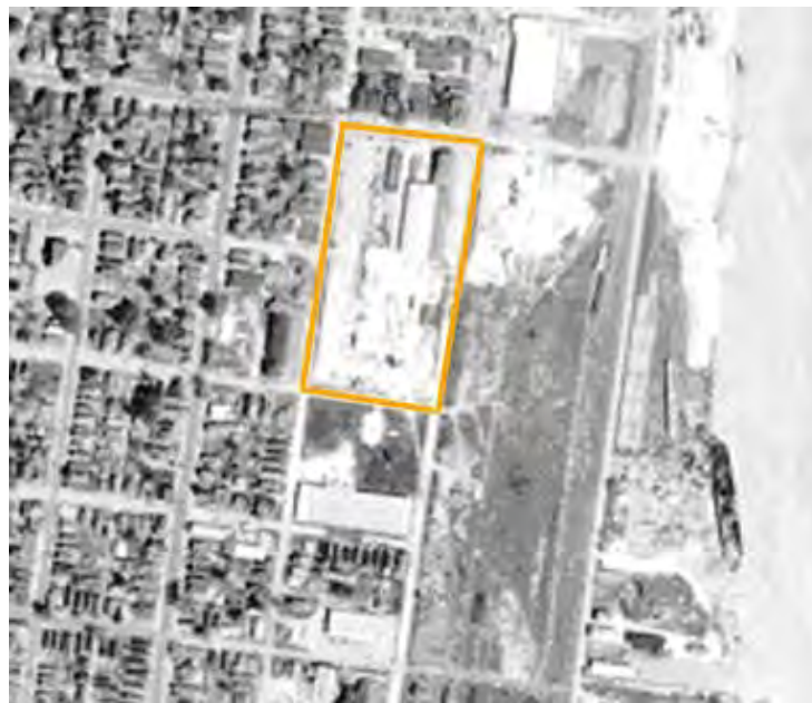
Figure 26. Detail of a 1950 aerial view between Charleston and Elmira streets and east from S. Franklin Street showing a mixture of residential and industrial development (UA 2006). The highlighted portion is the site of the ephemeral GM&N rail yard. In fact, faint indications of both the GM&N and L&N rail lines can be seen on the commercially-developed areas in this photograph.
