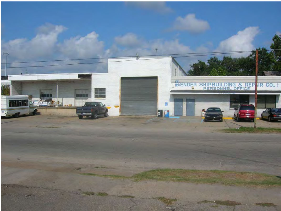
Figure 48. View to the west of former Bender Structure 13, Shipyard Personnel Office and Warehouse.
