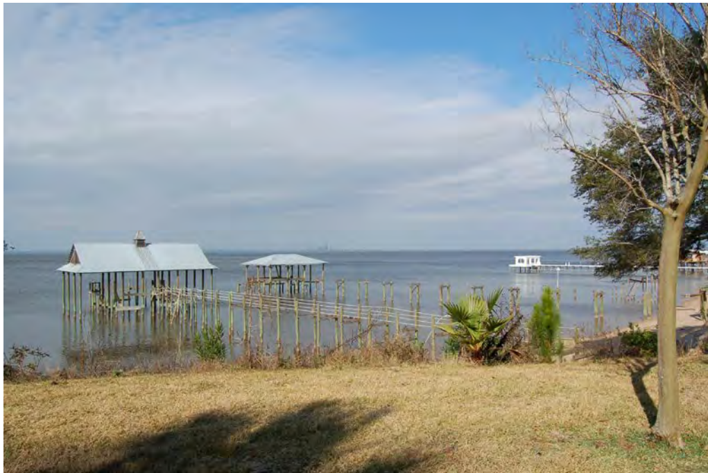
Figure 38-5. View to the northwest viewed of the proposed I-10 Mobile River Bridge showing Alternate A from the front of the Captain Adams-Stone House (Resource #38). The RSA Tower, RSA-Bank Trust Building, and downtown Mobile at a distance of 9.0 miles are barely visible on the horizon near the center of the photograph. At this distance, Alternates A, B, B', and C would barely be visible and would not result in viewshed impacts.
