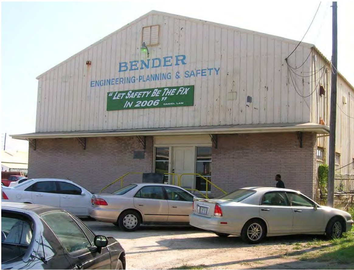
Figure 44. View to the east of the front of former Bender Structure 2, Engineering, Planning & Safety Shop.
