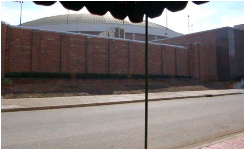
Figure 31-4. View to the southwest of Mobile Civic Center from the rear entrance of Malaga Inn (Resource #31).
