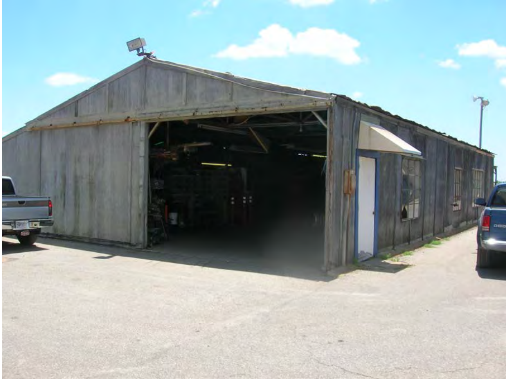
Figure 24. Front of Structure 6, originally auto repair shop, currently tool storage shed. View to the southeast.
