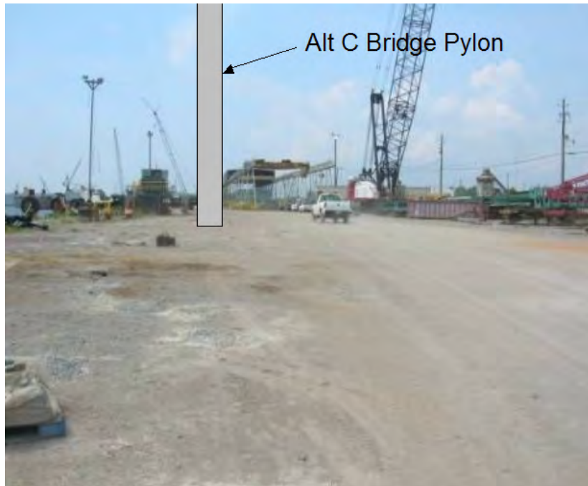
Figure 8. View to the south of the proposed location of Alternate C bridge pylon in an open area in the central portion of the former Bender Shipbuilding & Repair Company, Inc.
