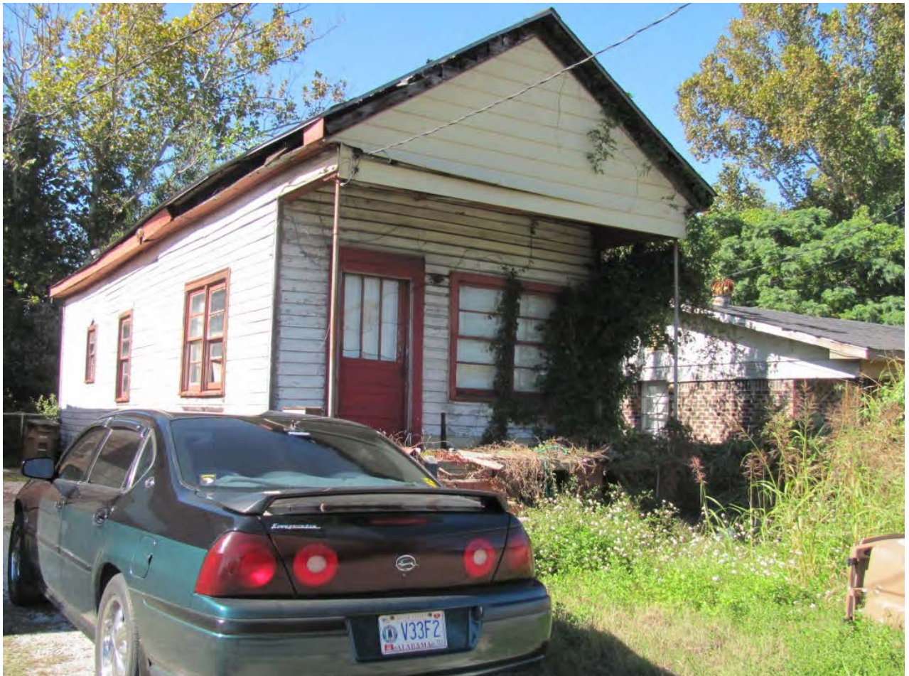
Figure 38. View to the west-northwest of Structure 21, shotgun house at 918 S. Hamilton Street on Survey Block 25.
