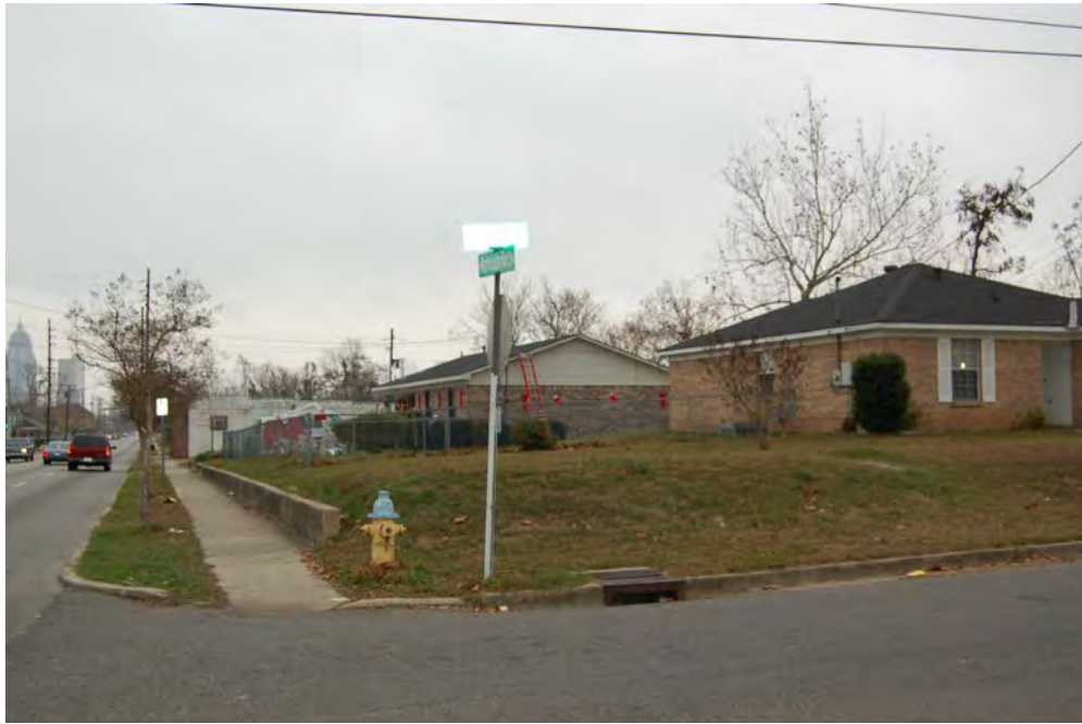
Figure 19-6. View to the east-southeast viewshed of the proposed I-10 Mobile River Bridge from the intersection of MLK Avenue and Hickory Street (Resource #19) showing Alternate B (behind trees above white flat roofed building on left side of photograph), a sparse tree canopy, new homes, and the RSA Tower and RSA-Bank Trust Building (left). Due to distance (1.6-1.7 miles) and blockage by structures, Alternate B would be partially visible (10-15%) from this intersection.
