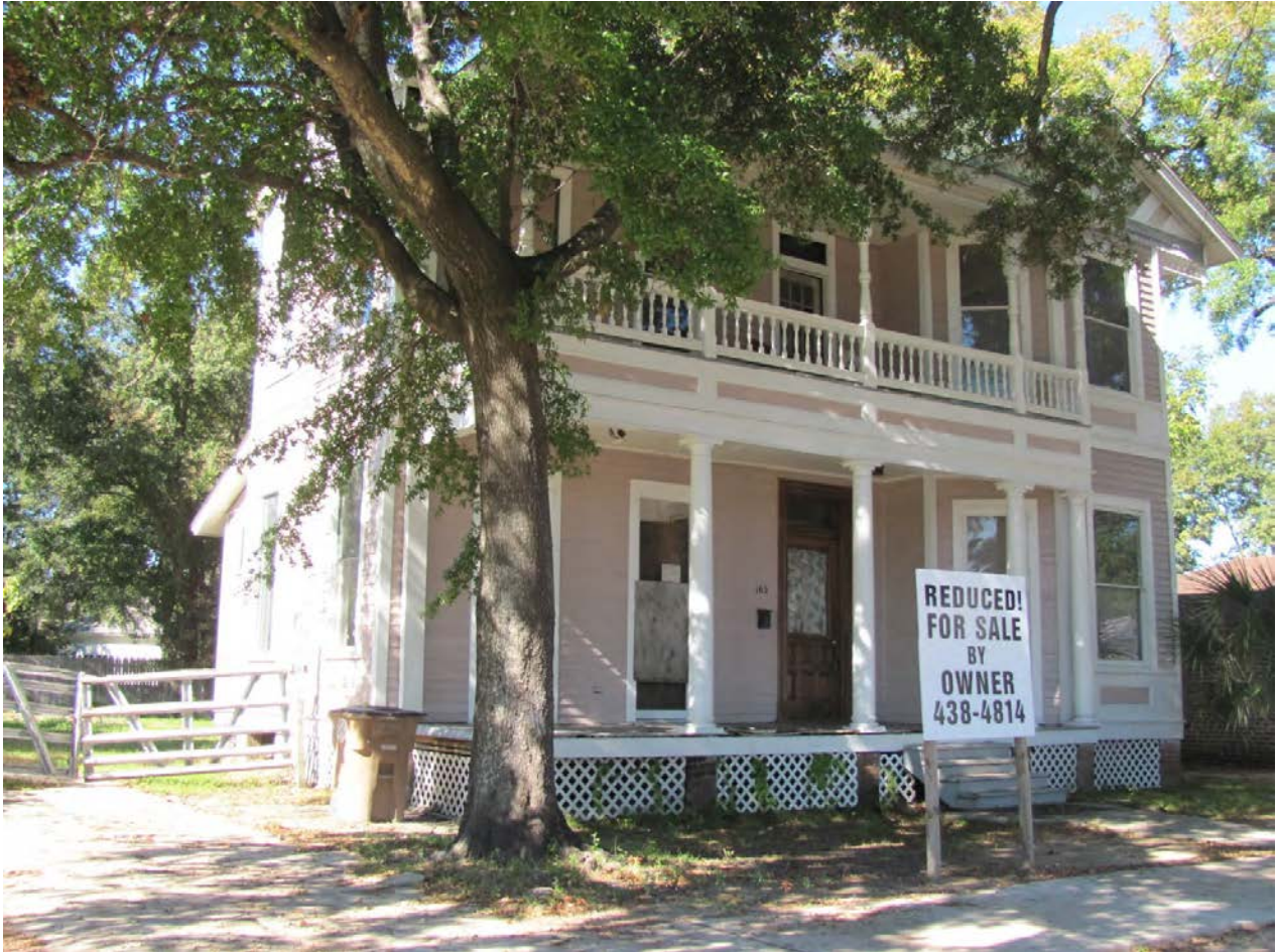
Figure 59-1. View to the west of historic structure at 162 S. Broad Street (Resource #59) in the Oakleigh Garden Historic District.
