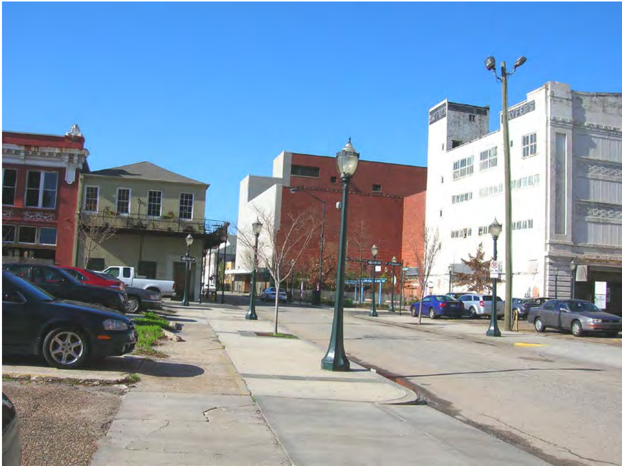
Figure 26-1. View to the west of the intersection of St. Emanuel and Conti Streets (Resource #26) in the heart of downtown Mobile.
