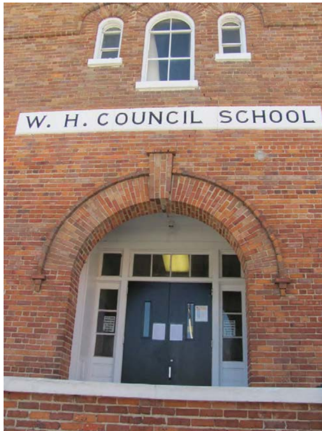
Figure 41-2. The original front of W. H. Council School (Resource #41) on the east side of the structure.
