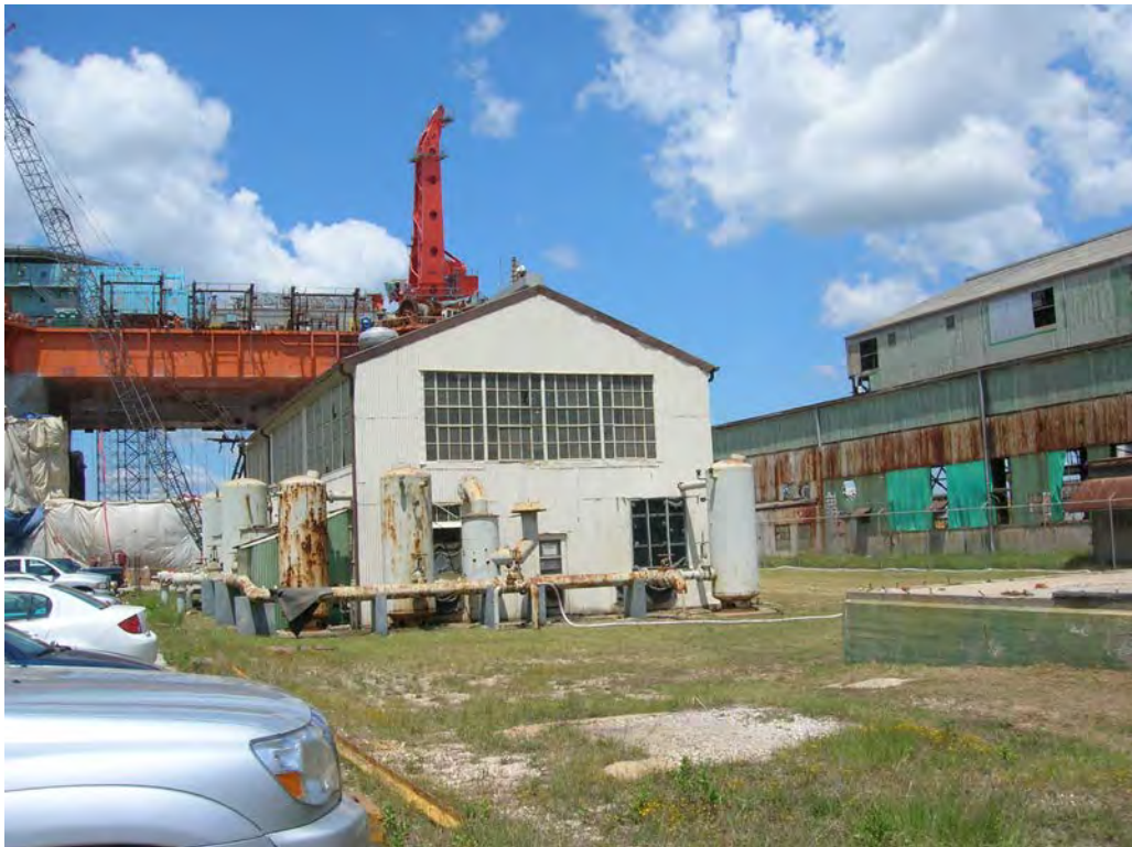
Figure 16. Rear of Structure 3, originally tool house, currently pump house. View to the west toward Alternate C.
