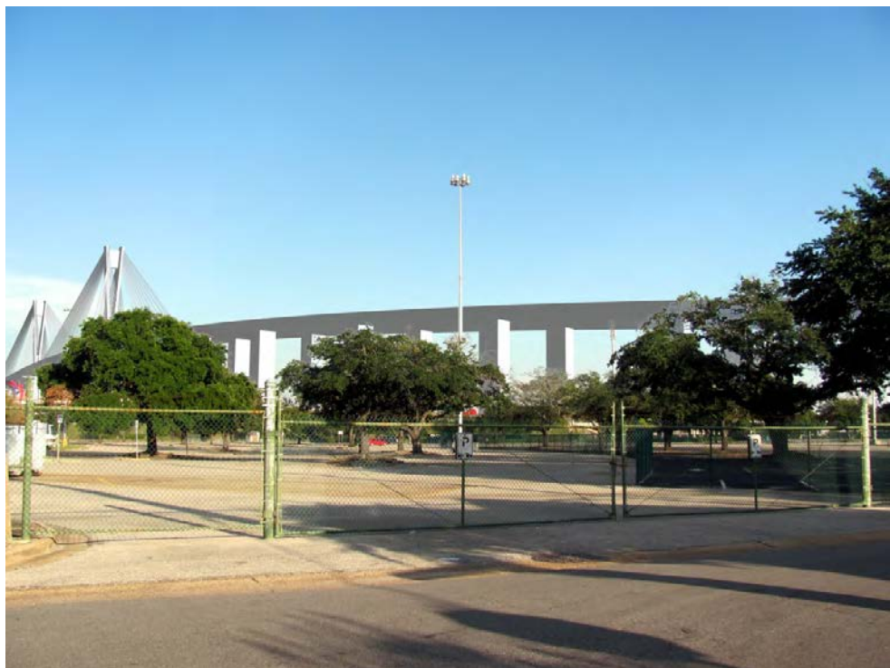
Figure 44-5. View to the southeast showing moderate tree canopy, Mobile Civic Center parking lot, and Alternate A (0.2 miles) which would be partially visible (50-60%) from the intersection of S. Lawrence and Eslava Streets (Resource #44).
