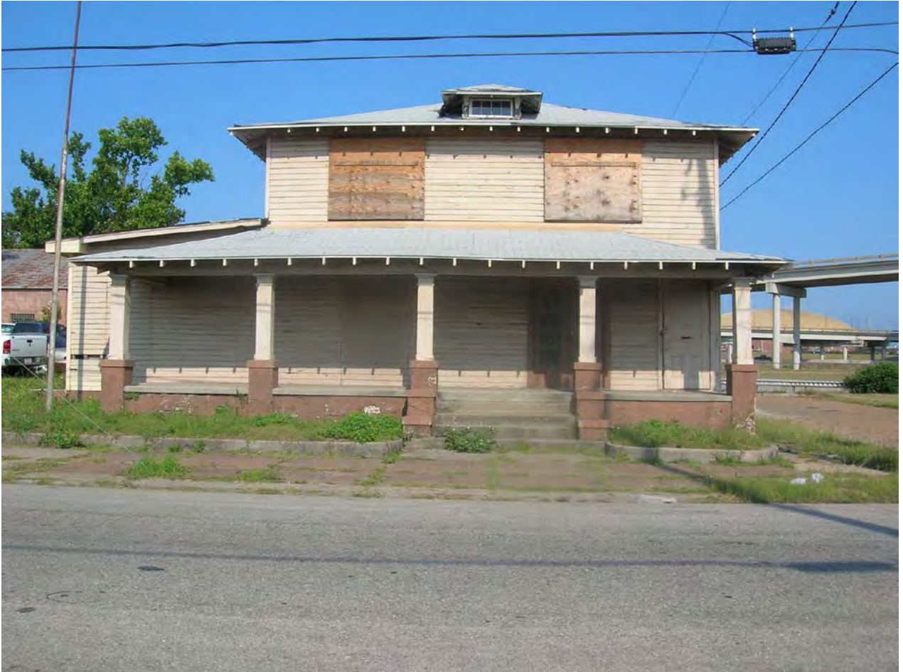
Figure 48. Structure 11, originally built as a residence and used as a “Union Hall” for shipyard workers during the mid-twentieth century, on S. Royal Street. It last served as a File Storage building for the former Bender Shipyard. View to the west toward Alternate A. Alternates B and B’ would cross immediately south of Structure 11. Alternate C would be located approximately 0.28 mile south of Structure 11.
