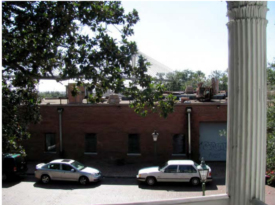
Figure 49-7. View to the south from the second-story front balcony of Condé-Charlotte Museum House (Resource #49) showing moderate tree canopy and nonhistoric brick commercial structure across Theater Street. Alternate C (0.5 miles) would be partially visible (20-30%) from this location.
