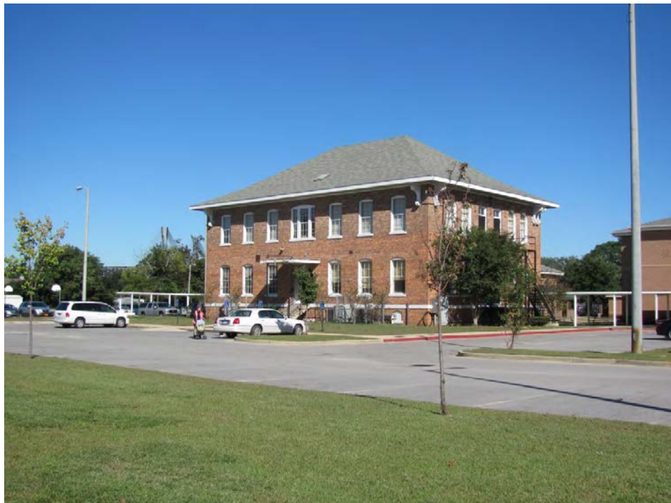
Figure 41-5. View to the northeast viewshed of the proposed I-10 Mobile River bridge showing moderate tree canopy and parking lots around W. H. Council School (Resource #41). Alternate C (0.4 miles) would be partially visible (20%) above the trees (left of school in photograph).
