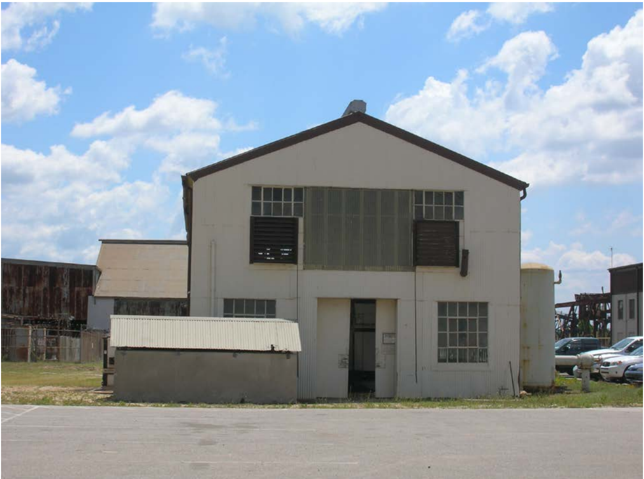
Figure 14. Front of Structure 3, originally tool house, currently pump house, at BAE Systems Southeast Shipyards. View to the east.
