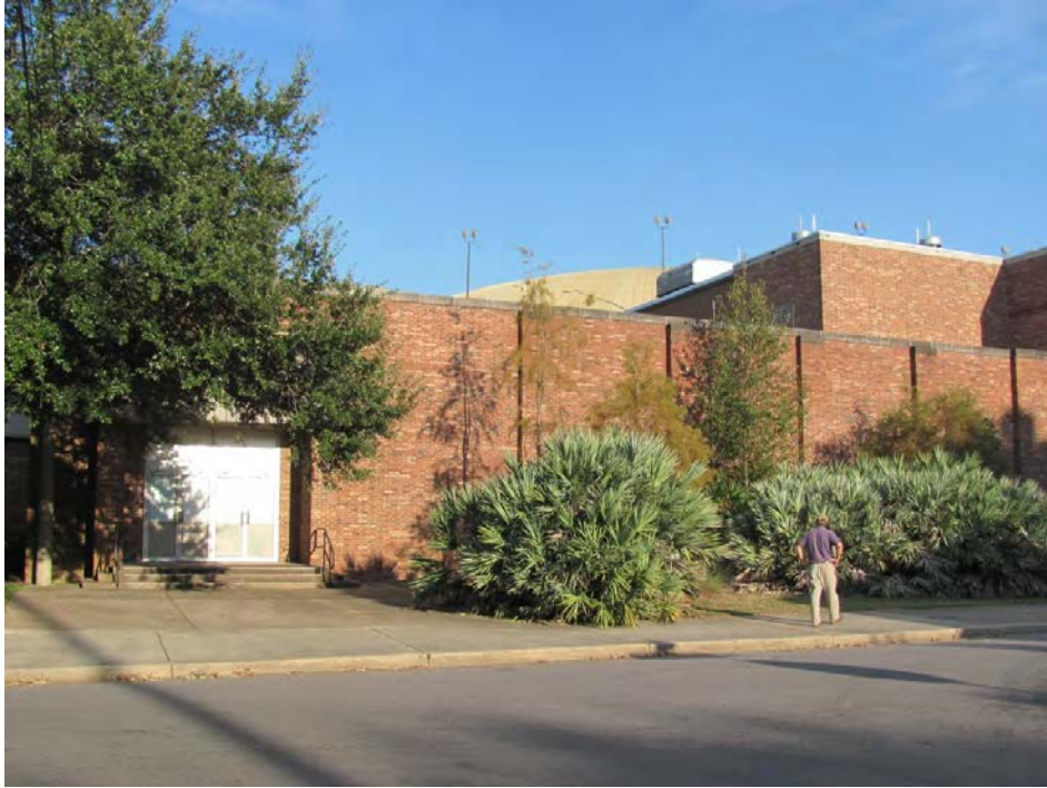
Figure 47-4. View to the east from the intersection of S. Lawrence and Monroe Streets (Resource #47) with moderate tree canopy and the Mobile Civic Center on S. Lawrence Street.
