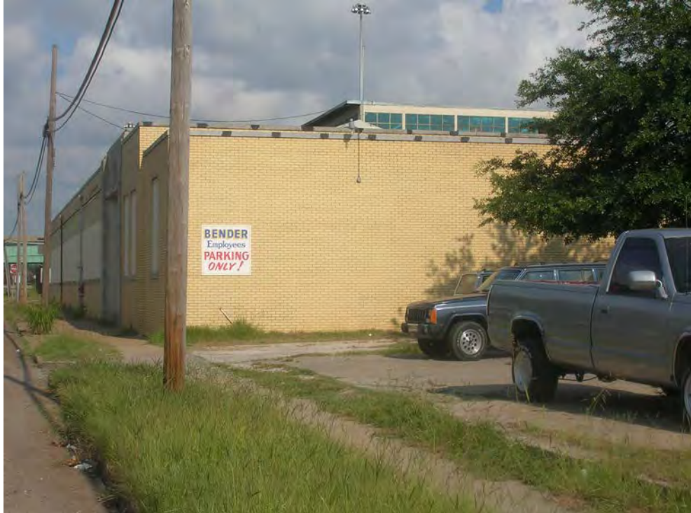
Figure 60. Structure 14, originally Mobile Linen Supply Company, later the National Linen Service Corporation, and last used as Warehouse No. 10 for the former Bender Shipyard. View to the northwest toward Alternates A, B, and B'.
