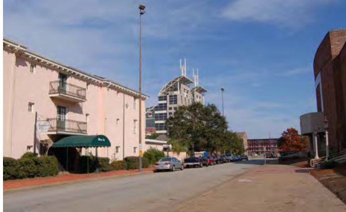
Figure 31-1. View to the northeast of the rear entrance (left) to Malaga Inn (Frohlichstein-Goldsmith Houses) (Resource #31) on Civic Center Drive in Church Street East Historic District. Also shown are Government Plaza (center) and Mobile Civic Center (right).
