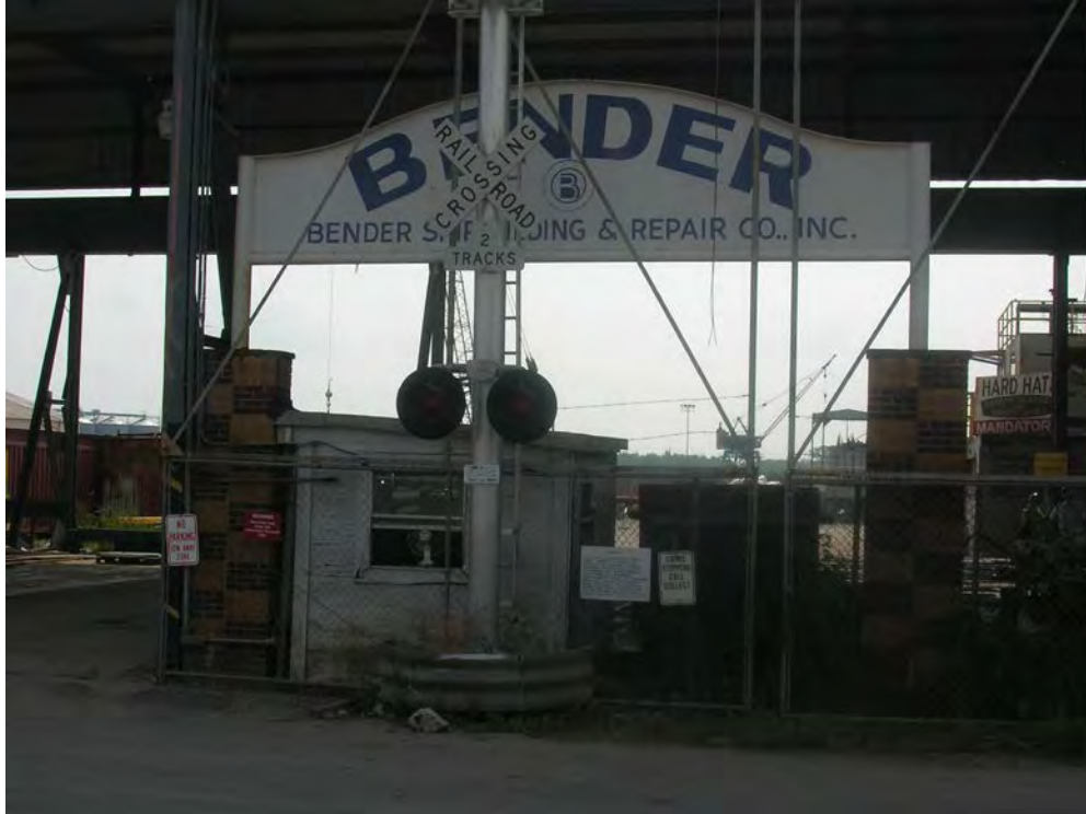
Figure 25. Original company sign at entrance to open workshop of Structure 3, Hull Fabrication Shop. View to the east toward the Mobile River.
