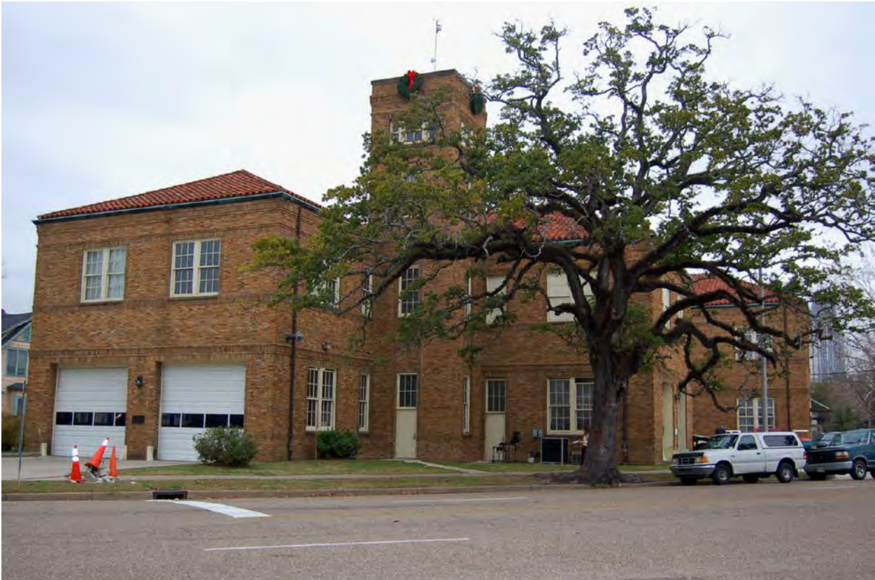
Figure 14-1. View to the northeast of Central Fire Station (Resource #14) at 701 St. Francis Street in the Lower Dauphin Historic District. RSA Tower is visible through the trees (right).
