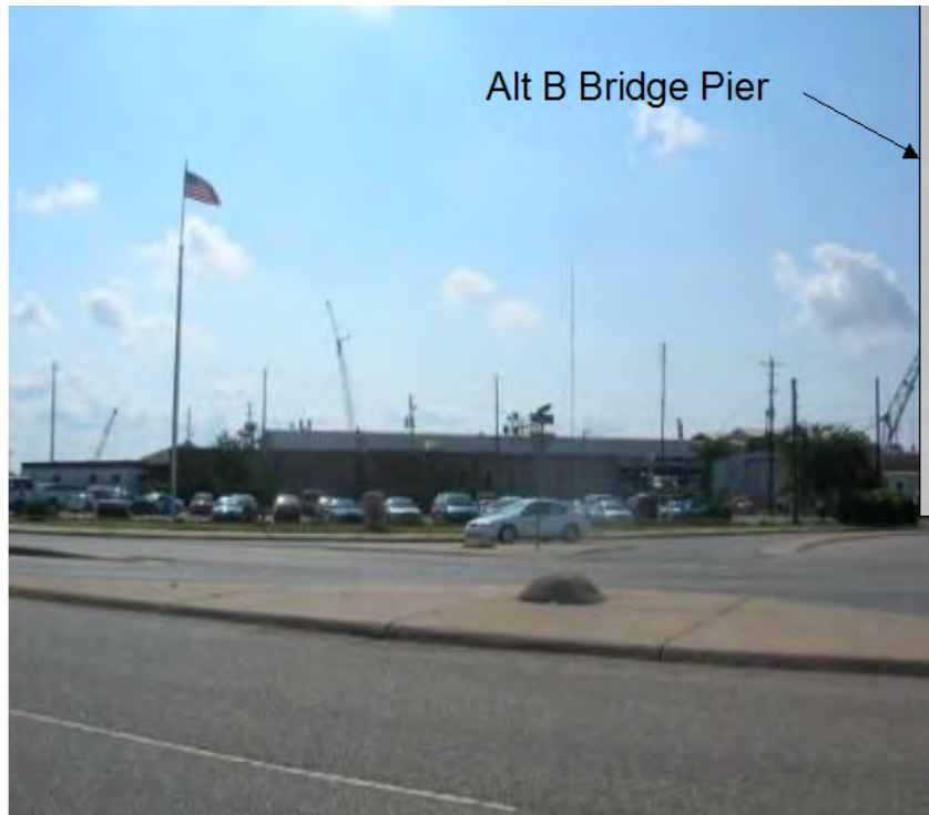
Figure 6. View to the east towards the Mobile River of the proposed location of Alternate B bridge pier south of the parking lot for the main offices of the former Bender Shipbuilding & Repair Company, Inc.
