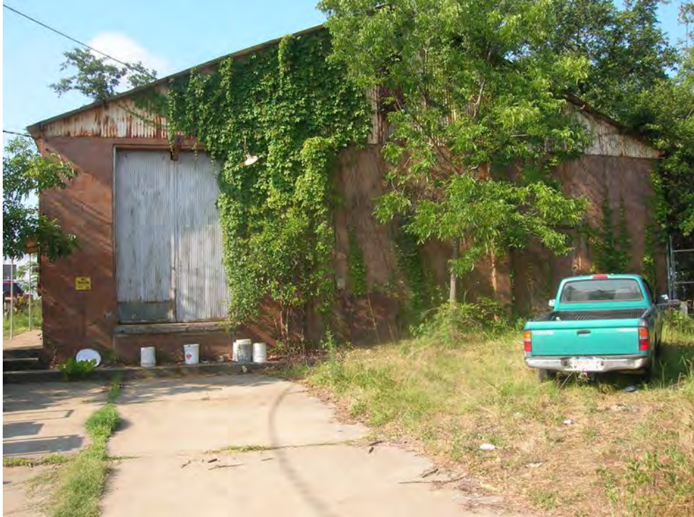
Figure 52. North side of Structure 12, originally Montgomery Elevator Company, former File Storage and Electrical Shop. View to the south.
