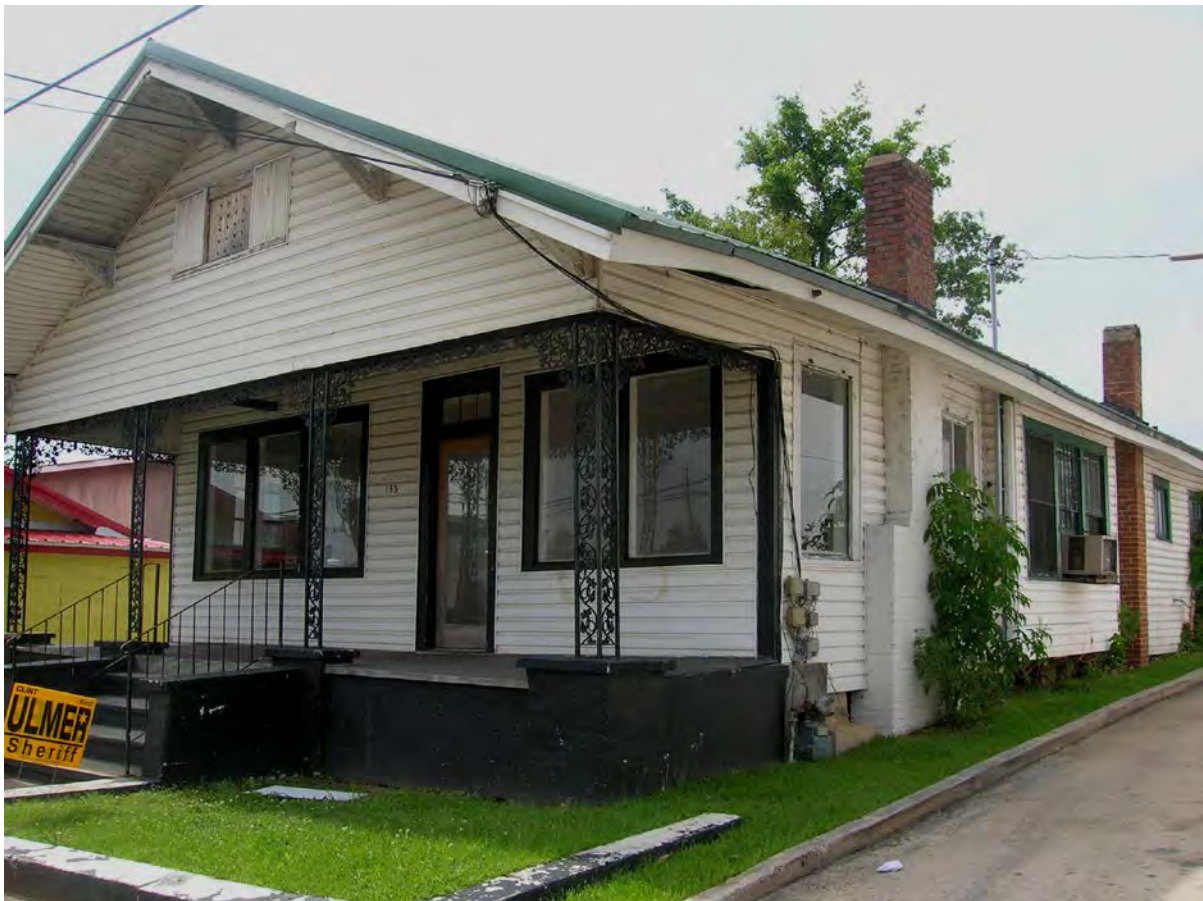
Figure 23. View to south of Structure 15, former residence, currently vacant, at 153 Canal Street on Survey Block 13.
