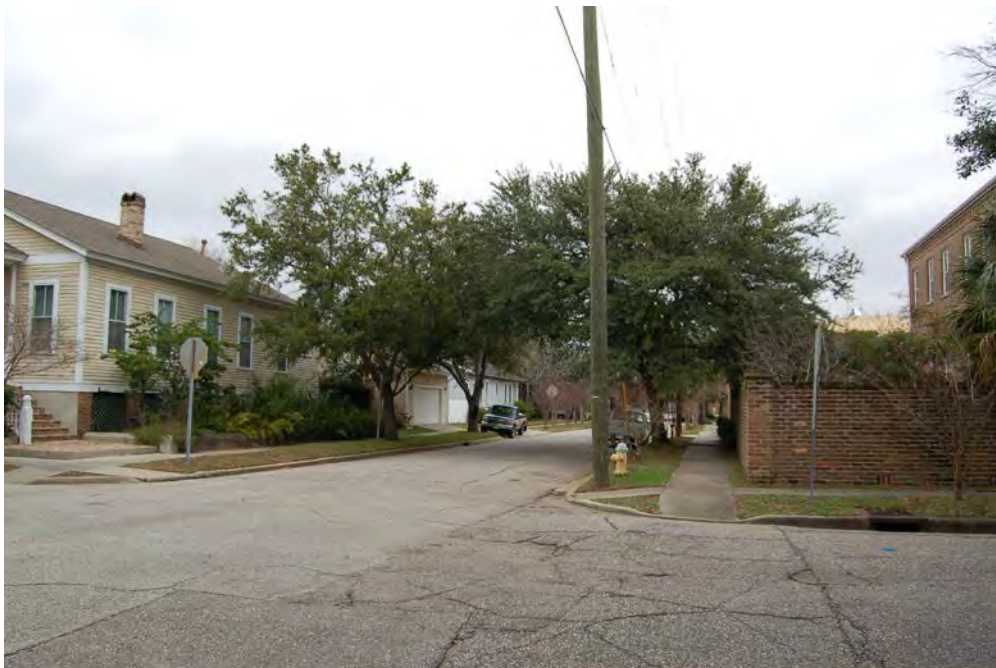
Figure 29-7. View from across S. Warren Street from Bunker-Brunson House (Resource #29) (left) down Monroe Street to the east viewshed of the proposed I-10 Mobile River Bridge showing Alternate B. Due to distance (0.4 mile) and tree canopy Alternate B would be partially visible (10%) above dome of Mobile Civic Center (right side of photograph) from the rear of the Bunker-Brunson House (Resource #29) (right side of photograph).
