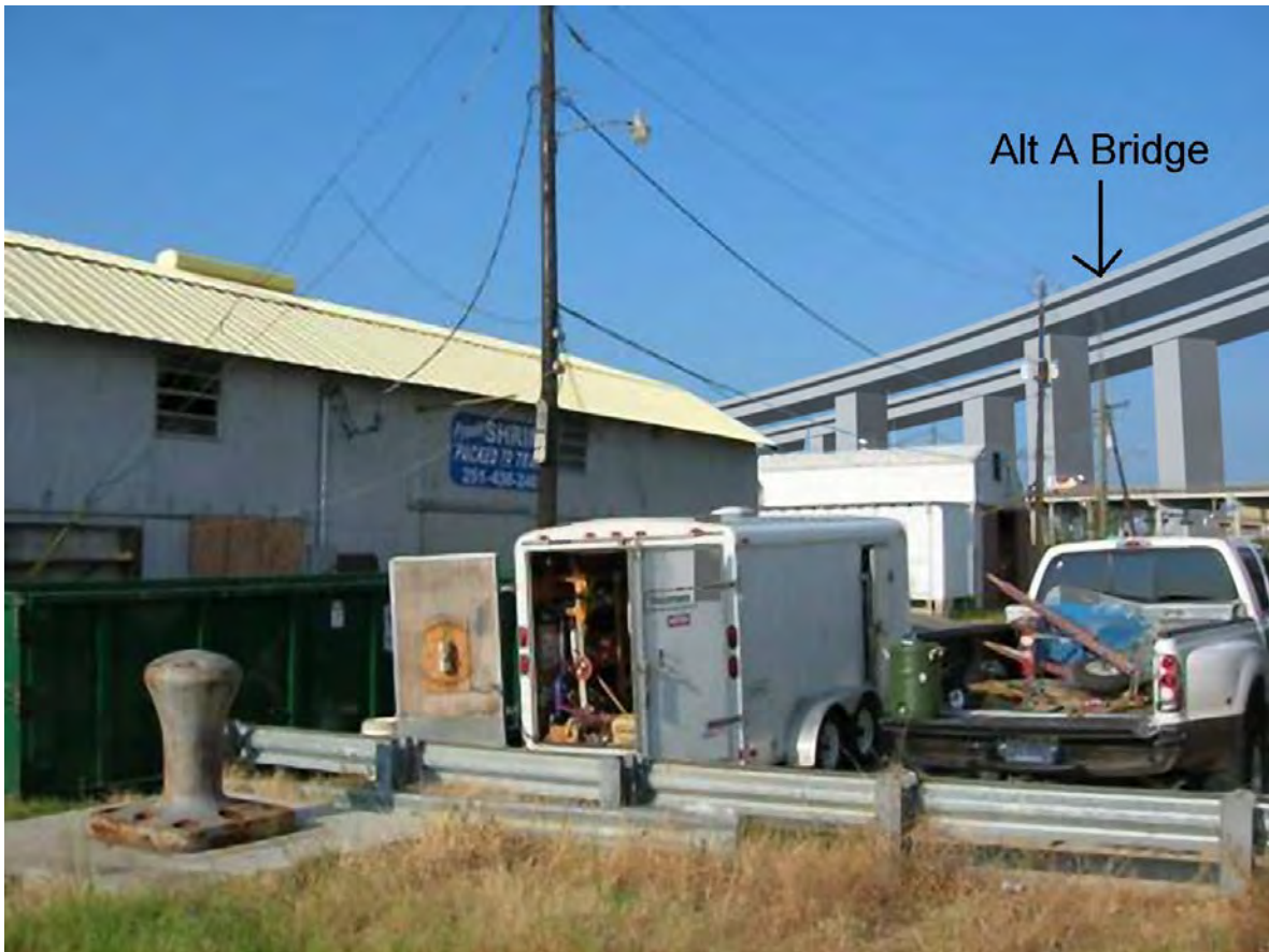
Figure 3. View to the southwest of the proposed Alternate A bridge west of Southern Fish & Oyster Company property (left) and Structure 1, Electrical Maintenance Shop (right) for the former Bender Shipbuilding & Repair Company, Inc.
