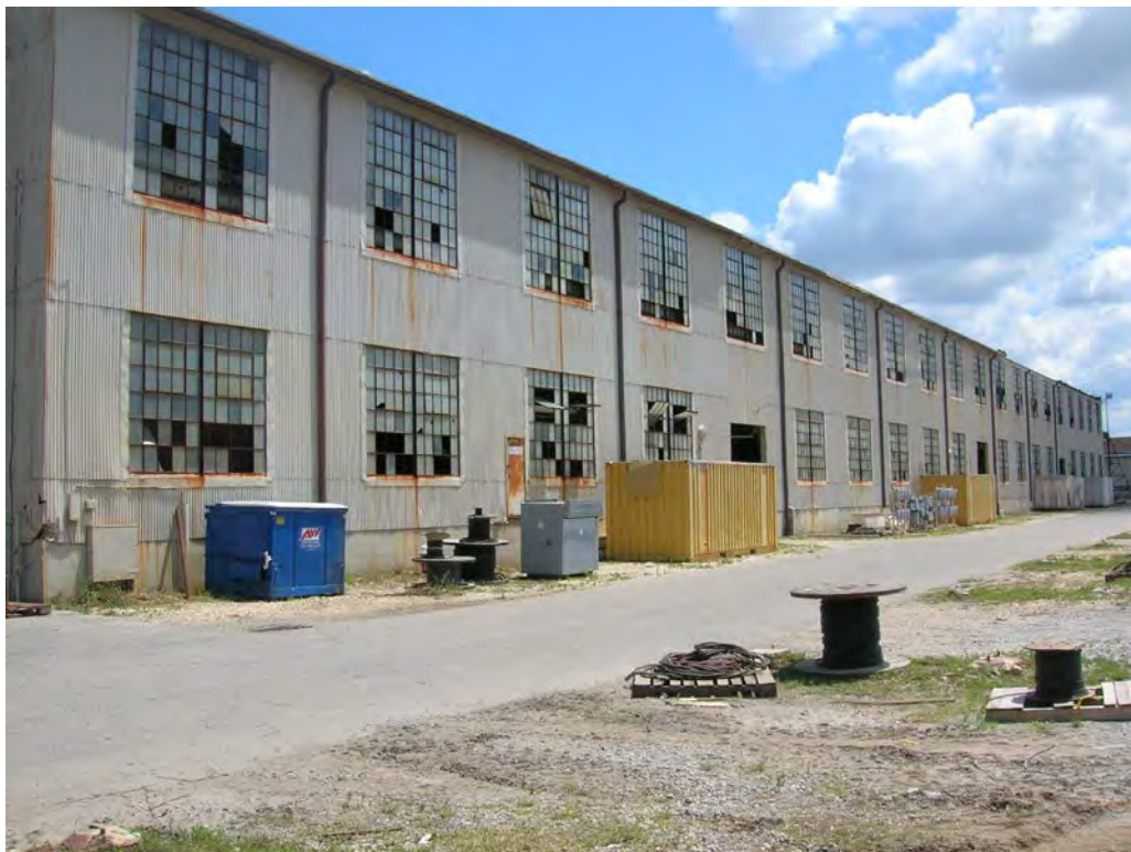
Figure 22. South side of Structure 5, Warehouse No. 2. View to the northeast.
