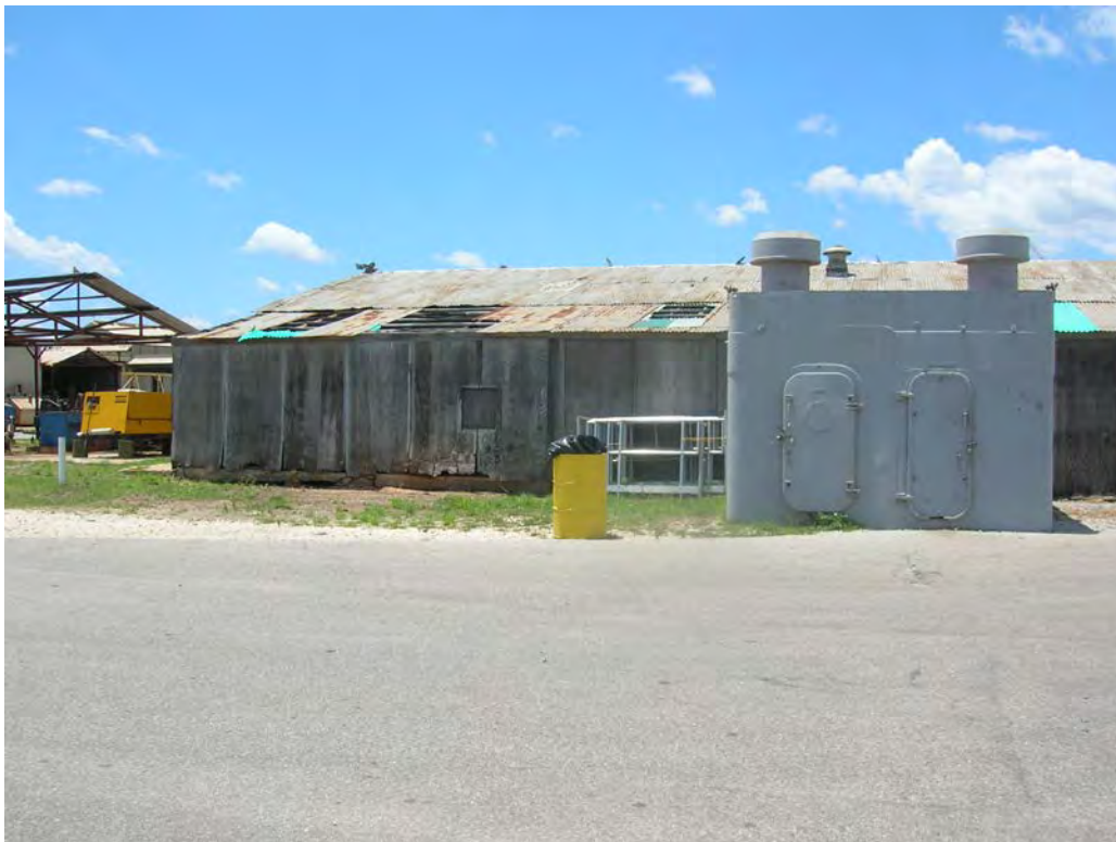
Figure 25. Front of Structure 6, originally auto repair shop, currently tool storage shed. View to the west toward Alternate C.
