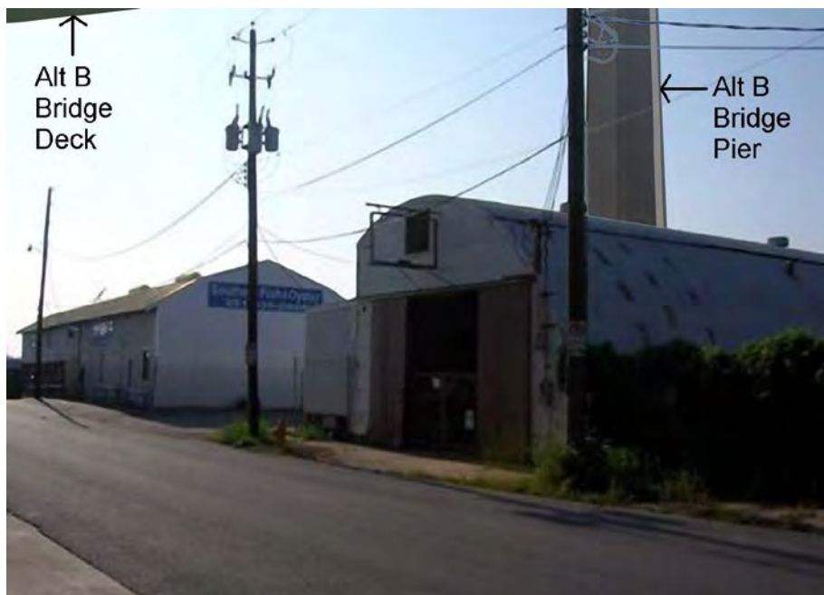
Figure 5. View to the southeast of the proposed location of Alternate B bridge deck and pier immediately south of Southern Fish & Oyster Company property (left) and Structure 1, Electrical Maintenance Shop (right) for the former Bender Shipbuilding & Repair Company, Inc., documented during this Phase I assessment.
