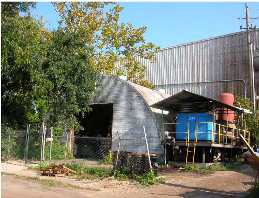
Figure 32. Structure 5, Quonset hut, with compressor on side (right), originally Radcliff Gravel Company, last used as a paint kitchen for the former Bender Shipyard. View to the northwest toward Alternates A, B, and B'.
