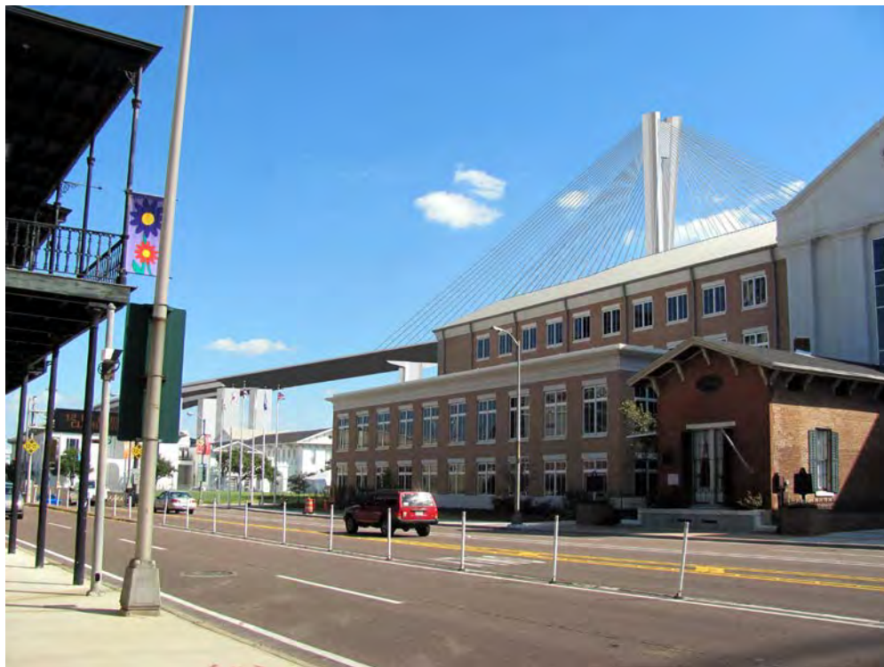
Figure 27-5. View from the intersection of Government and Conception Streets (Resource #27) to the southeast viewshed showing Alternate A bridge route and mixture of historic and nonhistoric structures, such as Dr. LeVert's Office (small brick building) in front of the multi-story Mobile County Probate Court (right), and the LaClede Hotel (left) on Government Street. Due to distance (0.3 miles) and blockage by structures, Alternate A would be visible (80-90%) above buildings from Resource #27.
