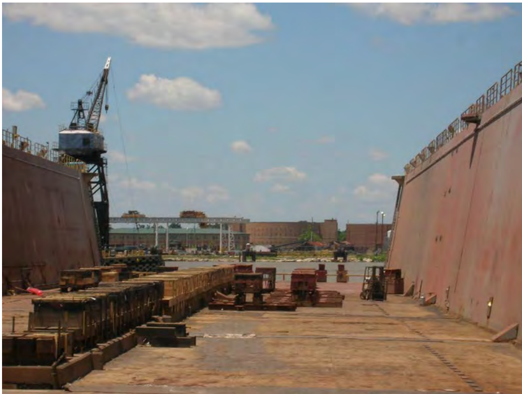
Figure 41. Structure 13, Dry Dock No. 17. View to the west toward Alternate C.
