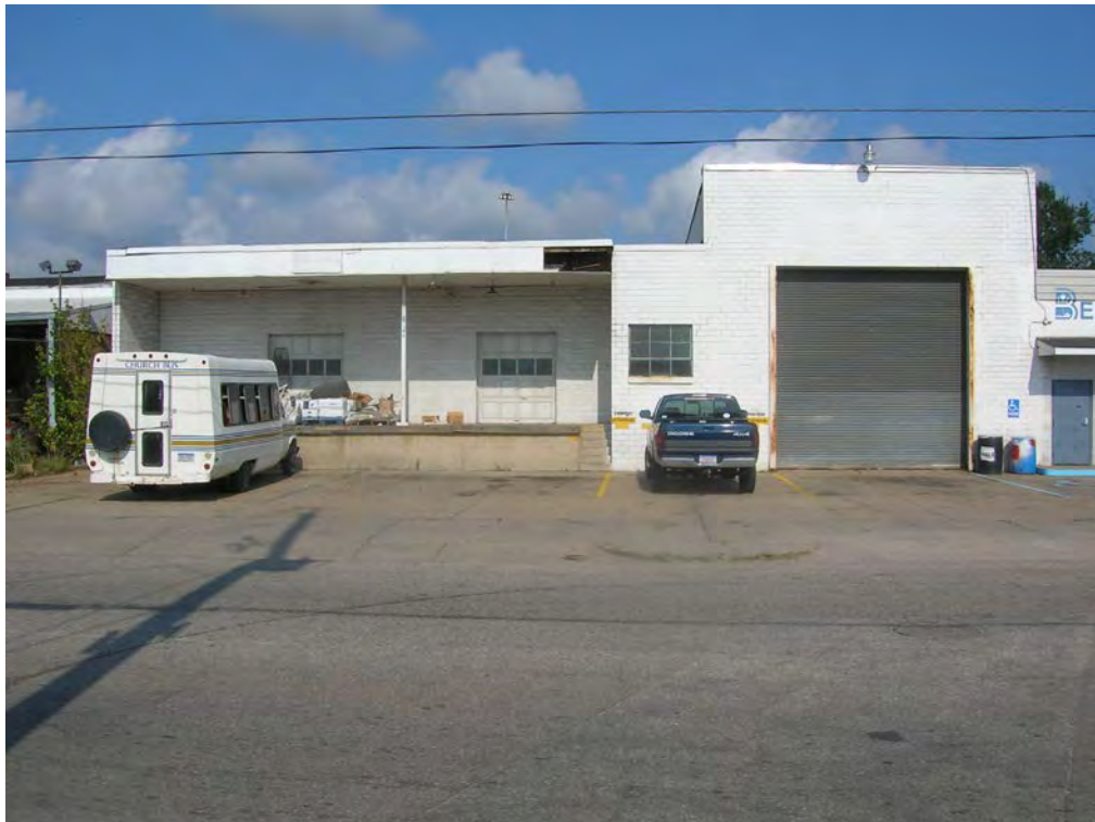
Figure 56. Structure 13, former Bender Shipyard warehouse. View to the west.
