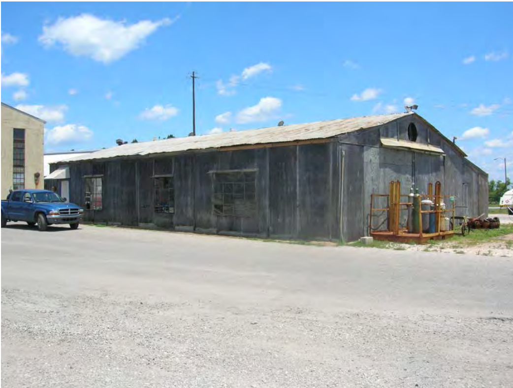
Figure 23. Structure 6, originally auto repair shop, currently tool storage shed, at BAE Systems Southeast Shipyards. View to the northeast.
