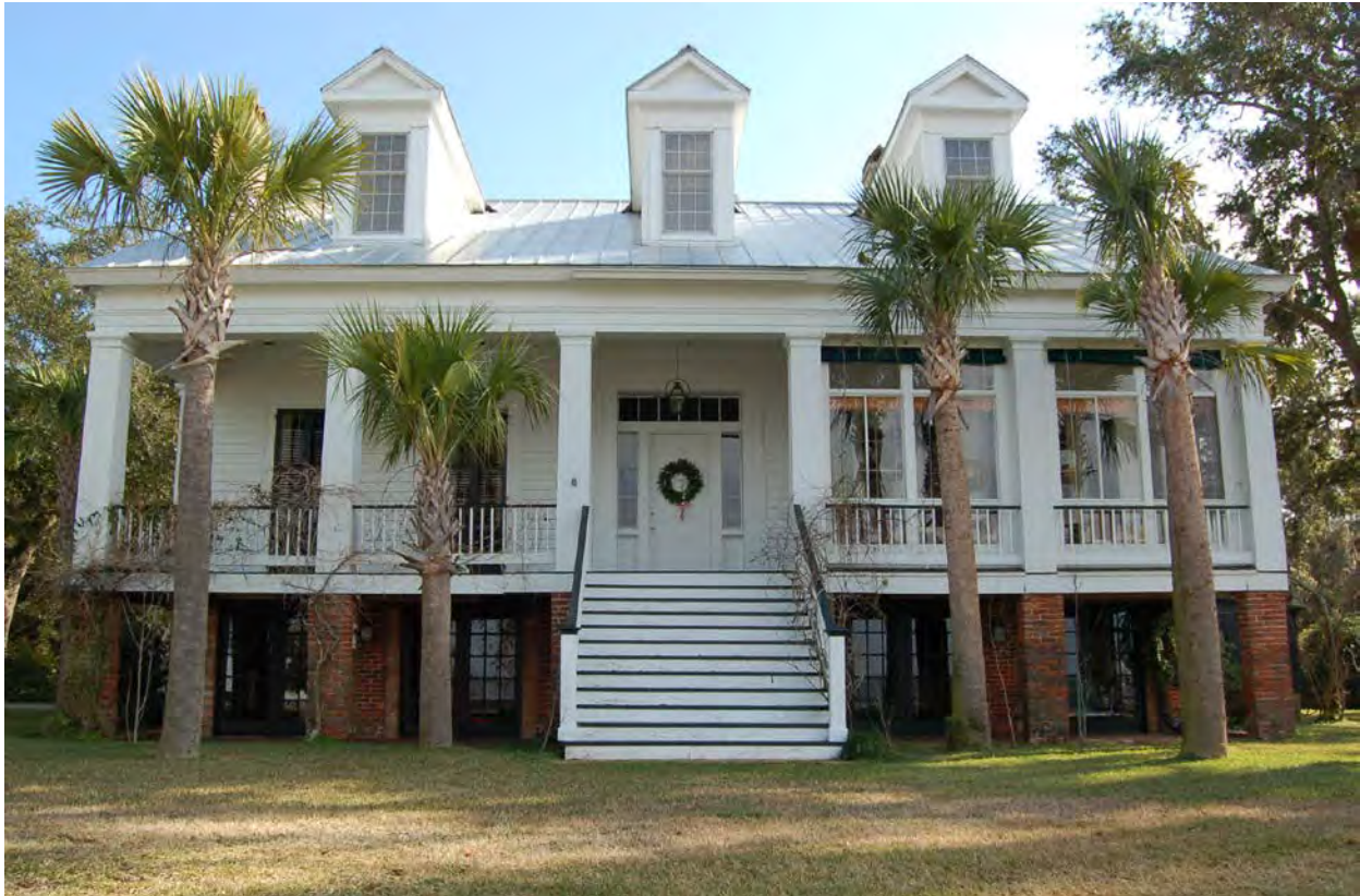
Figure 38-1. View of the west of the front of the ca. mid-1800s Captain Adams-Stone House (Resource #38) that overlooks Mobile Bay at 907 Captain O’Neal Drive in Daphne on the Eastern Shore.
