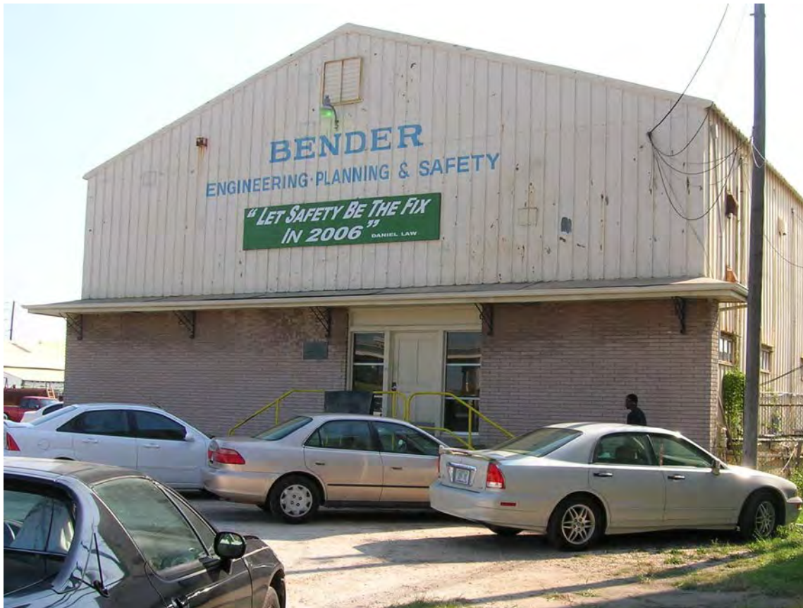
Figure 17. Front of Structure 2, Engineering, Planning & Safety Shop for the former Bender Shipyard. View to the east.
