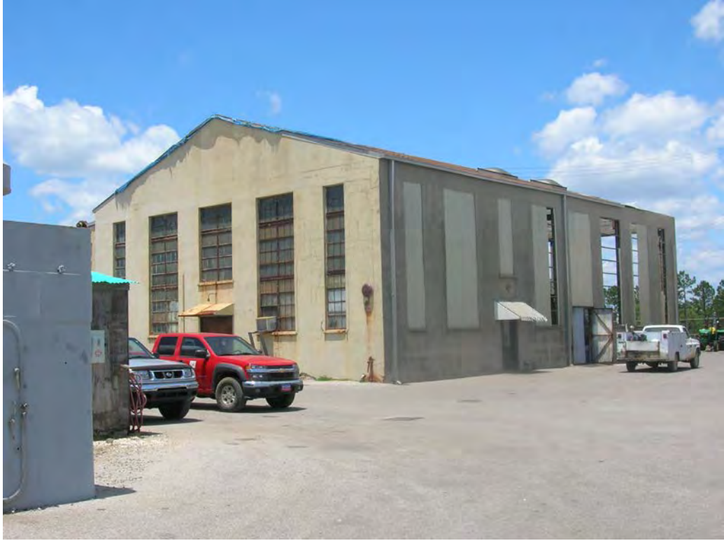
Figure 28. Structure 8, maintenance building. View to the northwest.
