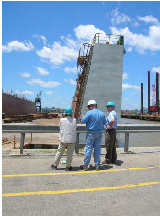
Figure 39. Structure 13, Dry Dock No. 17 at BAE Systems Southeast Shipyards. View to the west toward Alternate C.
