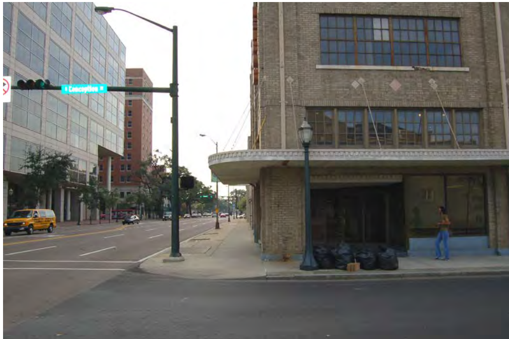
Figure 27-4. View to the south from the intersection of Government and Conception Streets (Resource #27) showing Government Plaza and historic Admiral Semmes Hotel (left) with sparse tree canopy, and historic commercial structure (right), all along Government Street.
