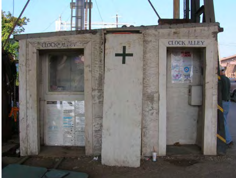
Figure 27. Two clock alleys and first aid cabinet at entrance to Structure 3, Hull Fabrication Shop. View to the west toward S. Water Street.
