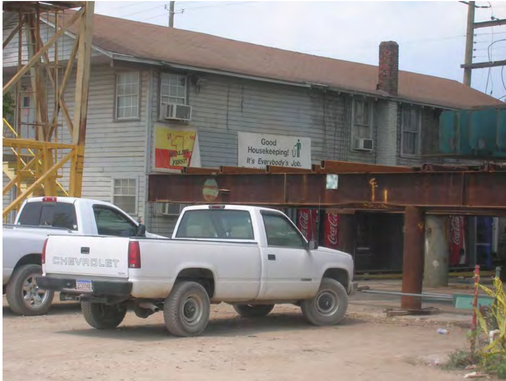
Figure 43. North side of Structure 9, originally Jackson Hope Towing Company office, former Production Office. View to the southwest.
