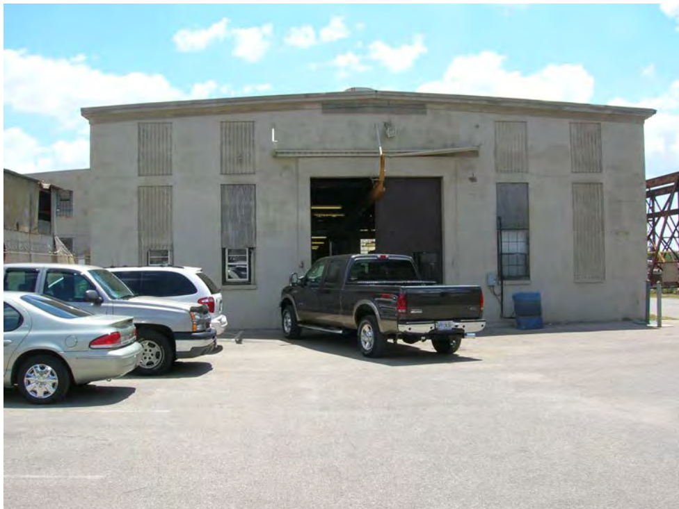
Figure 17. Front of Structure 4, electrical shop at BAE Systems Southeast Shipyards. View to the east.
