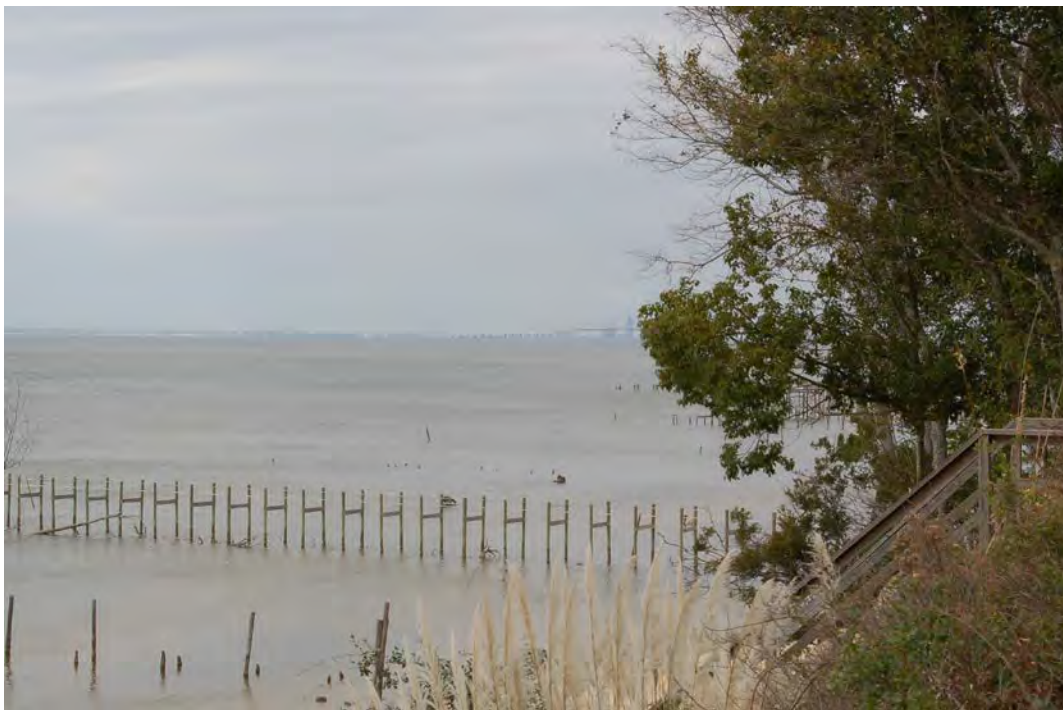
Figure 39-5. View to the northwest toward the proposed I-10 Mobile River Bridge showing Alternate A from halfway down the bluff at Seven Gables (Resource #39). The RSA Tower, RSA-Bank Trust Building, and downtown Mobile are barely visible on the horizon through the trees near the center of the photograph. At this distance (10.8 miles), Alternates A, B, B', and C would barely be visible and would not result in viewshed impacts on this resource.
