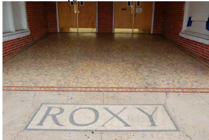
Figure 17-2. Tile floor at theater entrance.
