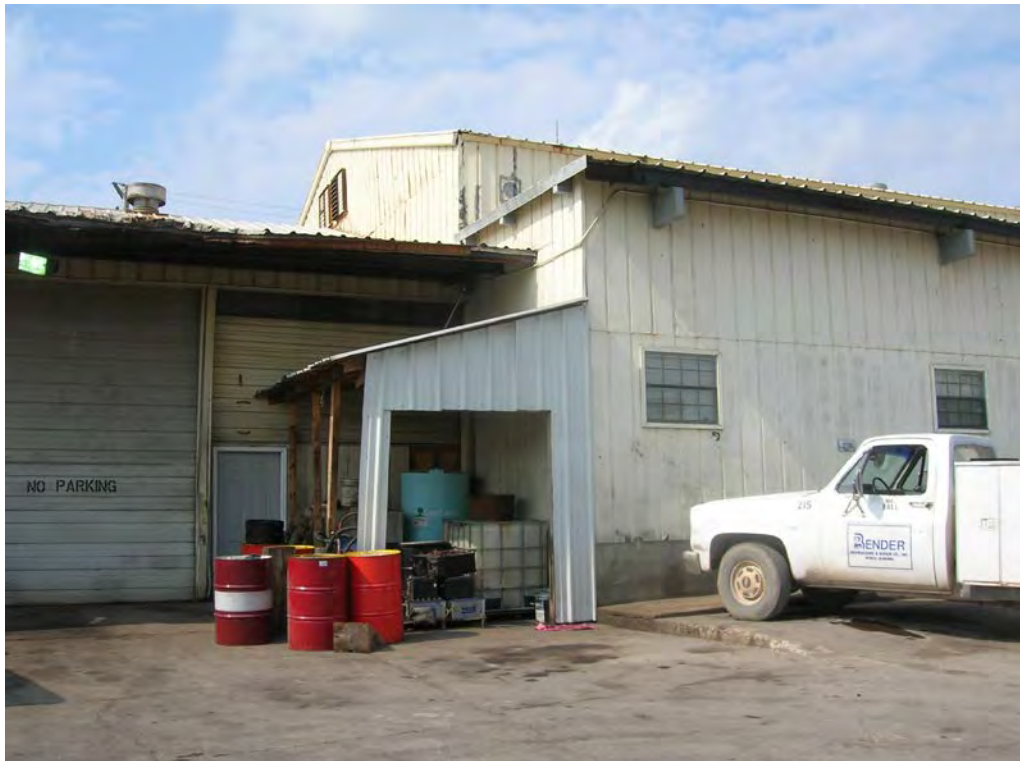
Figure 19. Rear of Structure 2, Engineering, Planning & Safety Shop. View to the south/southwest.
