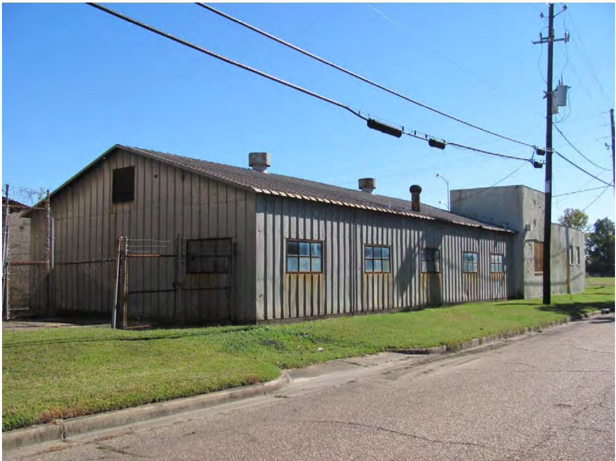
Figure 32. View to the southeast of Structure 19b, metal warehouse for A.W. Williams Inspection Co., Inc. along S. Franklin Street on Survey Block 32.
