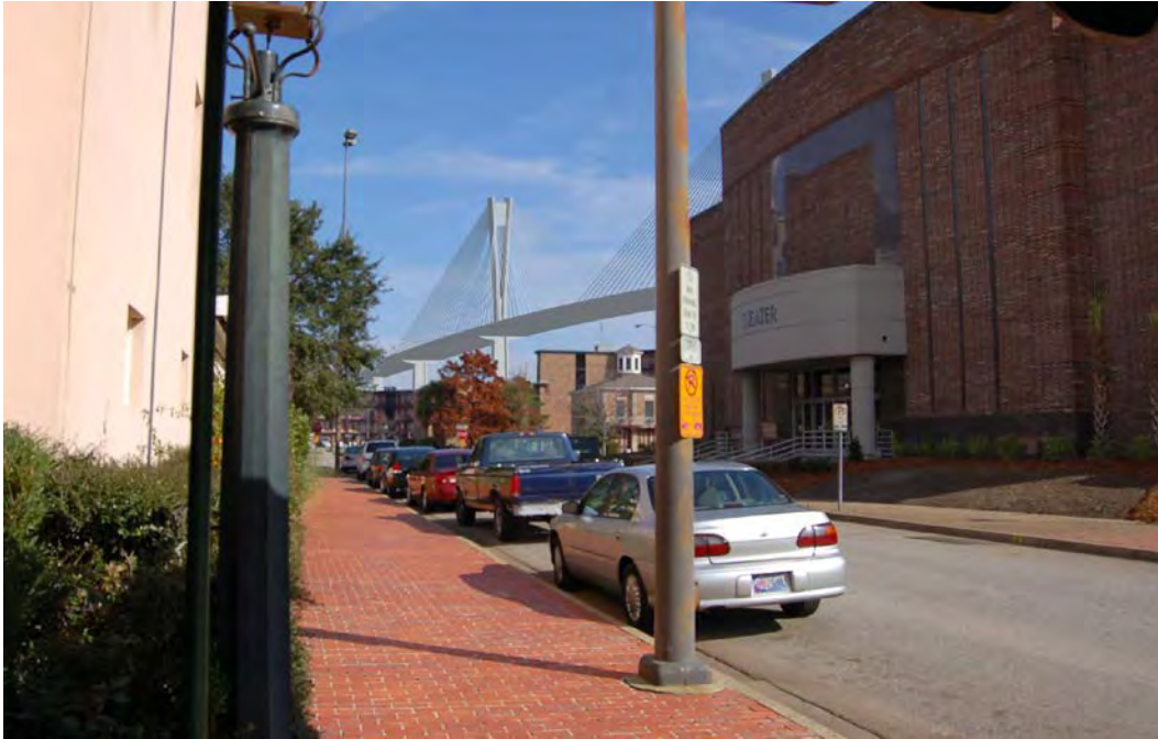
Figure 31-6. View from rear entrance of Malaga Inn (Resource #31) to the east-southeast of the proposed I-10 Mobile River Bridge showing Alternate A (0.3 miles) which would be partially visible (50-60%) above structures in the distance down Civic Center Drive.
