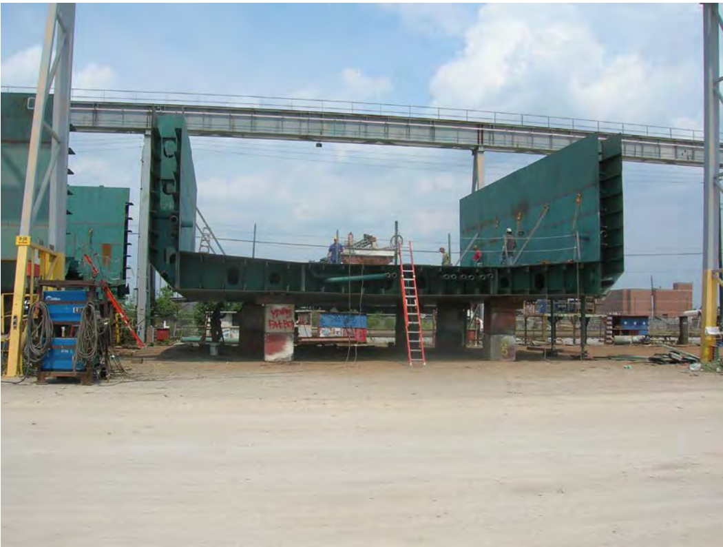
Figure 41. Ship hull in bay of Structure 8, Hull Fabrication and Assembly Shop. View to the west.
