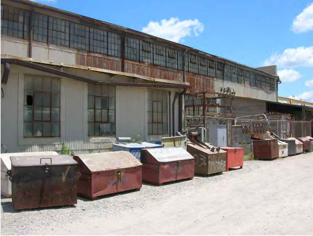
Figure 34. South side of Structure 11, Machine Shop. View to the northeast.
