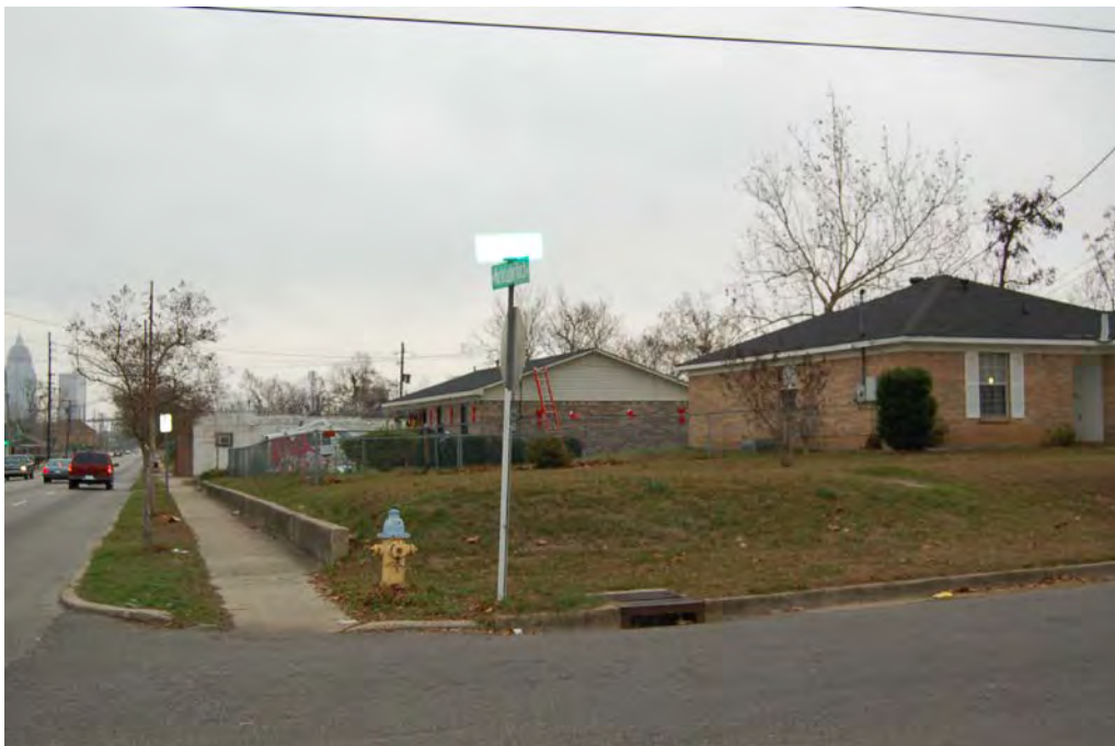
Figure 19-5. View to the east-southeast viewed of the proposed I-10 Mobile River Bridge from the intersection of MLK Avenue and Hickory Street (Resource #19) showing Alternate A (above trees on left side of photograph), a sparse tree canopy, new homes, and the RSA Tower and RSA-Bank Trust Building (left). Due to distance (1.6-1.7 miles) and blockage by structures, Alternate A would be partially visible (10-15%) from this intersection.
