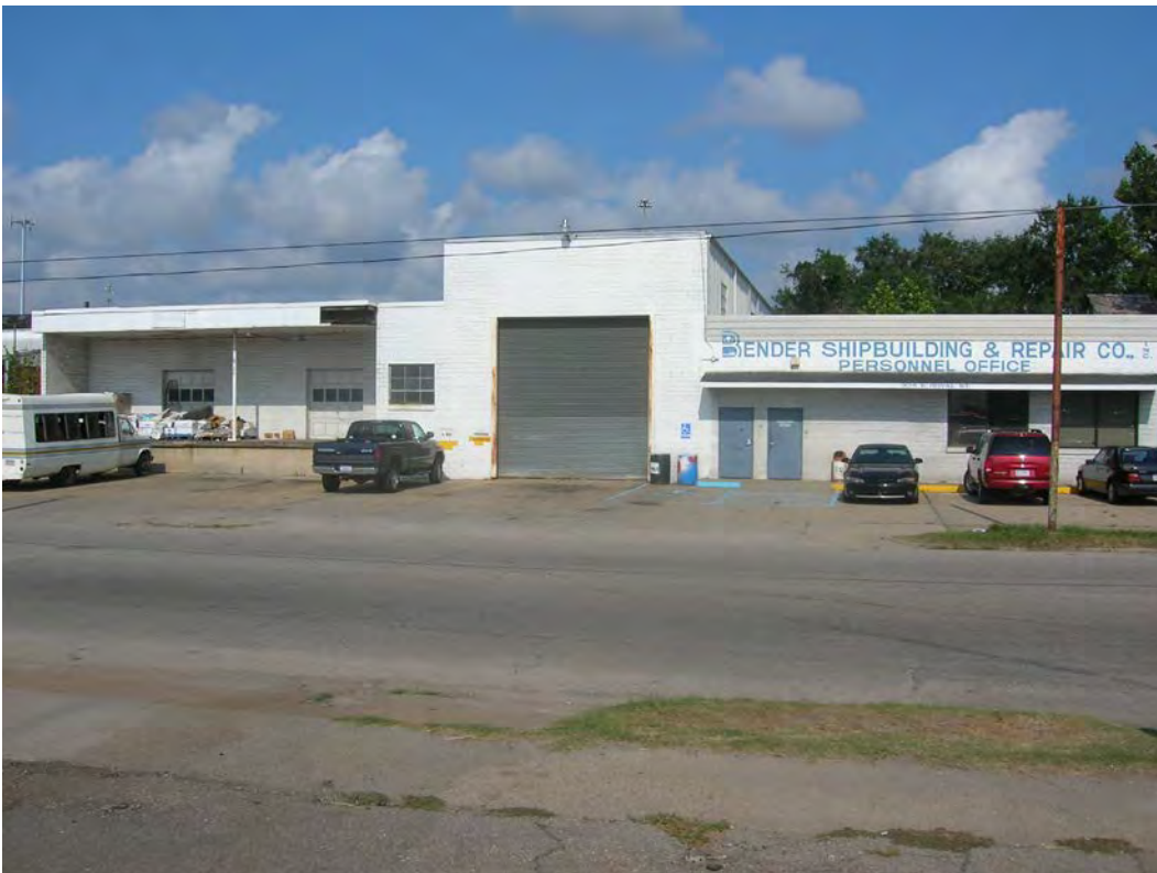
Figure 54. Structure 13, originally Pittsburgh Plate Glass Company, former Personnel Office and Warehouse at the former Bender Shipyard. View to the west toward Alternates A, B, and B’.
