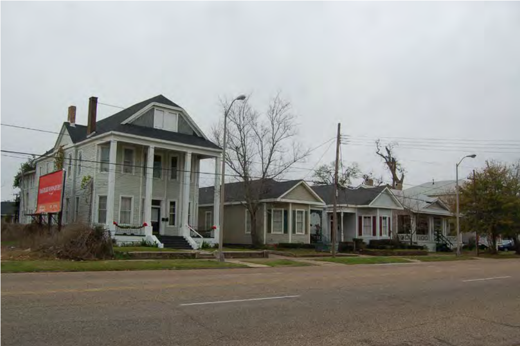
Figure 11-3. View to the southwest showing the structure at 809 Springhill Avenue (Resource #11) (left) and a row of historic houses on the south side of Springhill Avenue.
