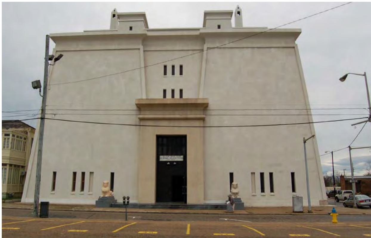
Figure 36-1. View to the west of the 1921 Scottish Rites Temple (Resource #36) at 351 St. Francis Street in Lower Dauphin Historic District.
