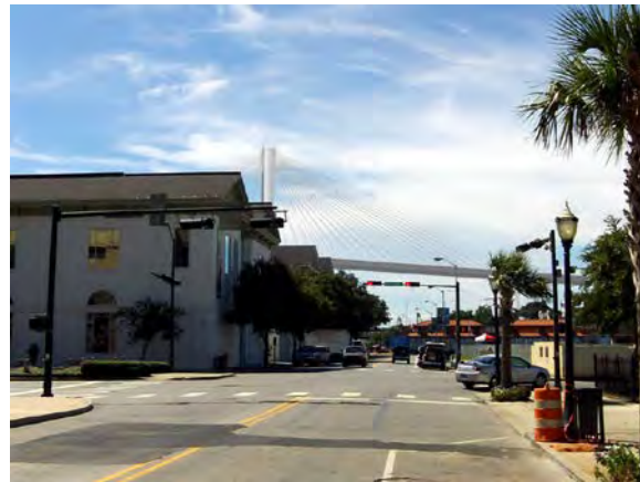
Figure 51-7. View to south from S. Royal Street showing Alternate B (0.3 miles). Alternate B' would be similarly visible.
