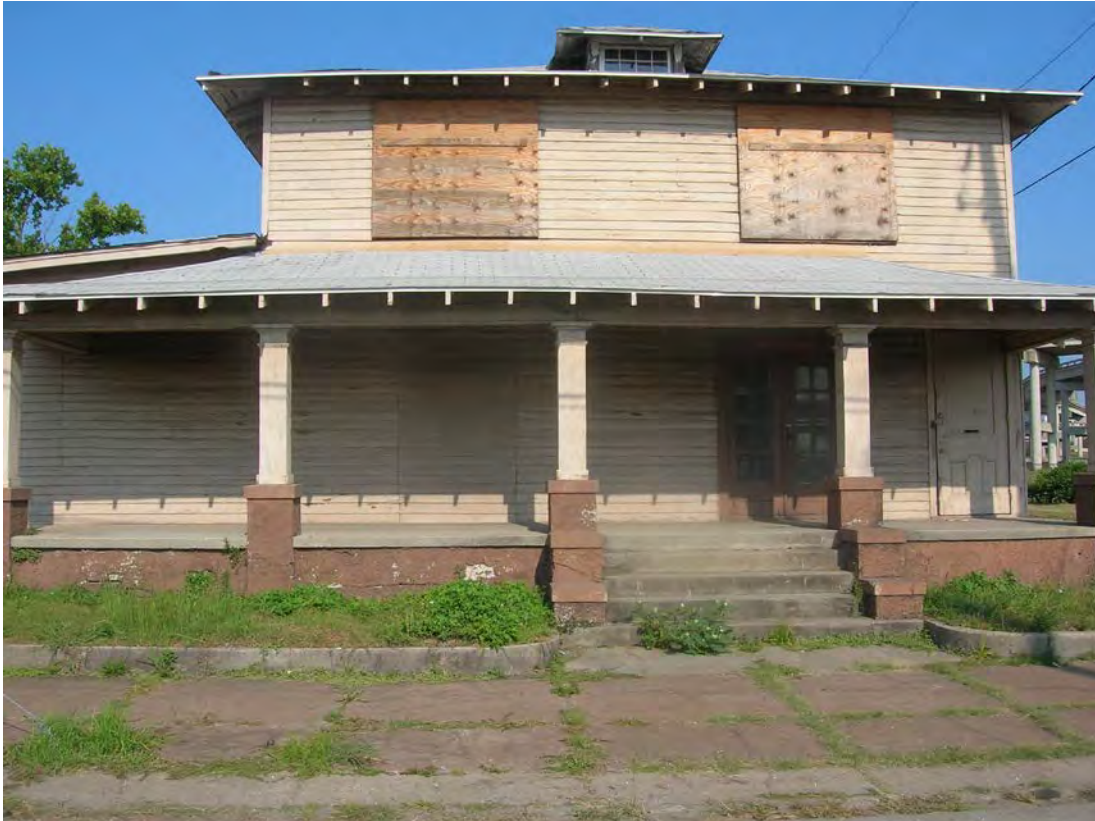
The old Union Hall, (former Bender Structure 11) on S. Royal Street
