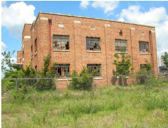
Figure 11. East side of Structure 1, main office. View to the west.
