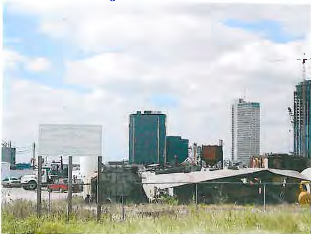
Harrison Brothers Dry Dock & Repair Yard looking west from Dunlap Drive. (Alternatives A, B and B')
