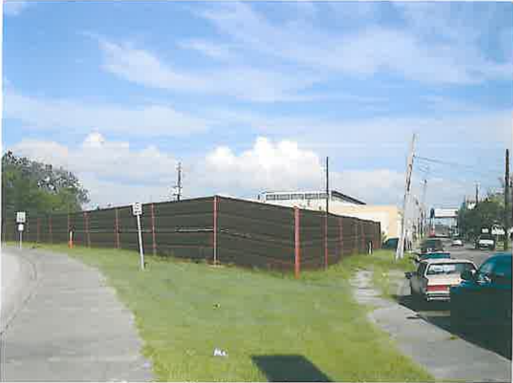
Complete Equipment North Parcel looking east along Canal Street (Alternative B and B'). Building behind fence is the former National Linen Service Site.
