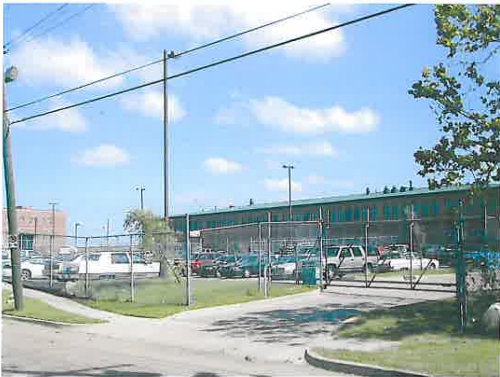
Back side of Sheriff's Office from Saint Emanuel Street (Alternate C)
