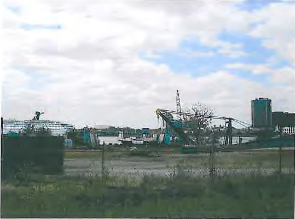
Harrison Brothers Dry Dock & Repair Yard looking west from Dunlap Drive (Alternative A).
