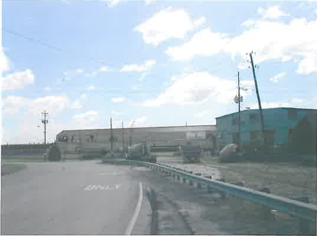
Atlantic Marine looking south along Dunlap Drive near Pinto Pass. Alternative C alignment runs between the two buildings.
