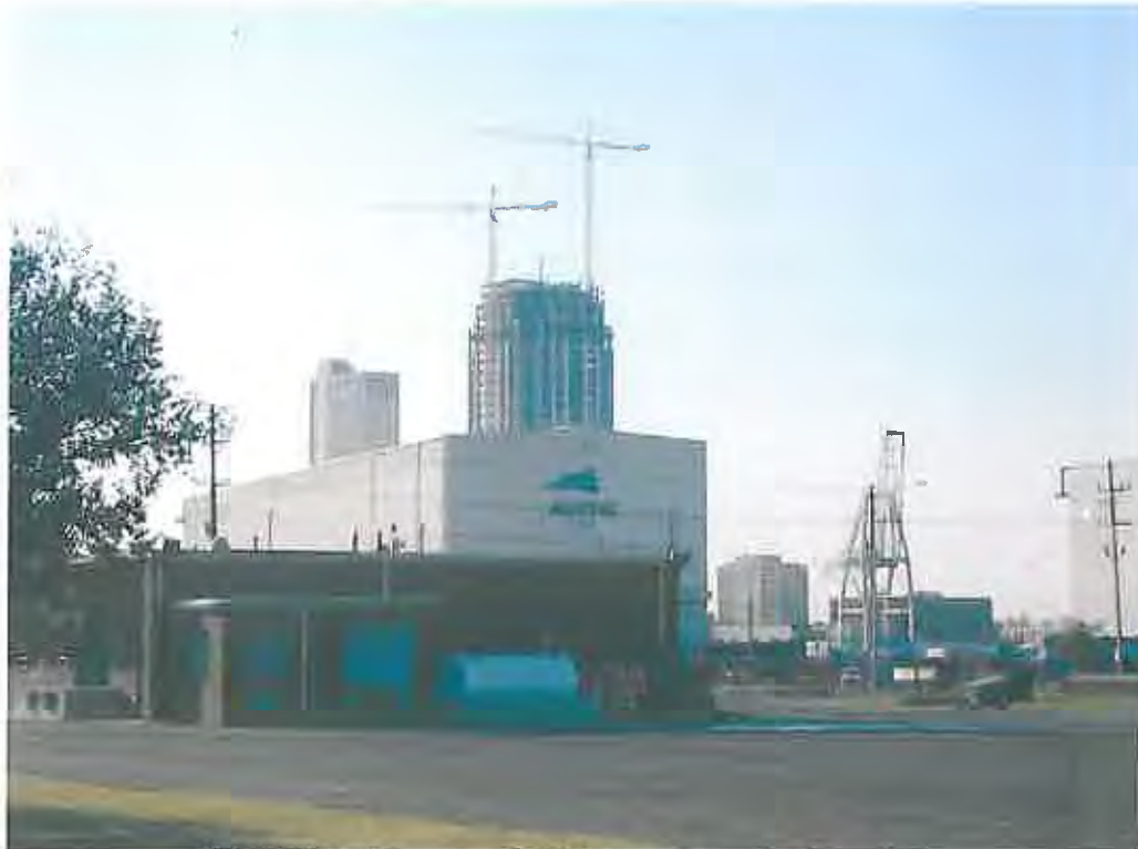
ALDOT Maintenance Building and new fueling station looking northwest from Addsko Road near Alternative A
