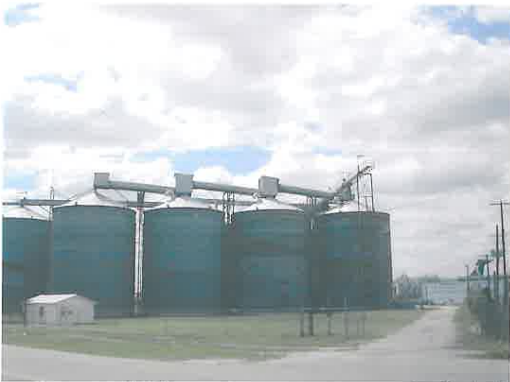
Harrison Brothers Dry Dock & Repair Yard grain silos looking west from Dunlap Drive. (Alternative B and B')
