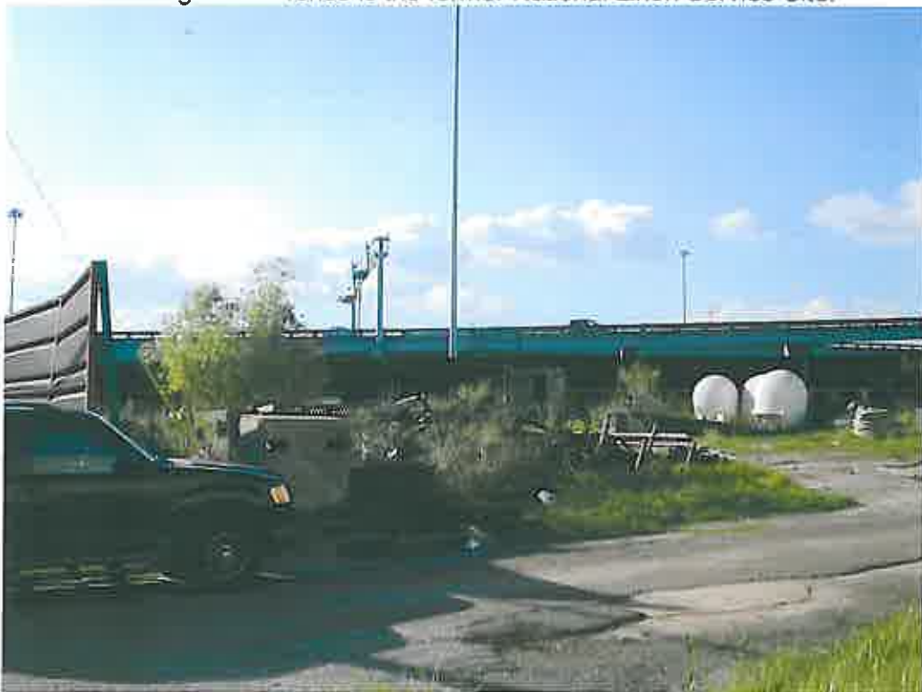
Complete Equipment North Parcel looking west from Canal Street (Alternative B and B'). This is the area behind the fence in the previous photograph.
