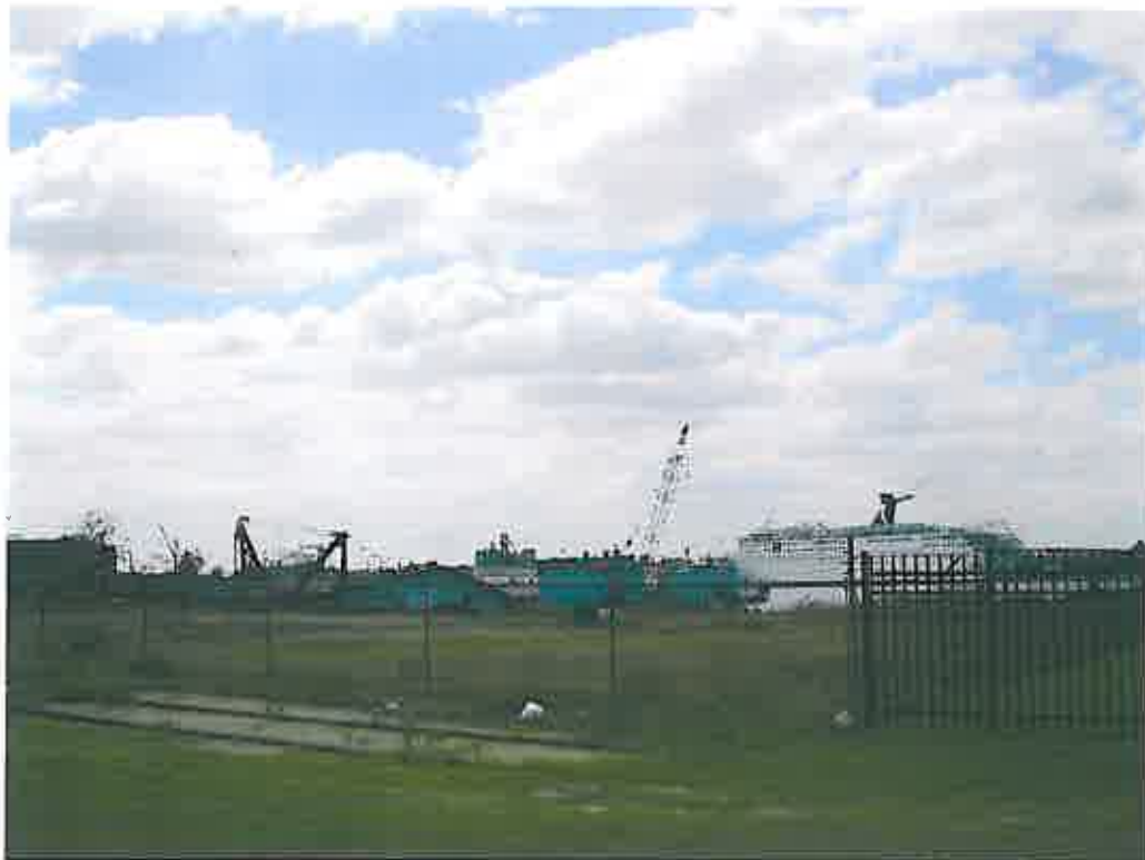
Harrison Brothers Dry Dock & Repair Yard looking west from Dunlap Drive adjacent to I-10 Wallace Tunnel Right-of-Way (Alternative A).
