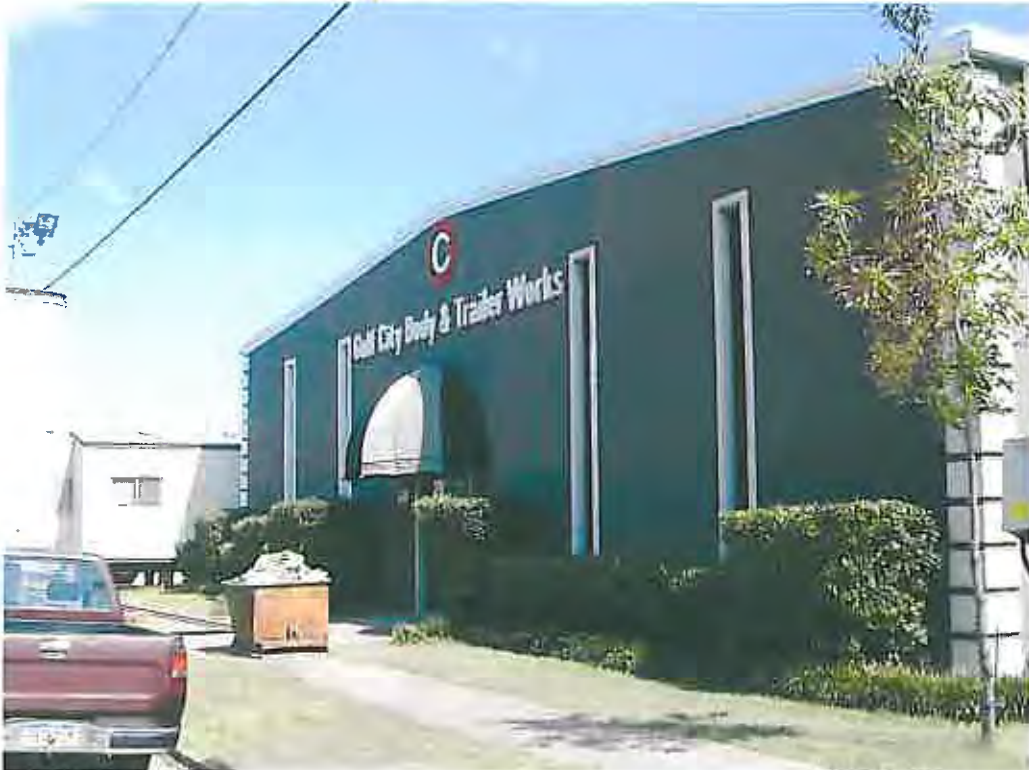
Gulf City Body & Trailer Works main office located at 601 South Conception Street. The business occupies several buildings over a large area (See Map)
