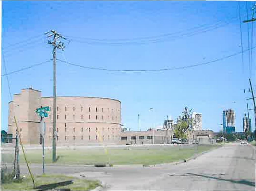
Mobile County Metro Jail from corner of Savannah and Saint Emanuel looking north (Alternative C). The former Mobile Bus Maintenance site was located between the intersection and the jail.
