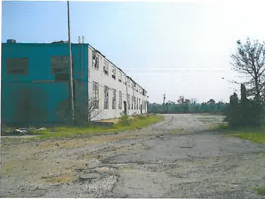
Atlantic Marine looking northeast toward Dunlap Drive along Alternative C alignment. Building on left is part of WW II Facility.
