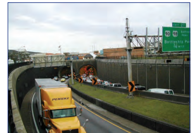
Traffic projections indicate that congestion in the Wallace Tunnel will worsen as traffic volumes through the tunnel increase.
