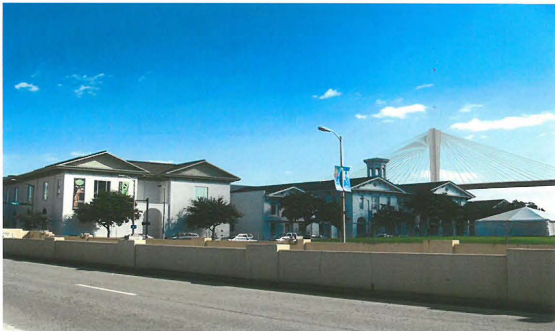
Photo Number 27 – Old Southern Market and Old City Hall (now Museum of Mobile) looking southeast toward Alternative B rendering.
