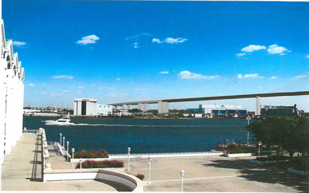
Photo Number 8 – Church Street East Historic District looking east toward Cooper Riverside Park and Alternative B' (Preferred) rendering.
