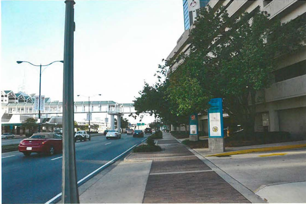
Photo Number 21 – Edge of Lower Dauphin Street Historic District looking south at Mobile Convention Center, elevated walkway, Maritime Museum, cruise terminal, and parking garage.
