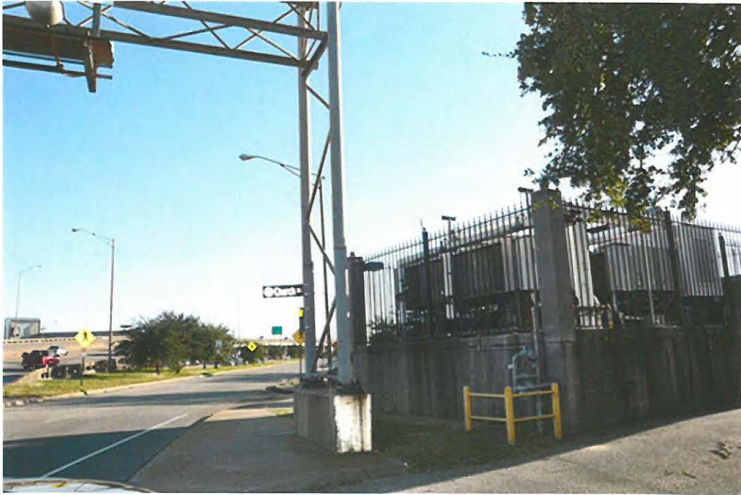
Photo Number 4 - Southeast corner of the Church Street East Historic District/Old Southern Market and Old City Hall looking south at I-10 ramp, overhead signs, and air conditioning unit.
