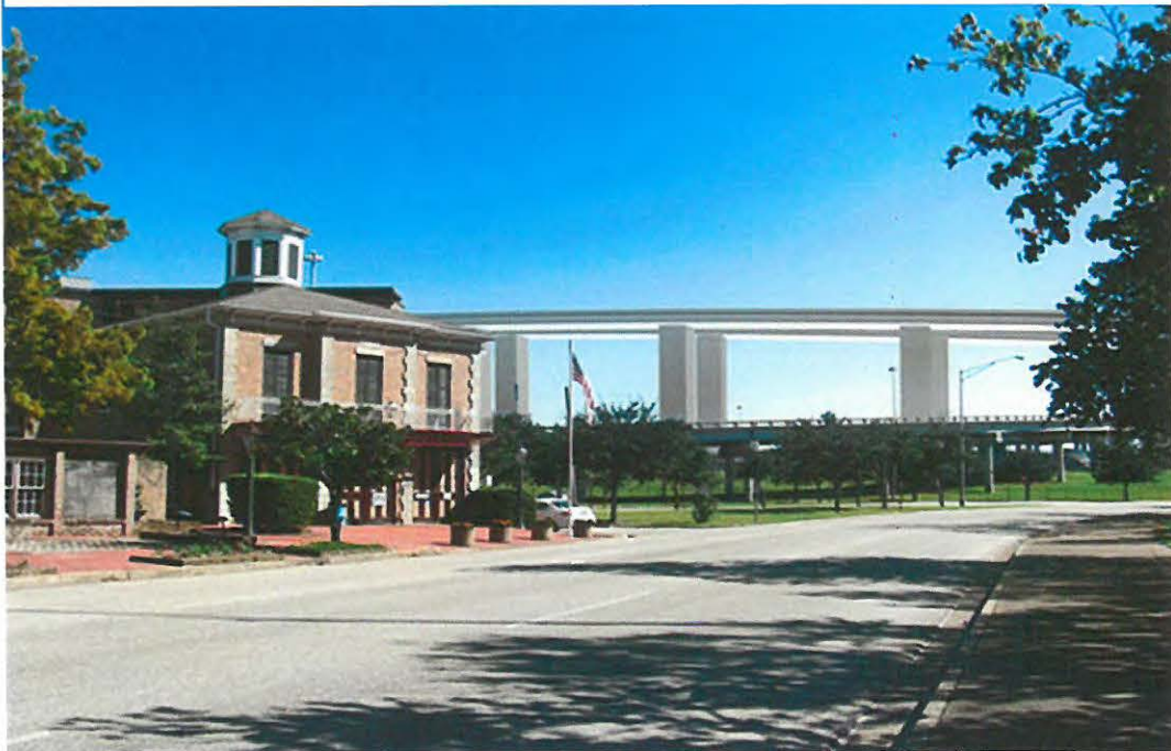
Photo Number 13 – Church Street East Historic District looking south toward the Phoenix Fire Museum and Alternative A rendering.
