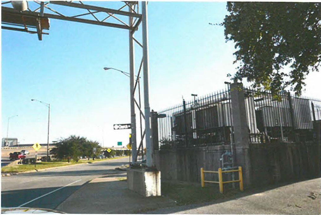
Photo Number 4 - Southeast corner of the Church Street East Historic District/Old Southern Market and Old City Hall looking south at I-10 ramp, overhead signs, and air conditioning unit.
