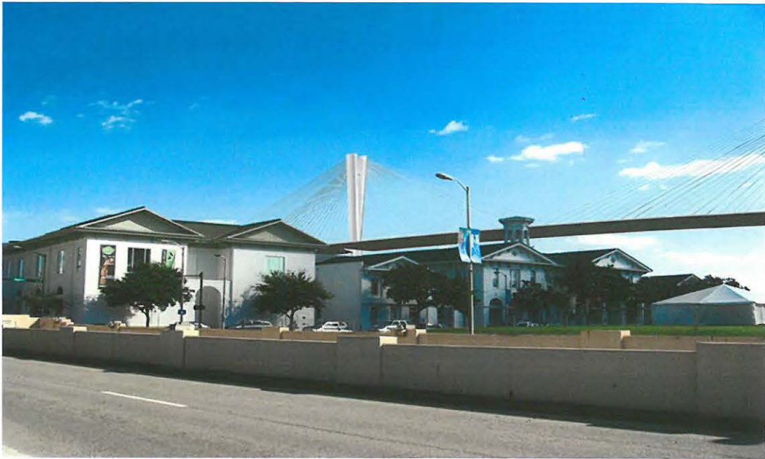
Photo Number 26 – Old Southern Market and Old City Hall (now Museum of Mobile) looking southeast toward Alternative A rendering.
