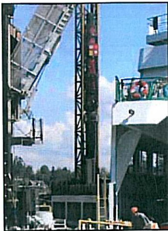
D30-42 Finishing Dolphin Piles.
